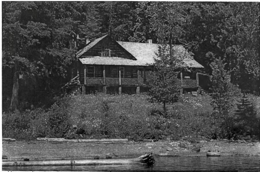
Big House, Kelly's Camp Historic District Glacier National Park, Flathead County, Montana Photograph No. 1
