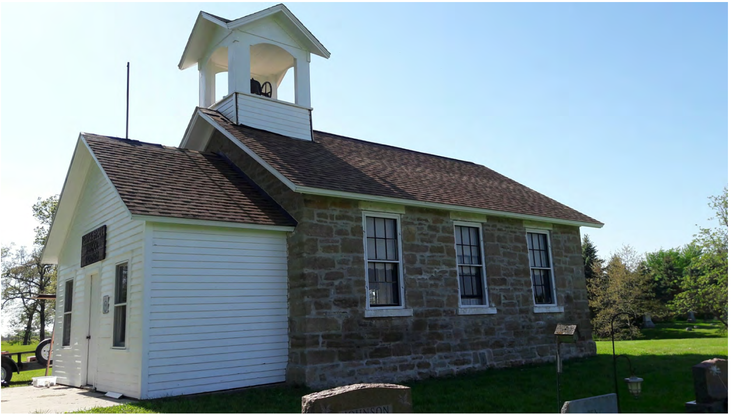
Figure 1. Prairie Grove School with new roof shingles, view northwest, May 2017 Photo by Gary Johnson, Iowa City, Iowa
