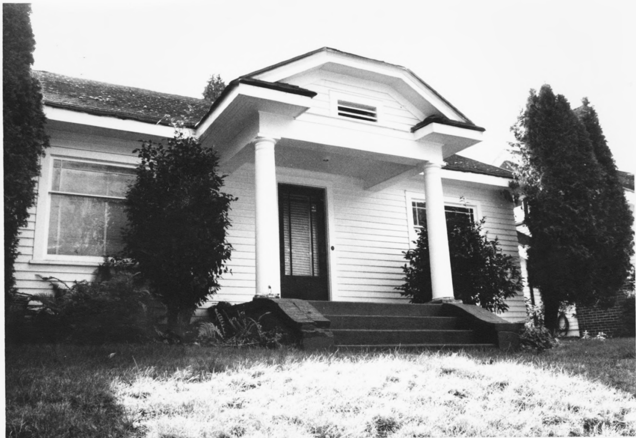
205 MAPLE PARK, NORTH FACADE, S. CAPITOL NEIGHBORHOOD H.D., # 54
