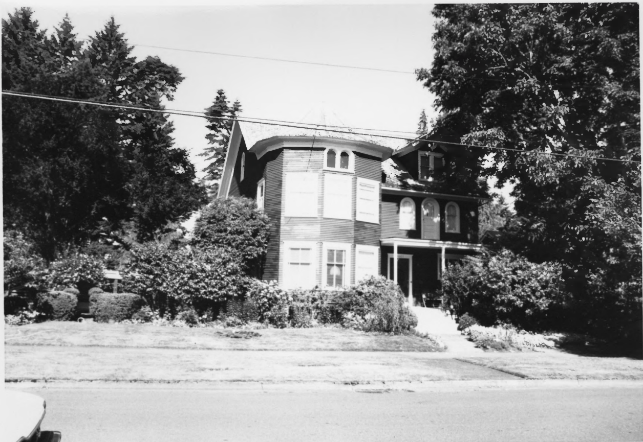
1825 S. COLUMBIA, EAST FACADE, S. CAPITOL NEIGHBORHOOD H.D., # 28
