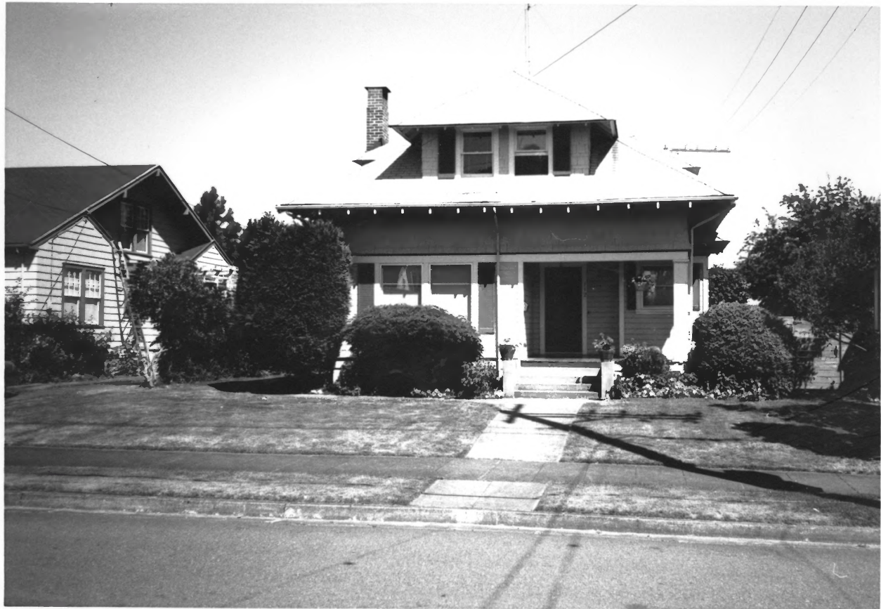
112 W. 18TH, SOUTH FACADE, S. CAPITOL NEIGHBORHOOD H.D. # 35
