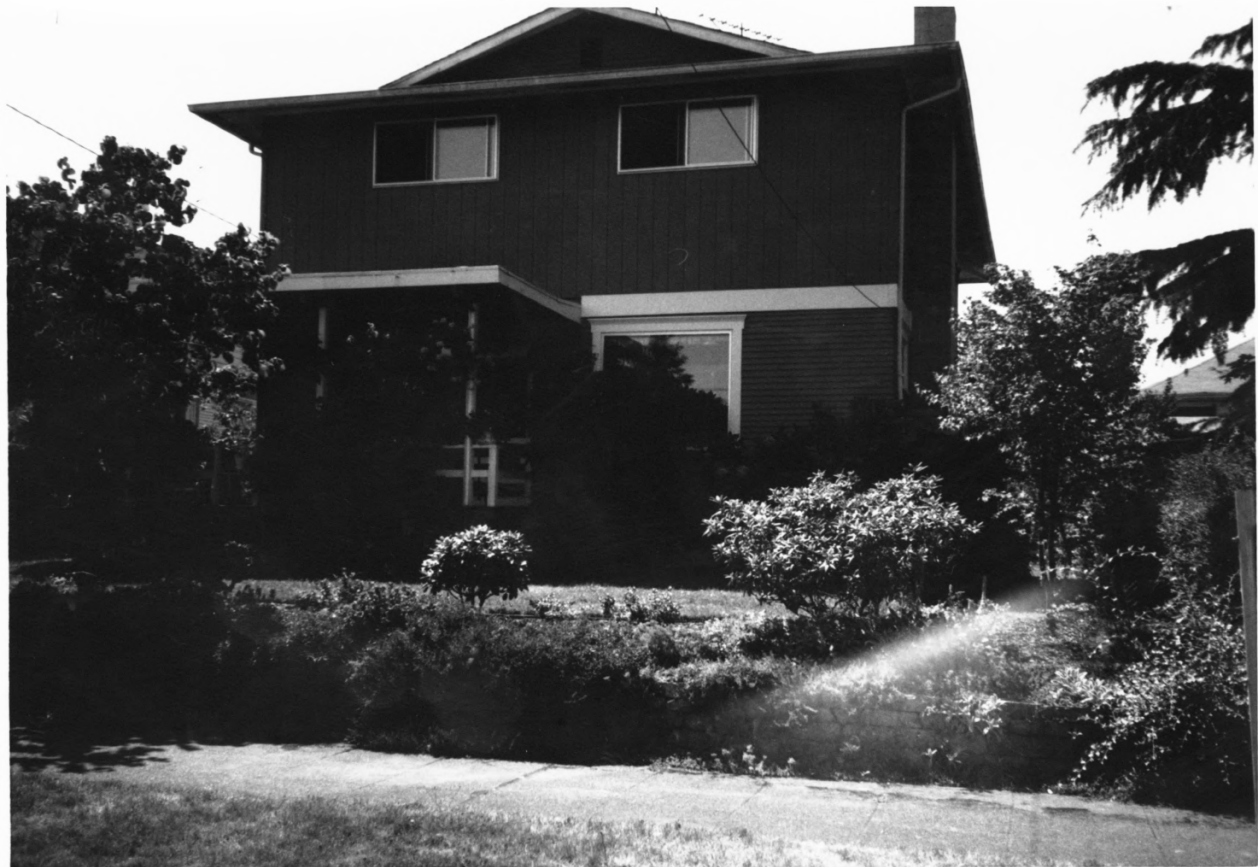
214 W. 18TH SOUTH FACADE, S. CAPITOL NEIGHBORHOOD H.D., # 37
