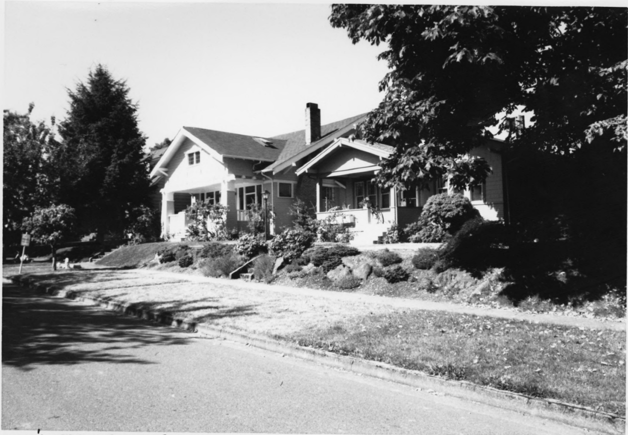
1513 & 1509 S. COLUMBIA, EAST FACADE, S. CAPITOL NEIGHBORHOOD H. D., # 58
