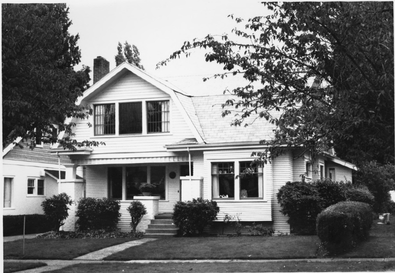
1532 S. COLUMBIA, WEST FACADE, S. CAPITOL NEIGHBORHOOD H.D., # 56
