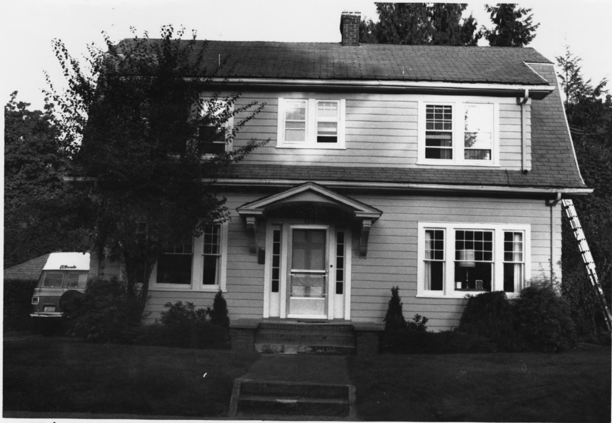
2518 S. WASHINGTON, WEST FACADE, S. CAPITOL NEIGHBORHOOD H.D. #1
