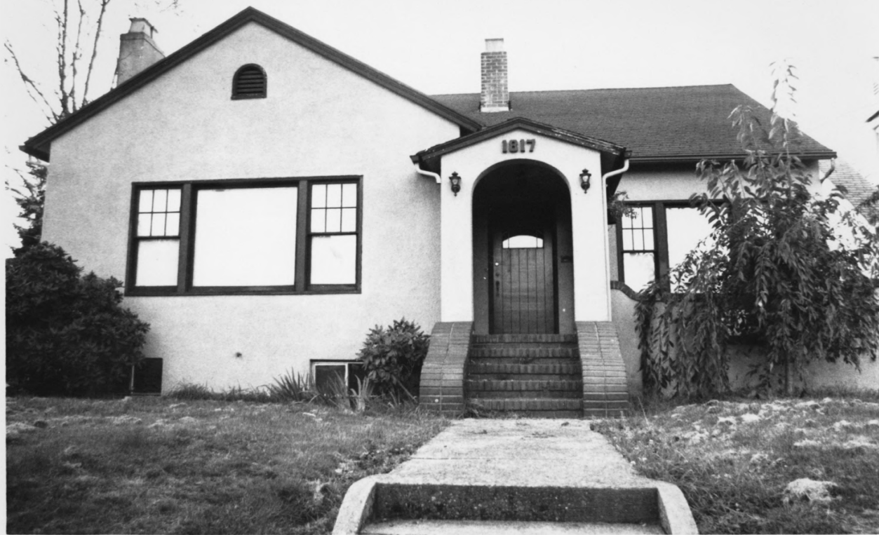
1817 S. FRANKLIN, EAST FACADE, S. CAPITOL NEIGHBORHOOD H. D., #31
