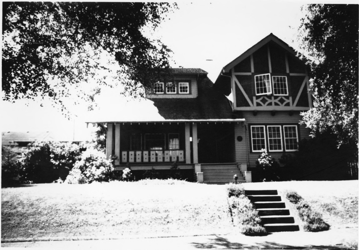
127 W. 17TH, NORTH FAÇADE, S. CAPITOL NEIGHBORHOOD H.D., #46
