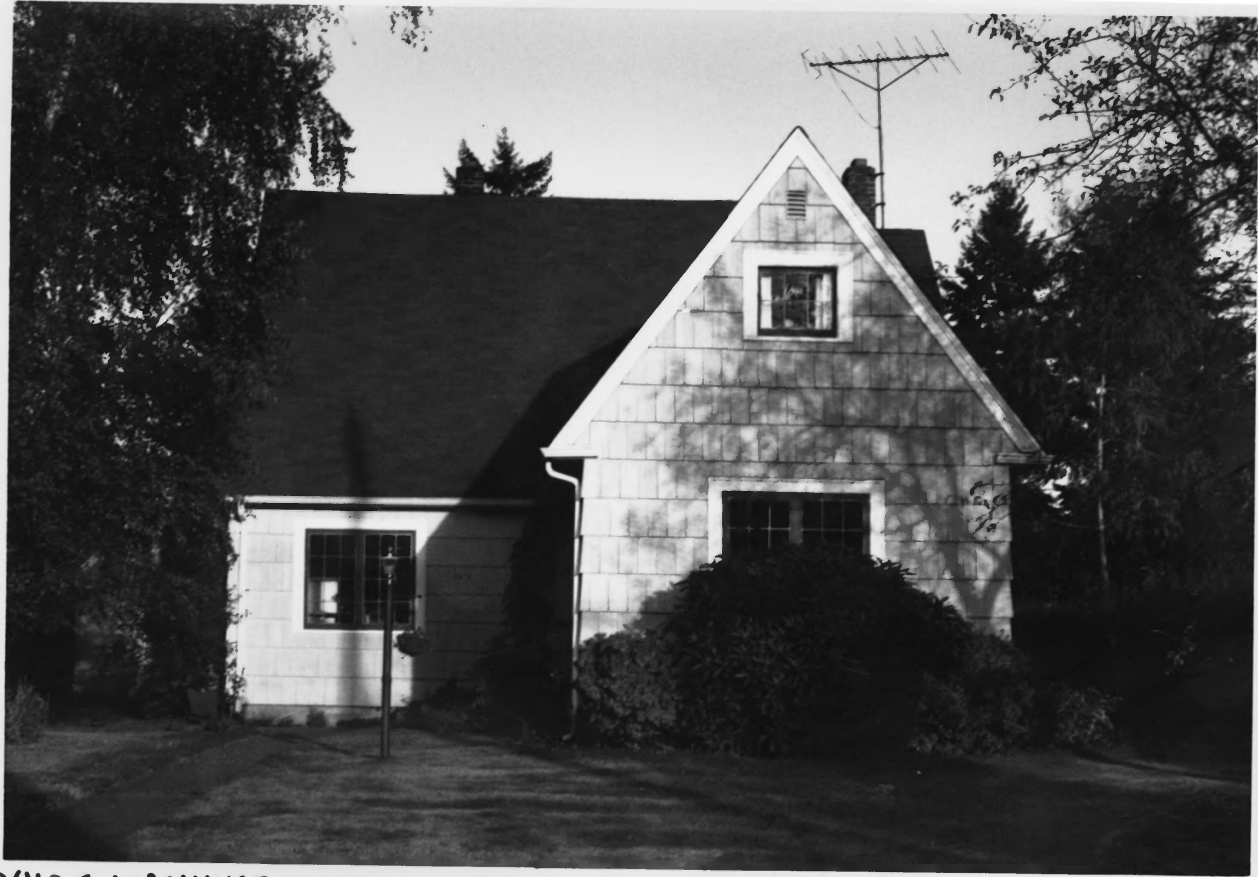
2412 S. WASHINGTON, WEST FACADE, S CAPITOL NEIGHBORHOOD H.D., #5
