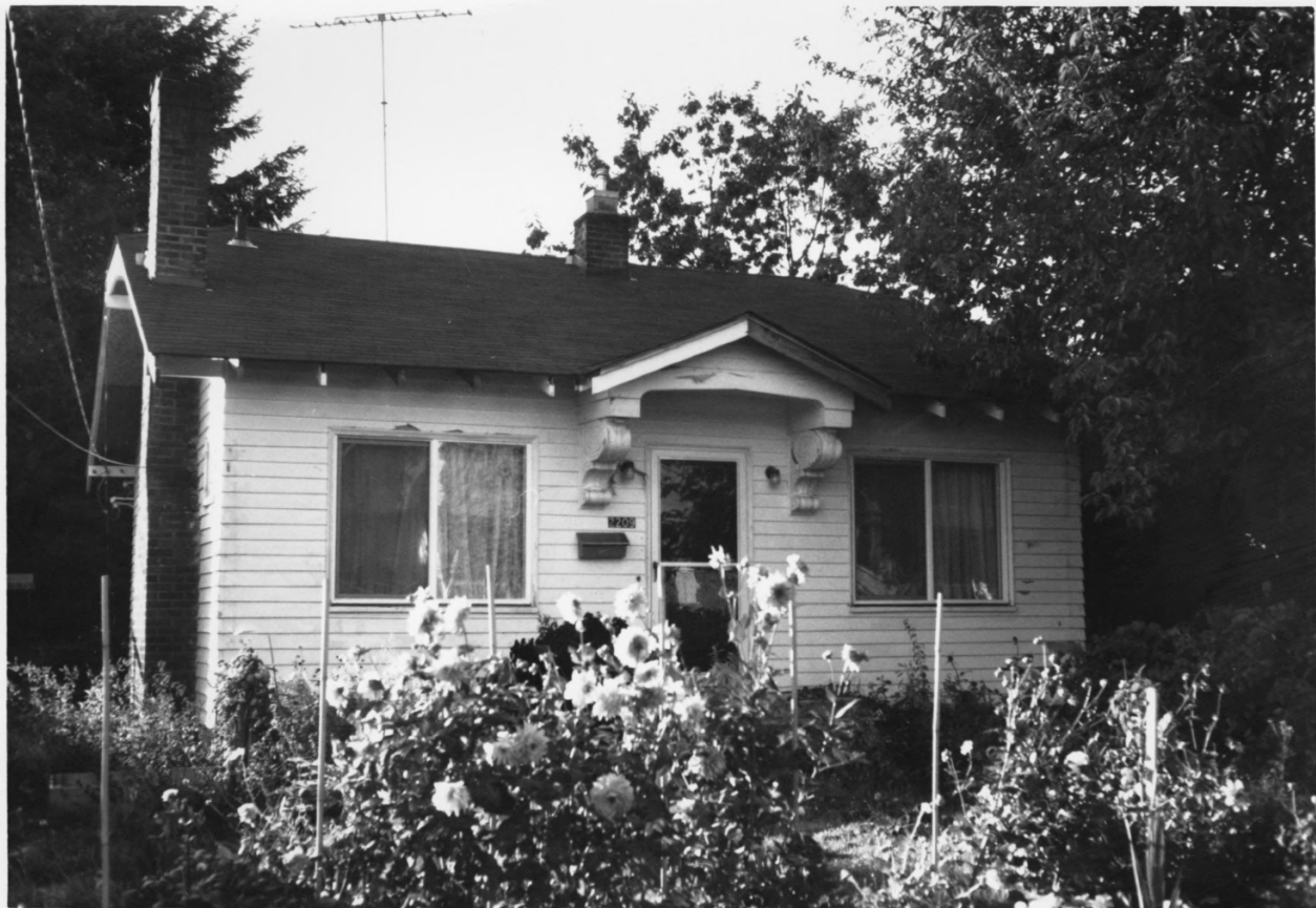
2209 S. WASHINGTON, EAST FACADE, S. CAPITOL NEIGHBORHOOD H.D., # 7
