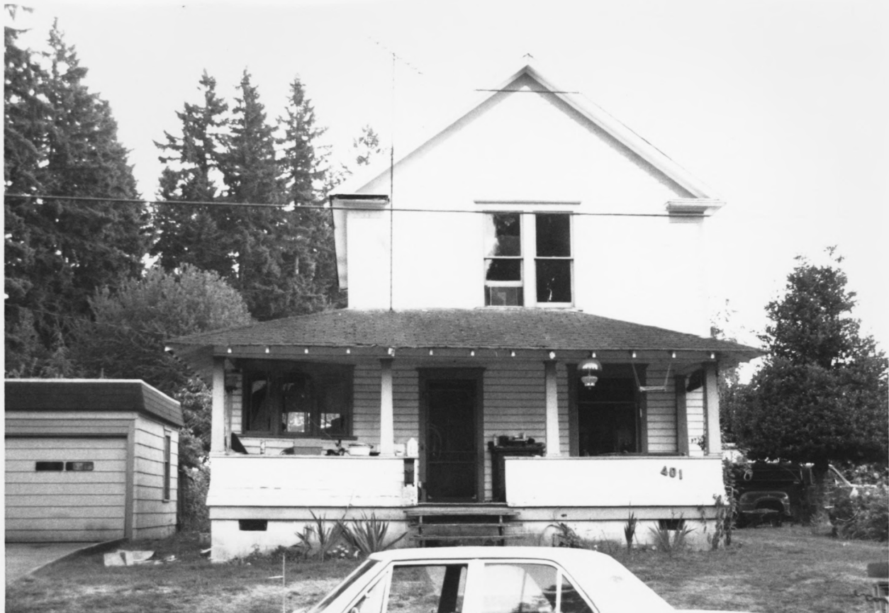
401 E 21ST, NORTH FACADE, S. CAPITOL NEIGHBORHOOD H.D., # 22
