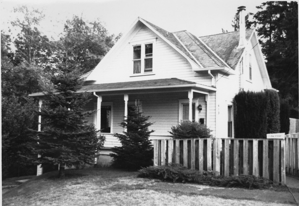
413 E. 21ST, NORTH FACADE, S. CAPITOL NEIGHBORHOOD H. D., #23
