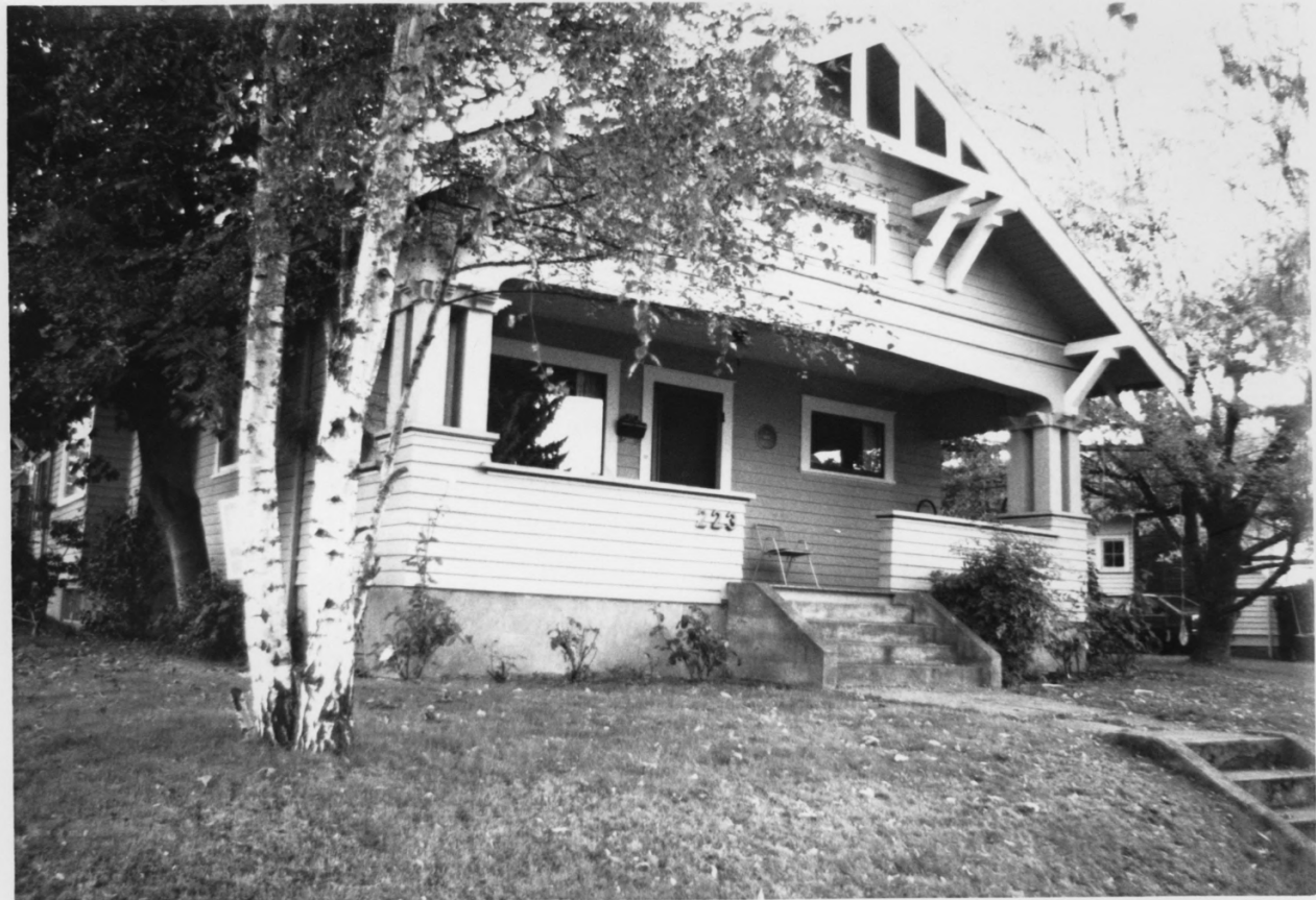
223 E. 18TH, NORTH FACADE, S. CAPITOL NEIGHBORHOOD H.D., #33
