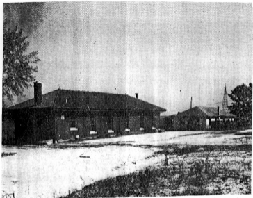
TRANSMITTING AND RECEIVING STATION —Within the walls of these two buildings some of the first commercial trans-Atlantic messages were sent and received by the Marconi company. In the background behind the white building to the right is one of the six towers constructed by the Marconi company in 1913. The tower is now United States government property, and is used by Evans laboratories.
