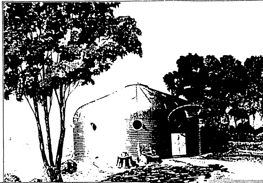
Converted grain bin redesigned by R. Buckminster Fuller for major housing use in the United States.
