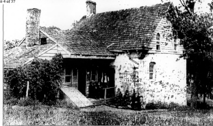
"Lafayette House." An historic dwelling converted to the use of the Staff erecting the New Brunswick Station.
