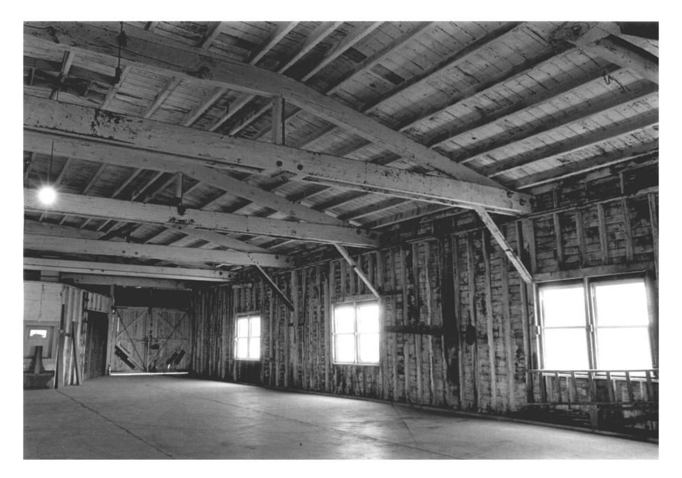
8 of 13 Note roof trusses Interior view: looking south to automobile entrance at front of upper story. Concrete floor poured in 1923
