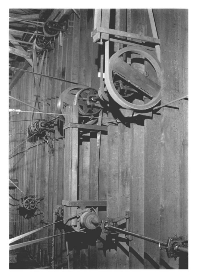
13 of 13 Interior view: detail of overhead line shafting, belts and pulleys driven by electric motor to operate equipment
