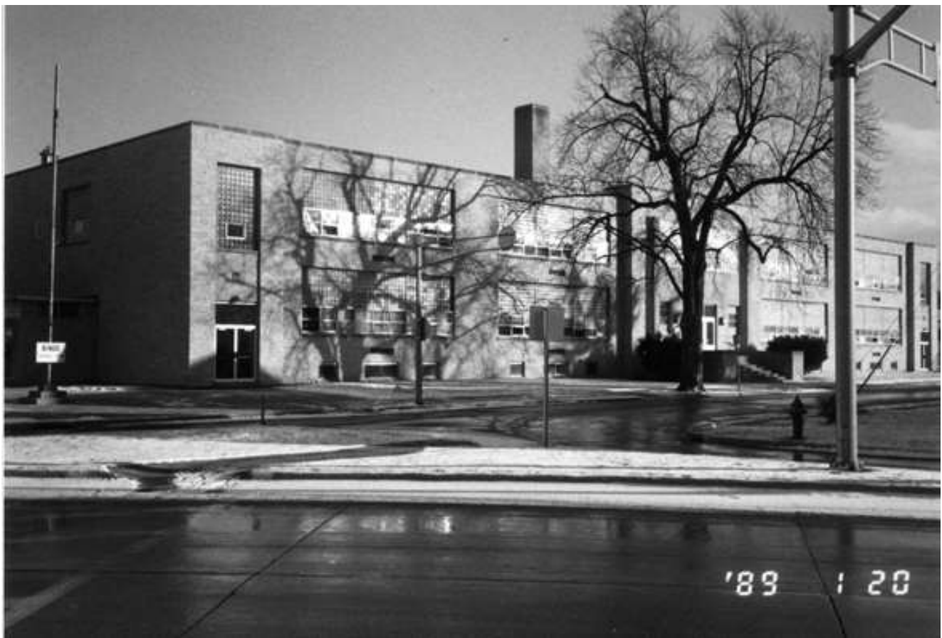
Figure 9: The St. Mary School in 1989, showing glass-block transoms. Wisconsin Architecture and History Inventory, accessed July 26, 2016.
