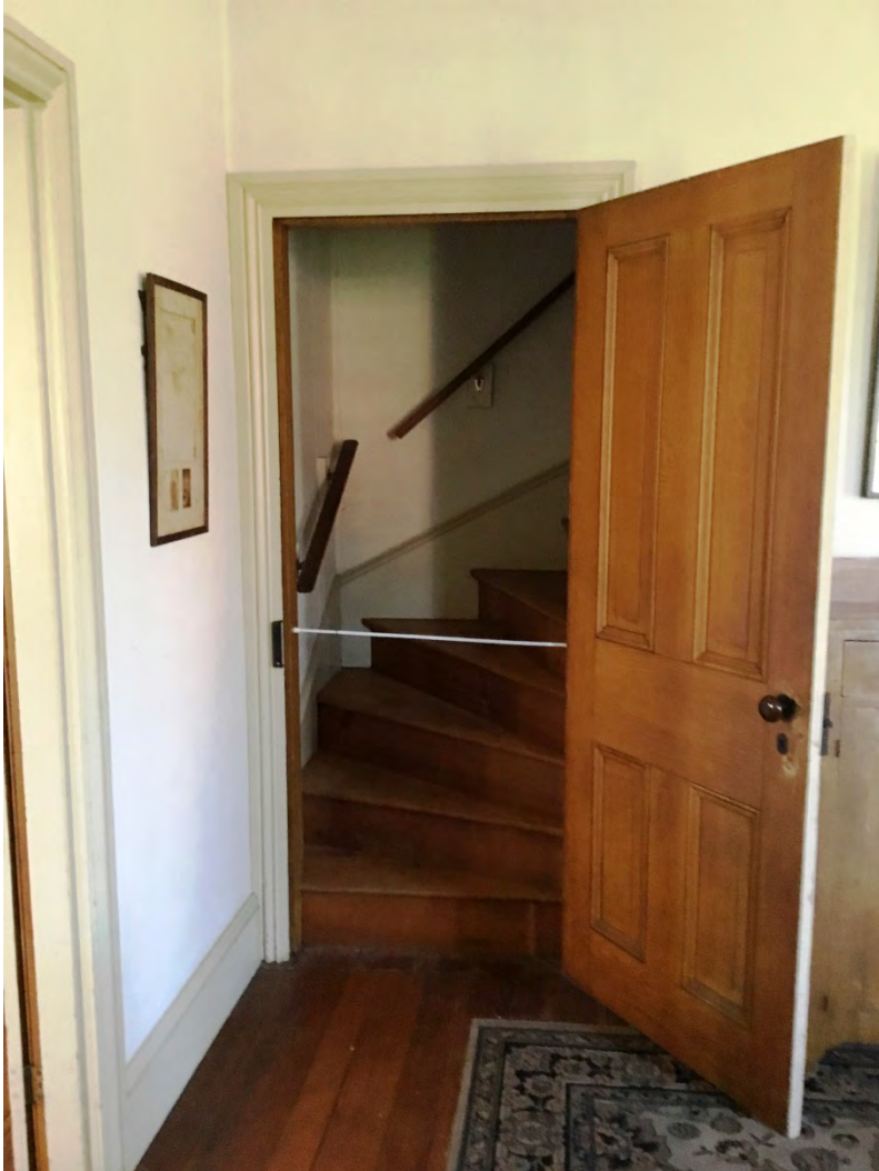
House Photo 6 of 15 1 st floor. Northeast room back stairs entrance facing south
