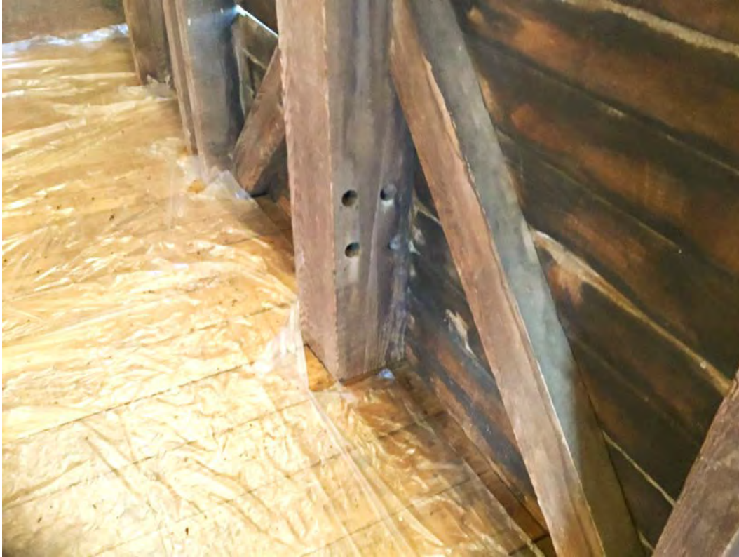
Barn interior 4 of 17. Trusses above bank doors facing north.
