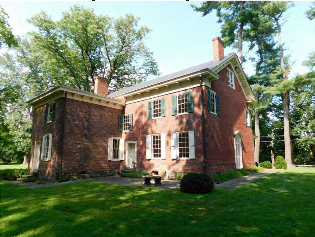
3 of 18. View of rear of house from southwest facing northeast
