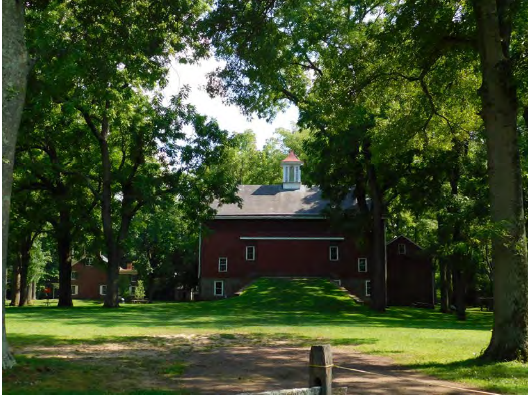
15 of 18. View of bank side of barn facing south
