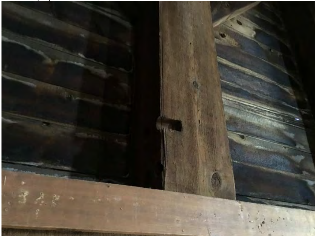
Barn interior 2 of 17. Post in west gable with wicket hole facing east
