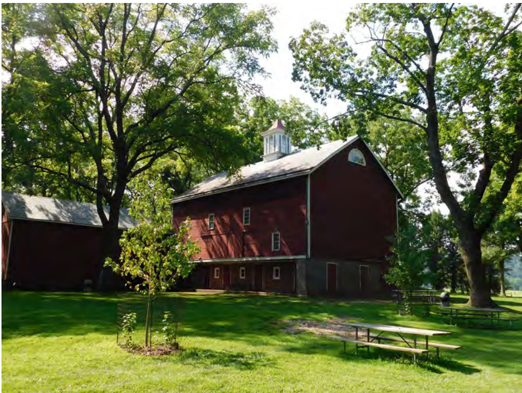
16 of 18. View of southeast corner of barn and wing facing northwest
