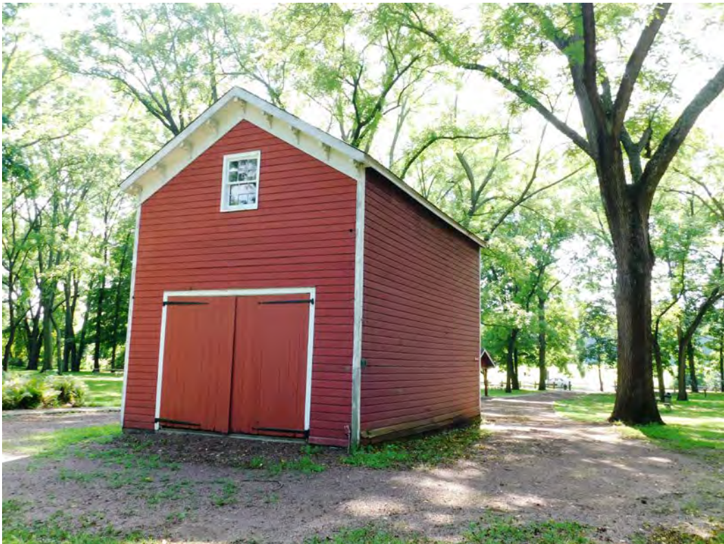
11 of 18. View of northeast corner of carriage house/wagon house facing southwest
