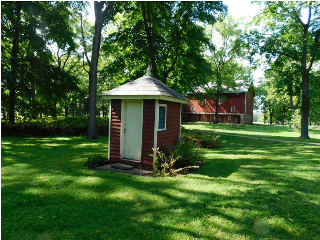
7 of 18. View of privy facing northwest
