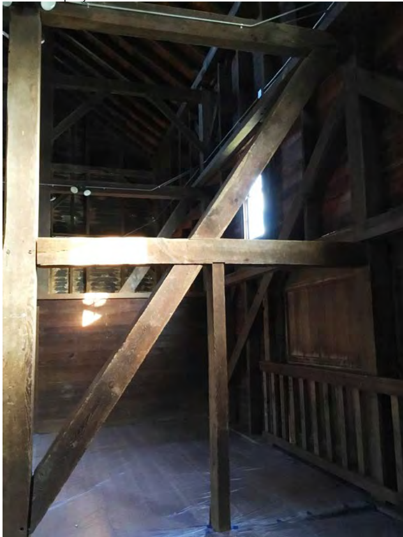
Barn interior 3 of 17. Passing brace in central bent facing east
