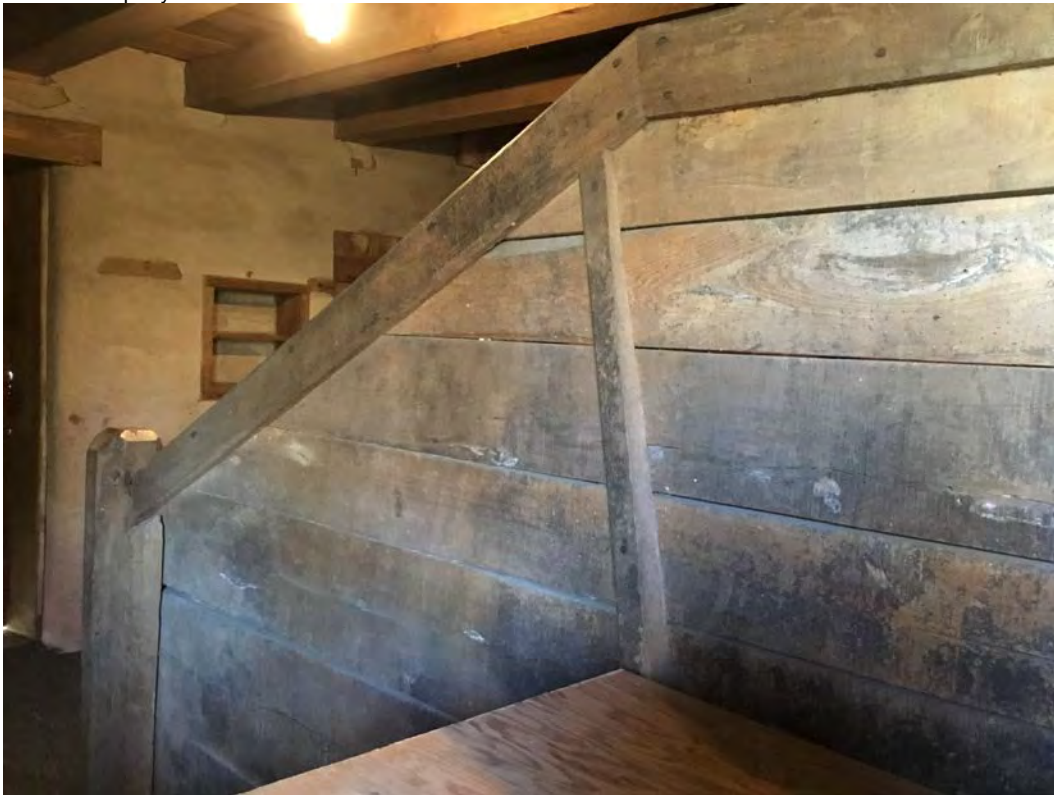
Barn interior photo 12 of 17. Stable level wooden horse stall partition facing south
