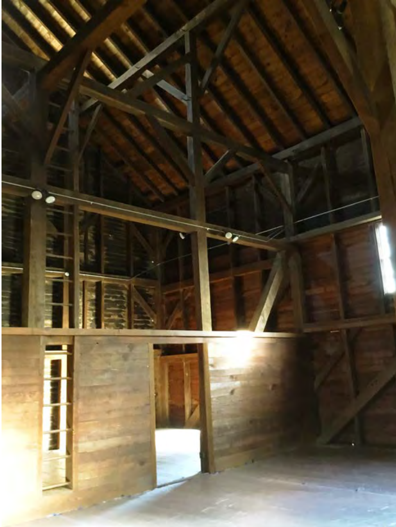
Barn interior photo 7 of 17. Mowstead wall facing southeast
