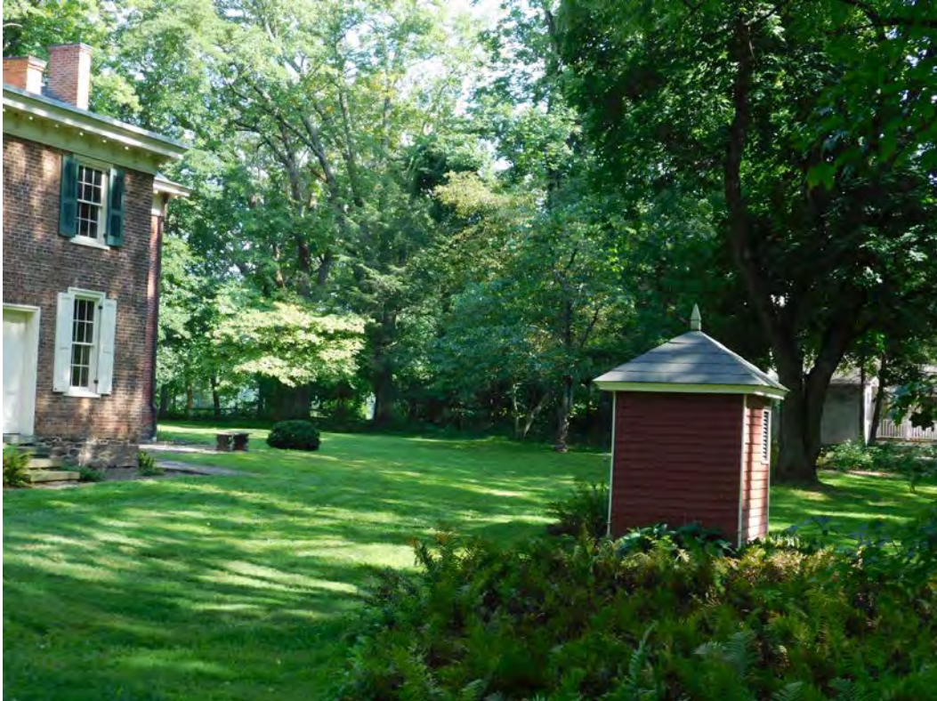
8 of 18. View of privy in relation to the rear of the house, facing south.
