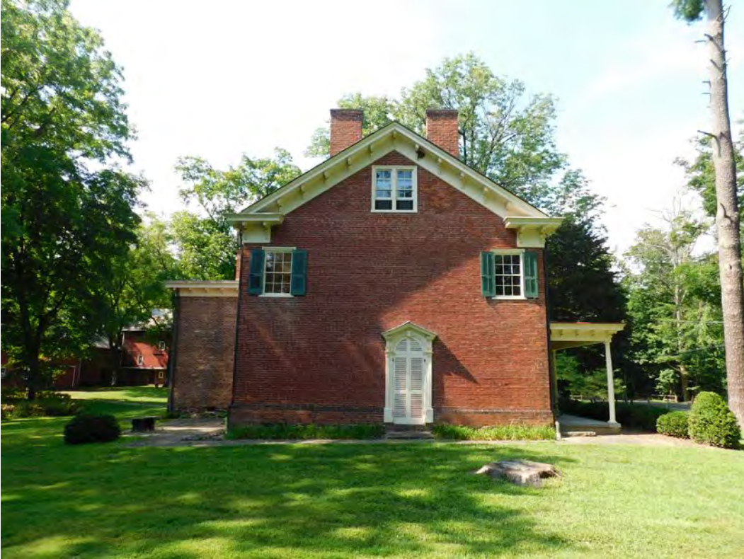
2 of 18. View of south gable end of house facing north
