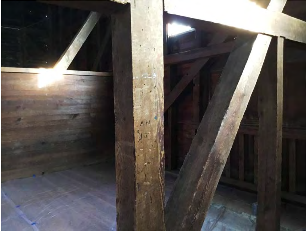
Barn interior photo 6 of 17. Mowstead post showing nail holes from original wall
