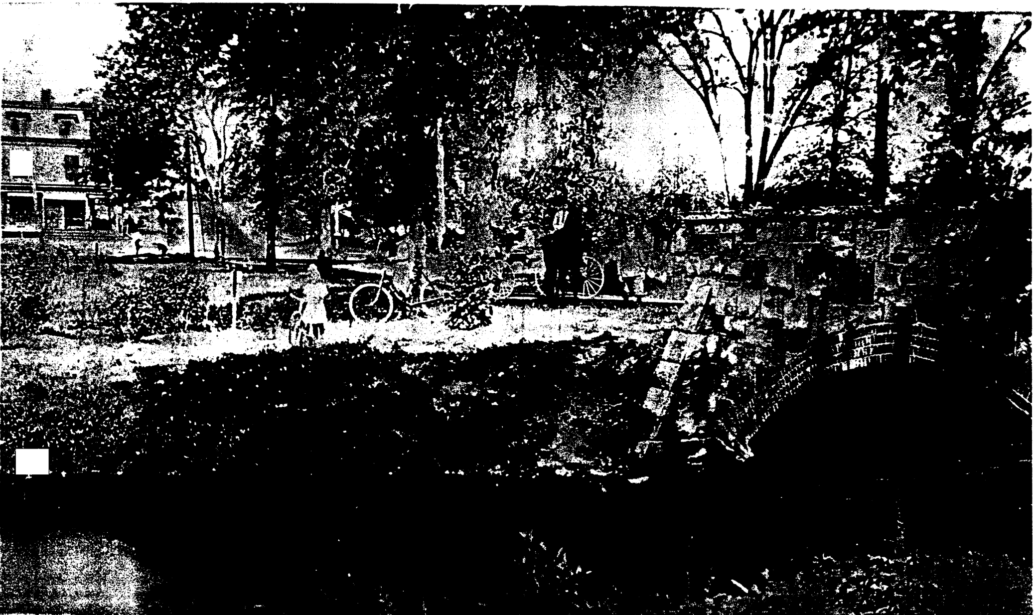
HARDENBURG AVE. LOOKING WEST FROM STONE BRIDGE
