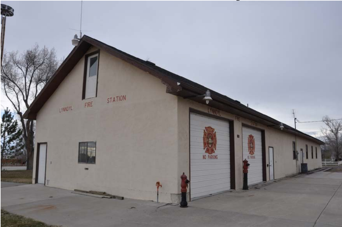
Photo No. 5. South and east elevations of 1983 section. Camera facing northwest.
