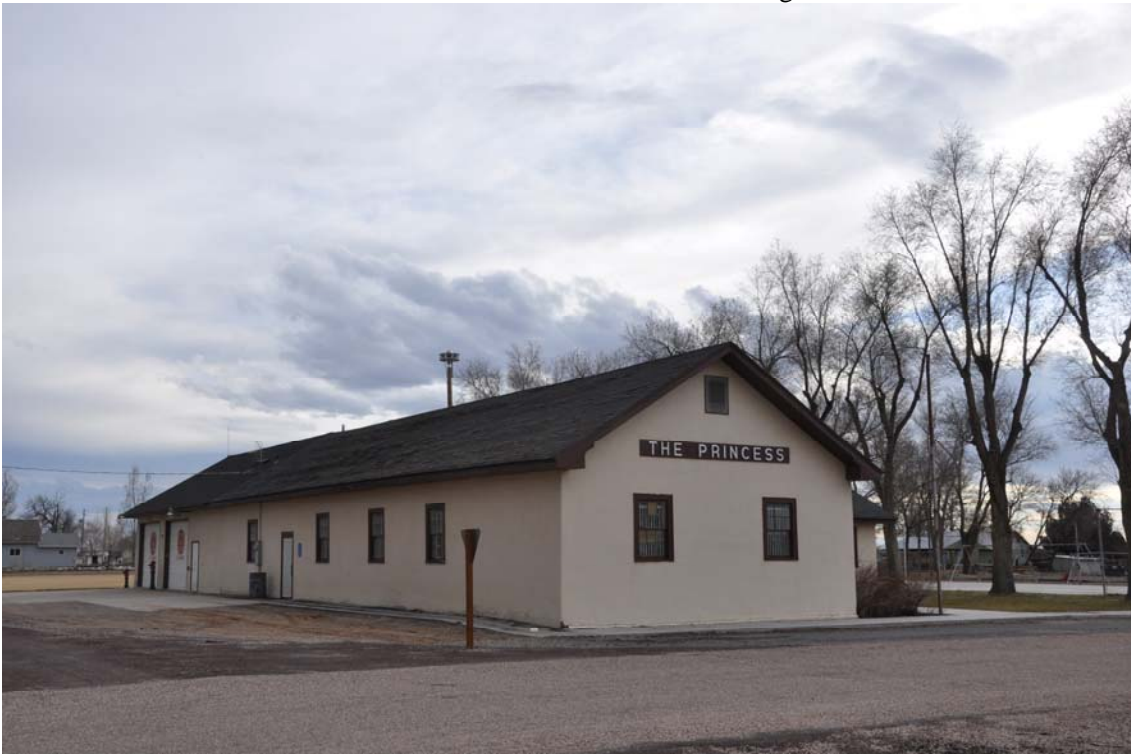
Photo No. 6. North and east elevations of 1914 section. Camera facing southwest.
