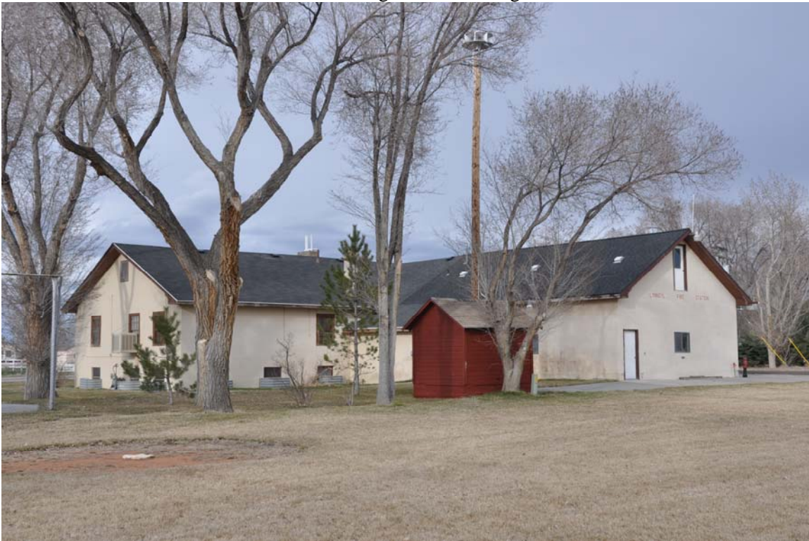
Photo No. 8. South and west elevation of building. Camera facing northeast.
