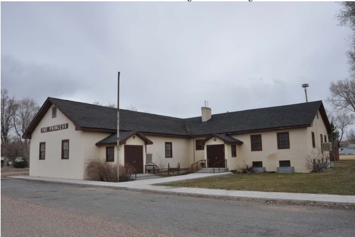
Photo No. 7. North and west elevations of building. Camera facing southeast.
