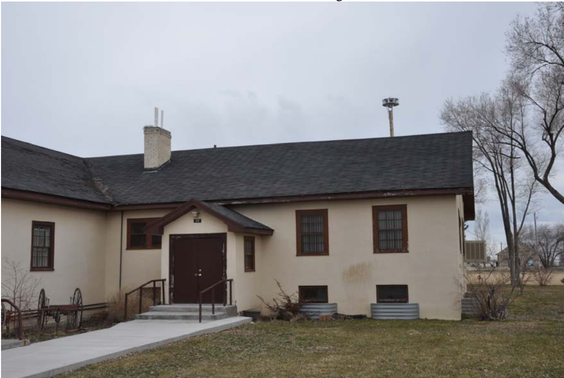
Photo No. 2. North elevation of 1936 section. Camera facing south.
