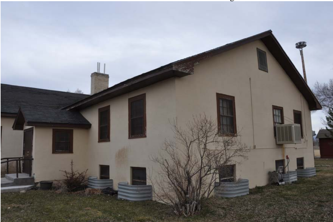
Photo No. 3 North and west elevations of 1936 section. Camera facing southeast.
