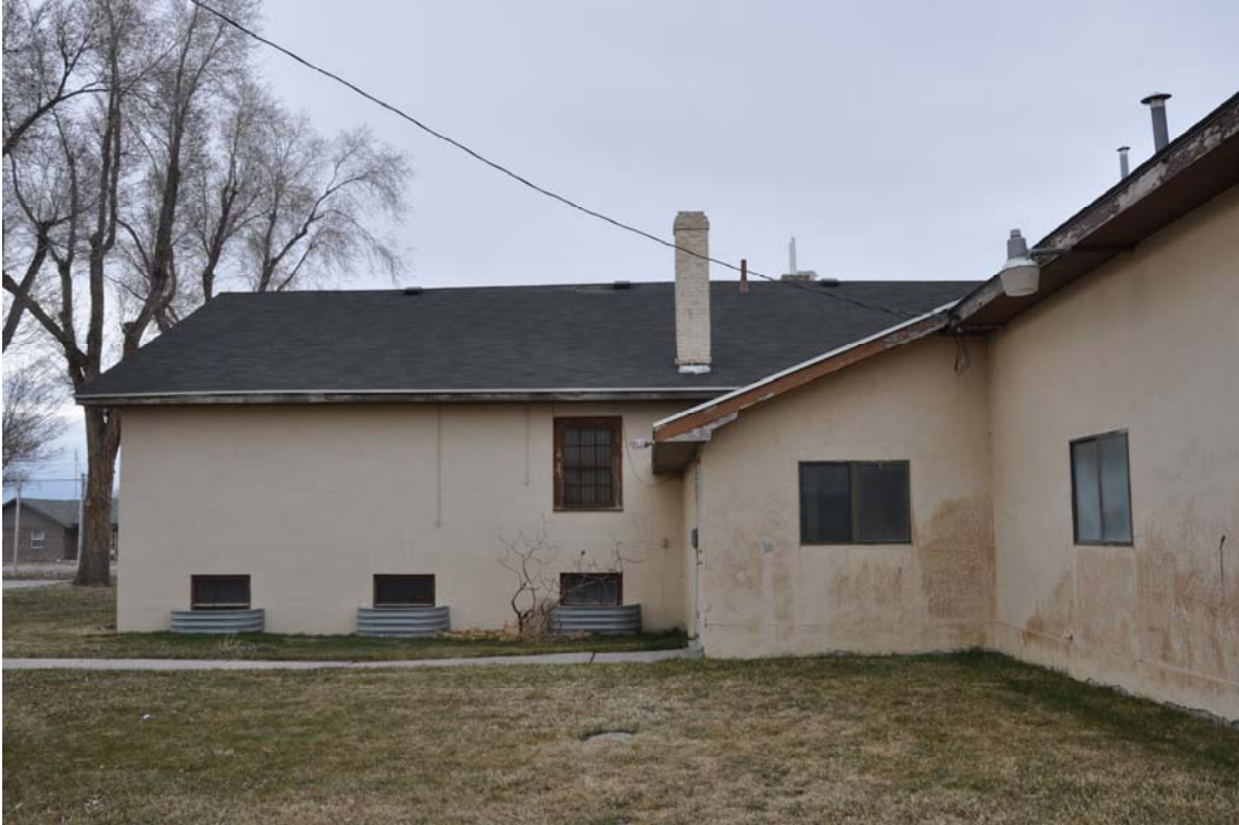
Photo No. 4. South elevation of 1936 section (left) and west elevation of 1983 section (right). Camera facing north.
