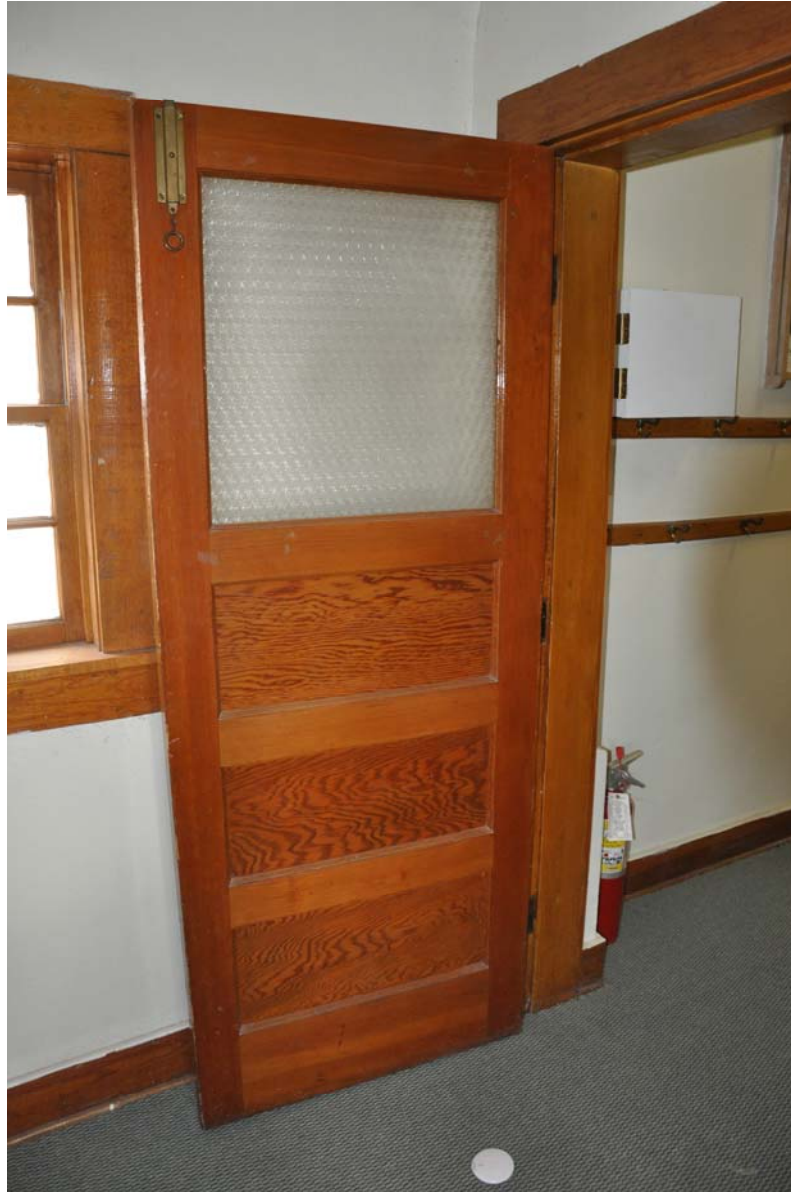
Photo No. 15. Door—typical finish for interior trim. Camera facing southwest.
