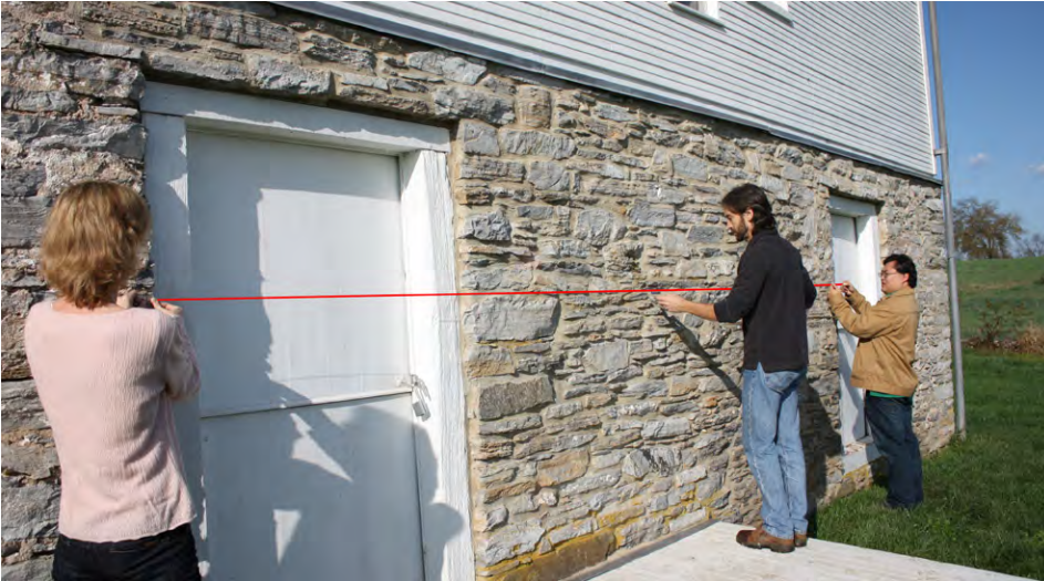
Creating a datum using a line level, Secondary House
