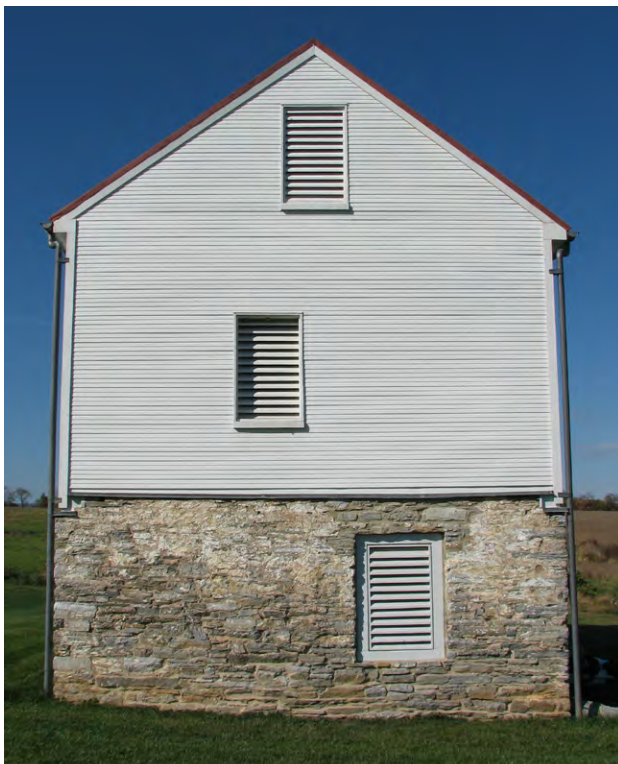
South Elevation, Secondary House
