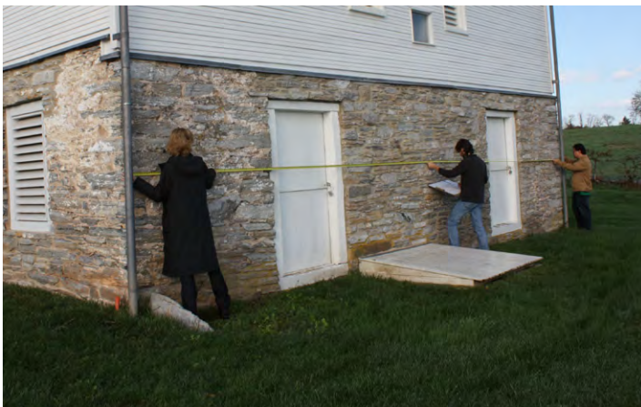
Measuring the first floor plan, Secondary House
