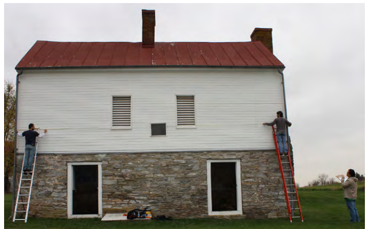
Measuring the second floor plan, Secondary House.
