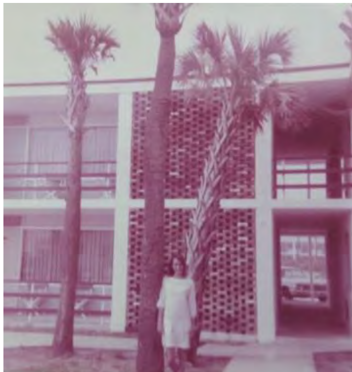
Figure 2: Brick lattice work, date unknown.
