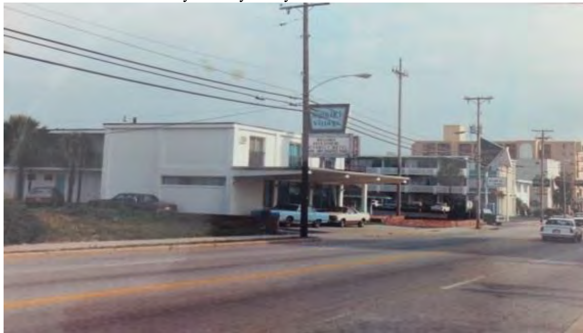
Figure 3: Original location of sign, c. 1985
