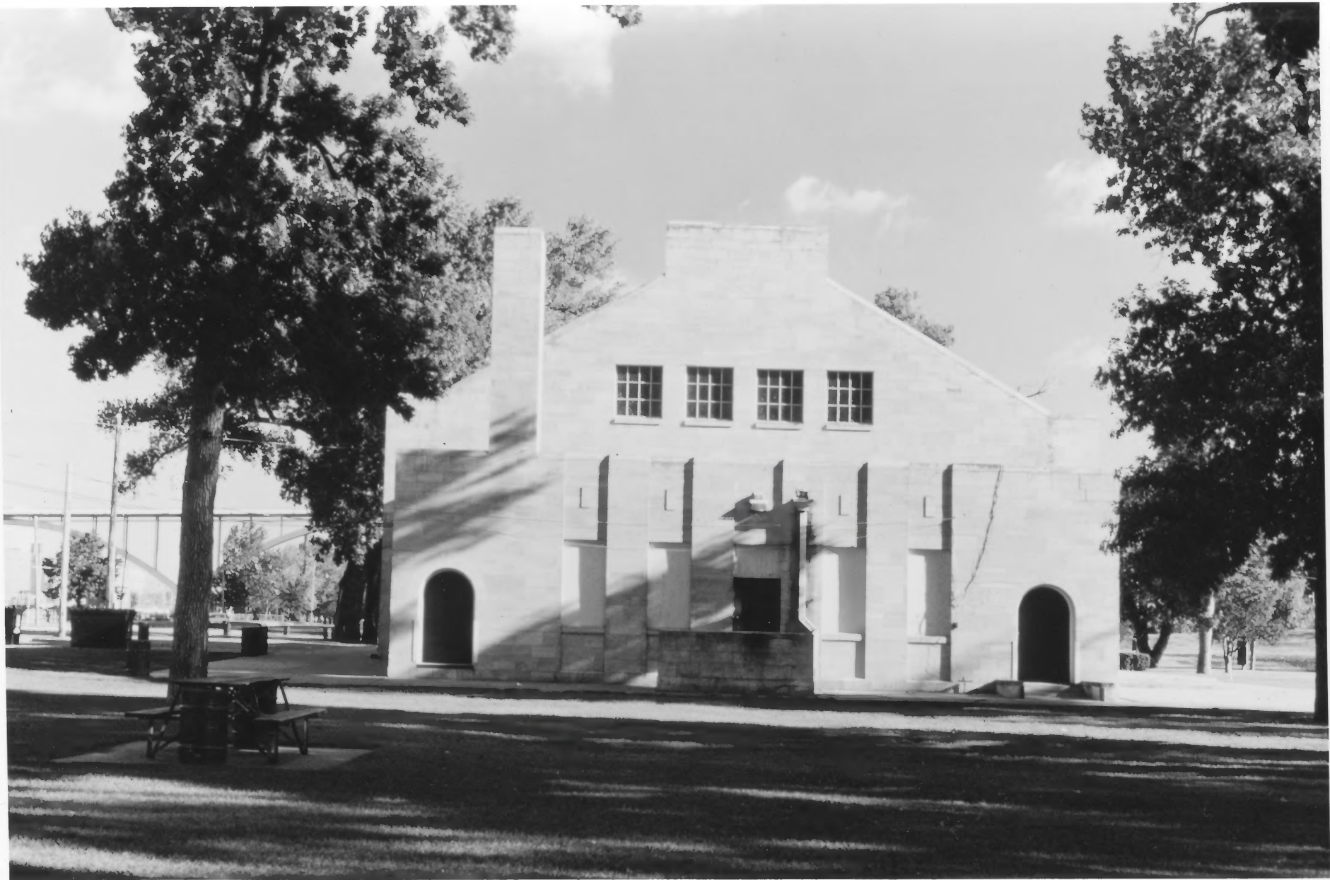
HARRIET ISLAND PAVILION ST. PAUL, RAMSEY COUNTY, MINNESOTA NO PHOTO I.D. NUMBER
