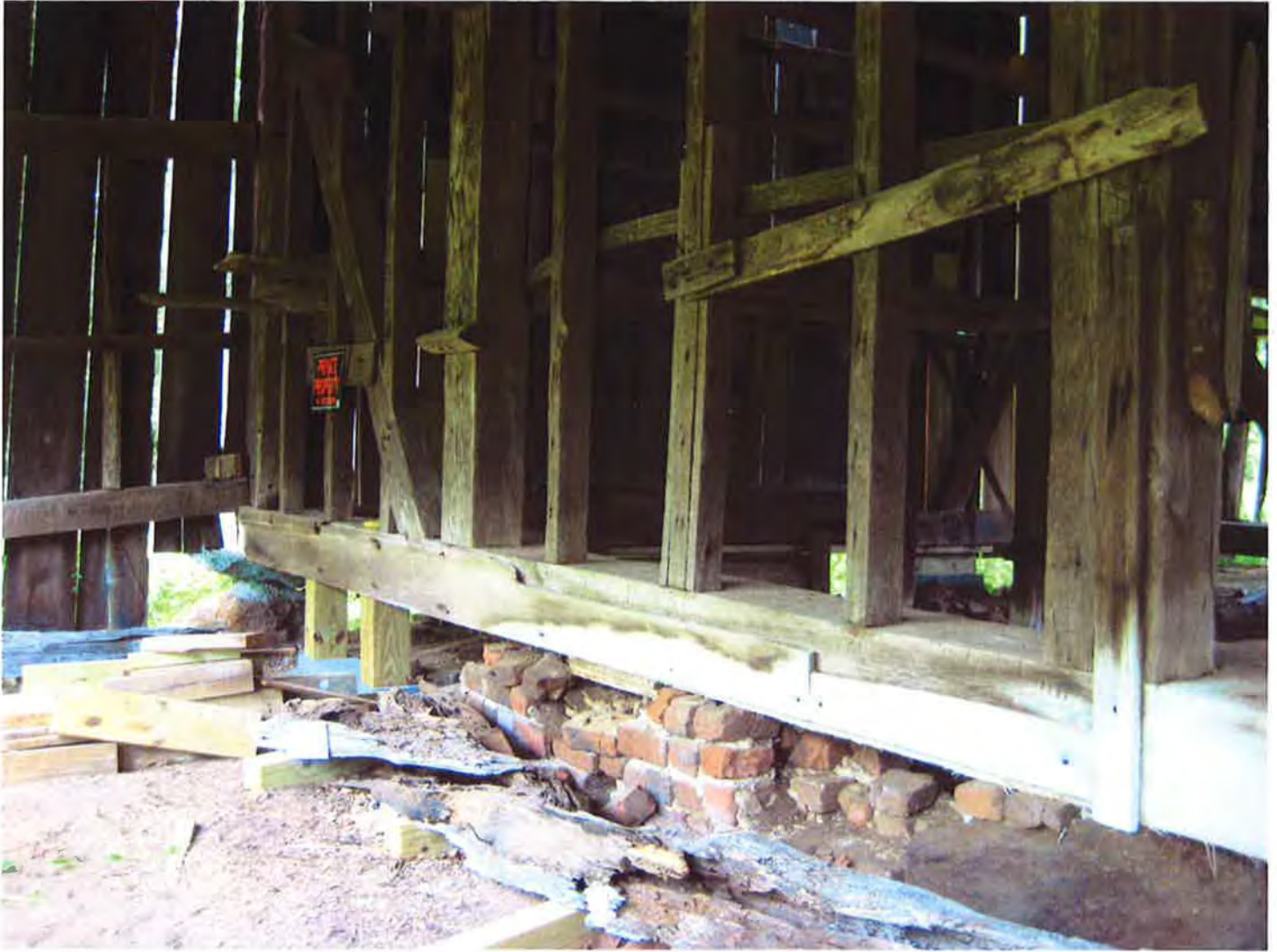
Interior framing and foundation detail, view from southeast, 8/11/2014
