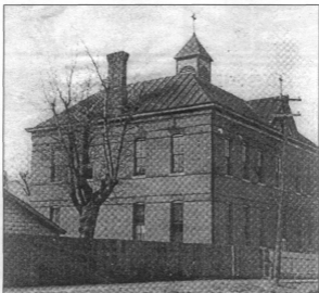
Figure 14: St. Mary's School (1894), view southwest, c. 1914
