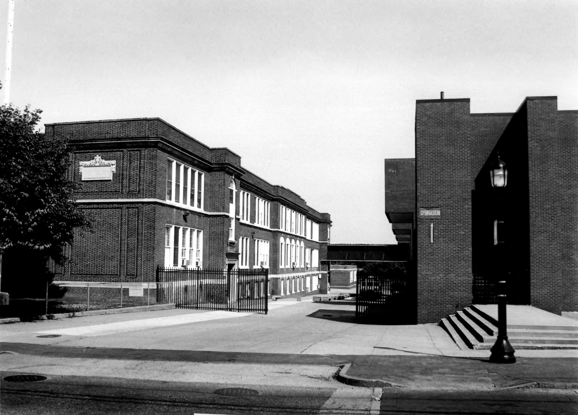
Photo 2. Howard High School South side elevation with walkway to new building
