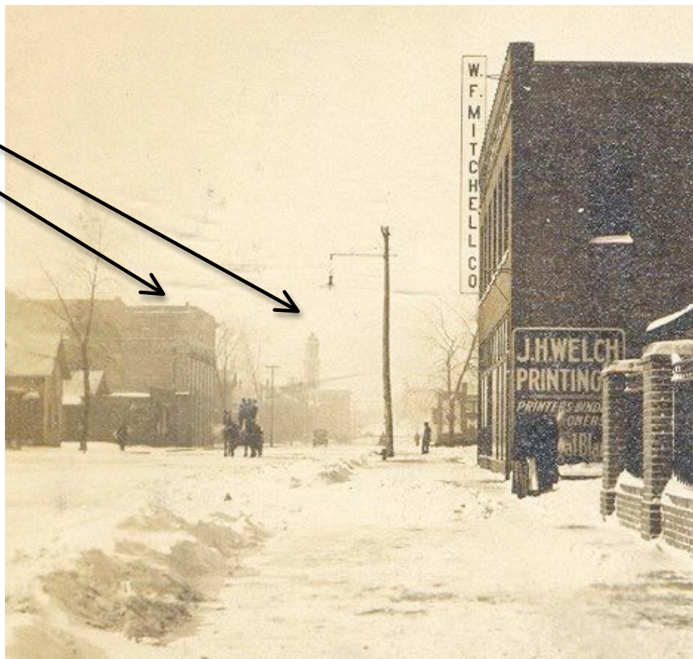
Figure 6: HISTORIC IMAGE – 1300-1400 Locust Street, January 1916
