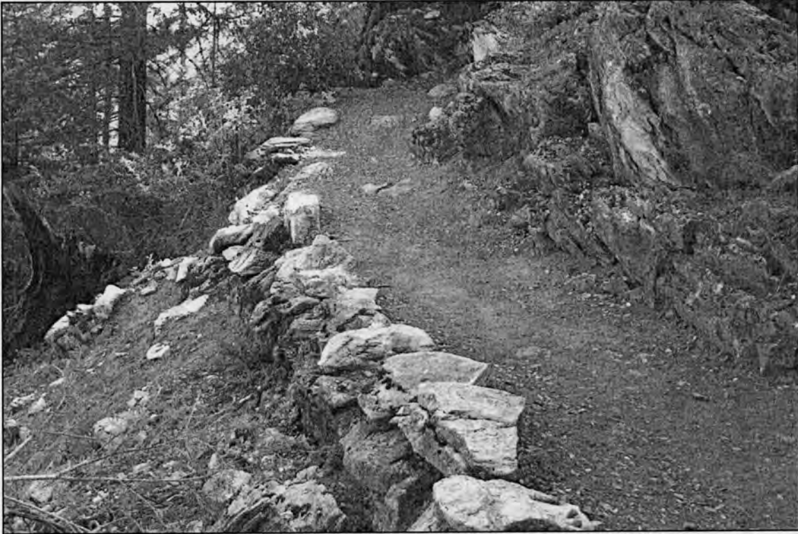
Photo 9 of 12: (OR_Josephine County_OregonCavesHistoricDistrictBoundaryIncrease_0009) Benching on Cliff Nature Trail, camera facing east
