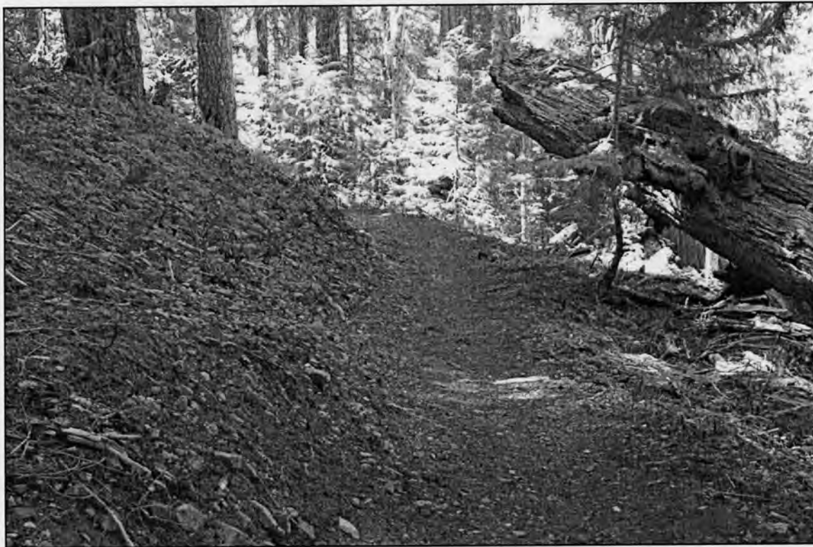
Photo 4 of 12: (OR_JosephineCounty_OregonCavesHistoricDistrictBoundaryIncrease_0004) Lake Mountain Trail, showing slope treatment, camera facing north
