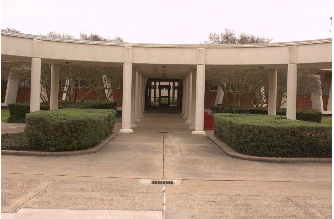
Photo 4 Northwest entrance. Camera facing Southeast.
