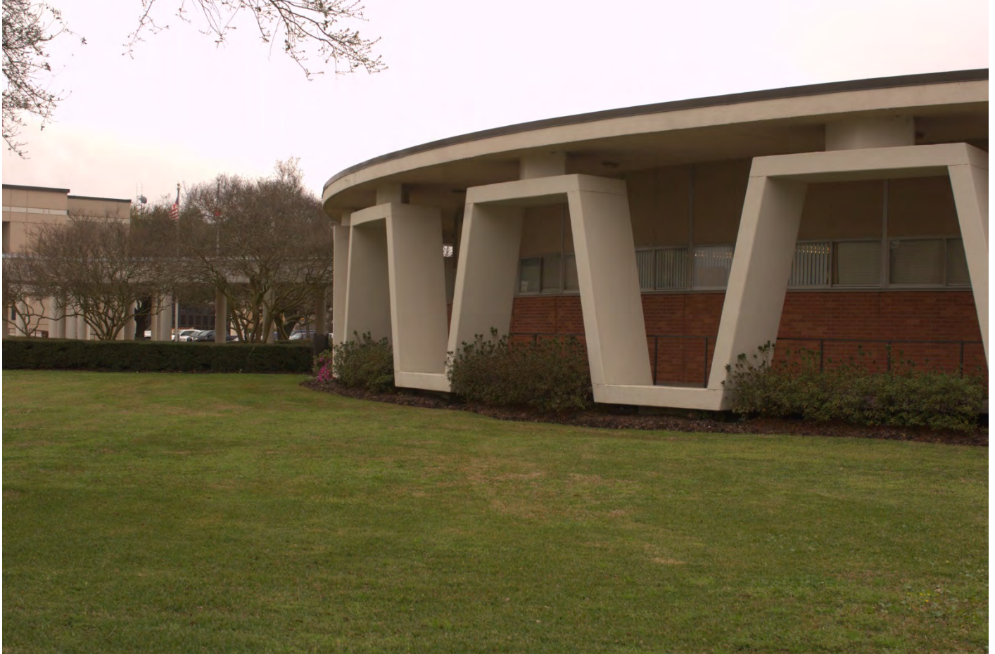
Photo 3 West side. Camera facing North.
