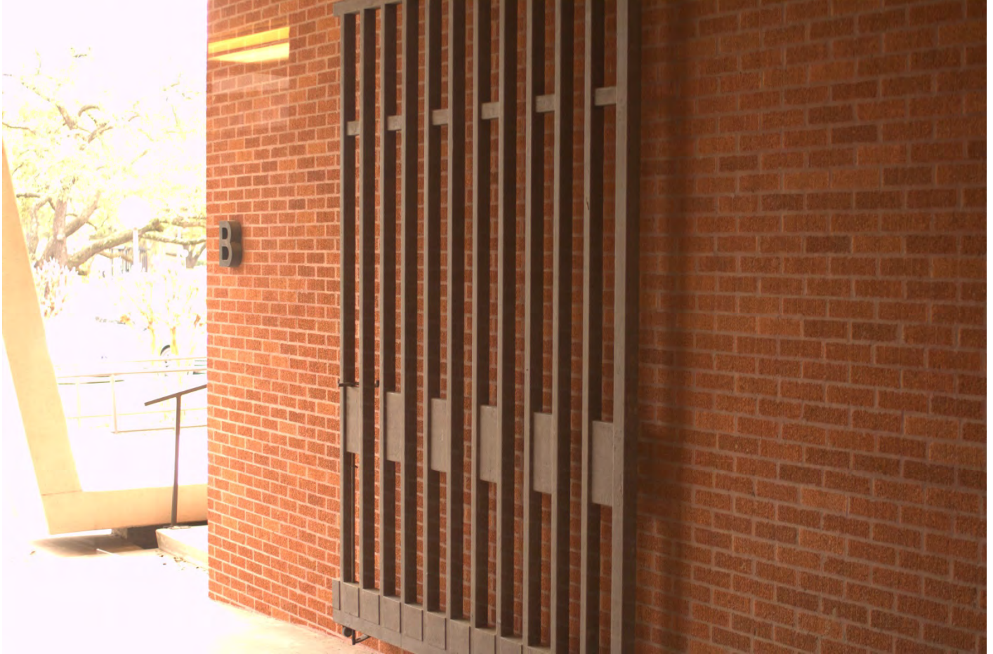
Photo 11 South entrance gate. Camera facing Southwest.
