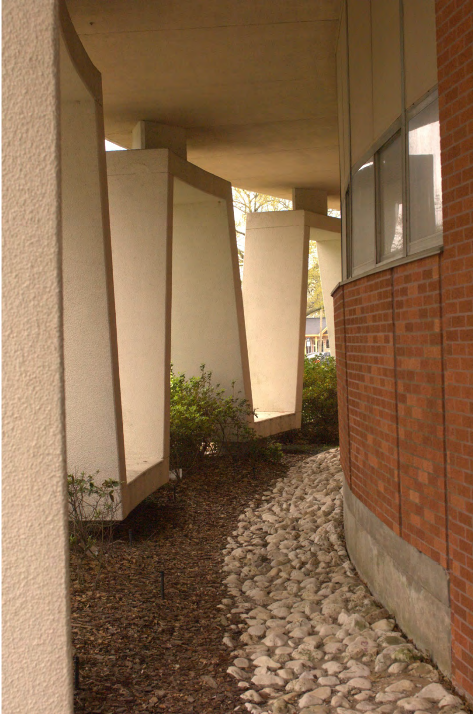
Photo 7 Eastside exterior detail. Camera facing south.
