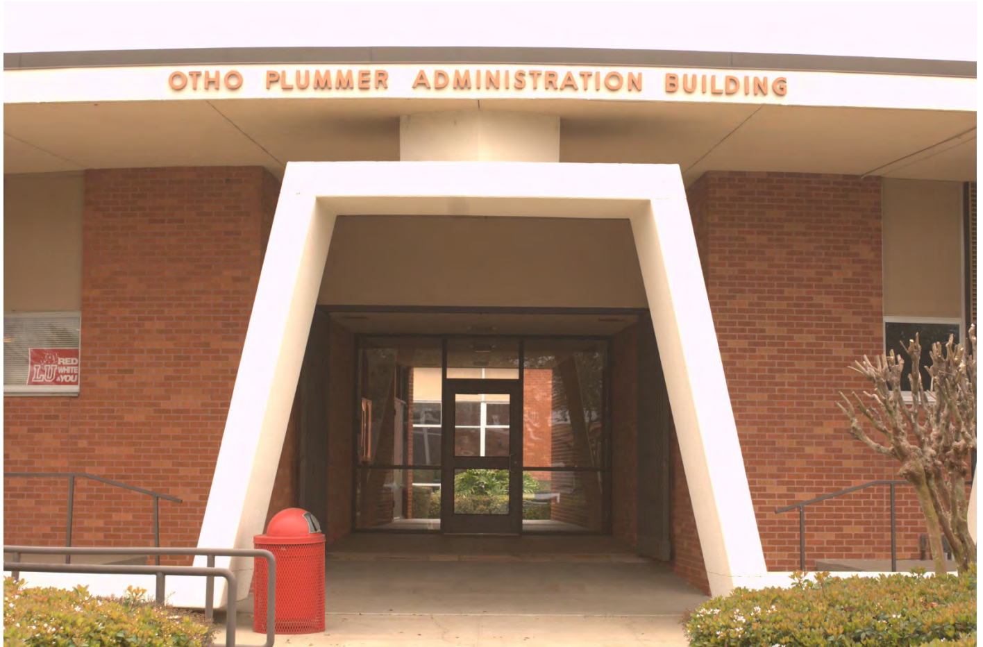
Photo 2 South entrance. Camera facing North.
