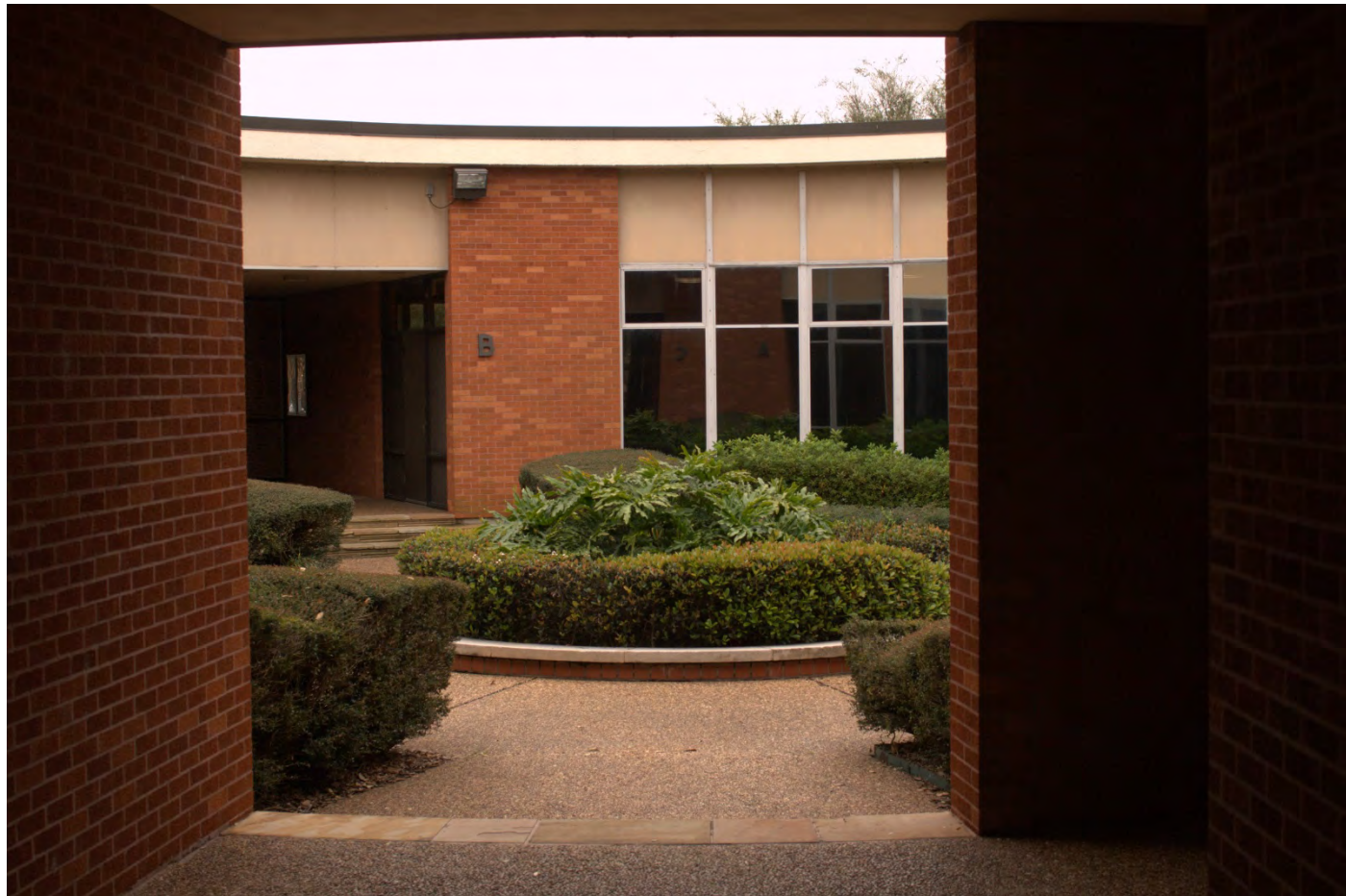
Photo 8 Interior courtyard. Camera facing Southwest.
