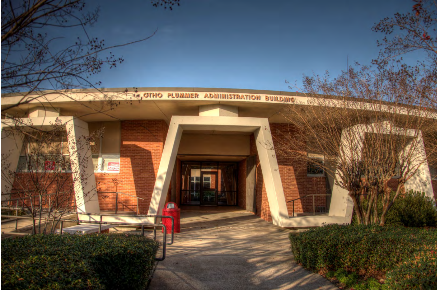
Photo 12 South Entrance. Camera facing North.
