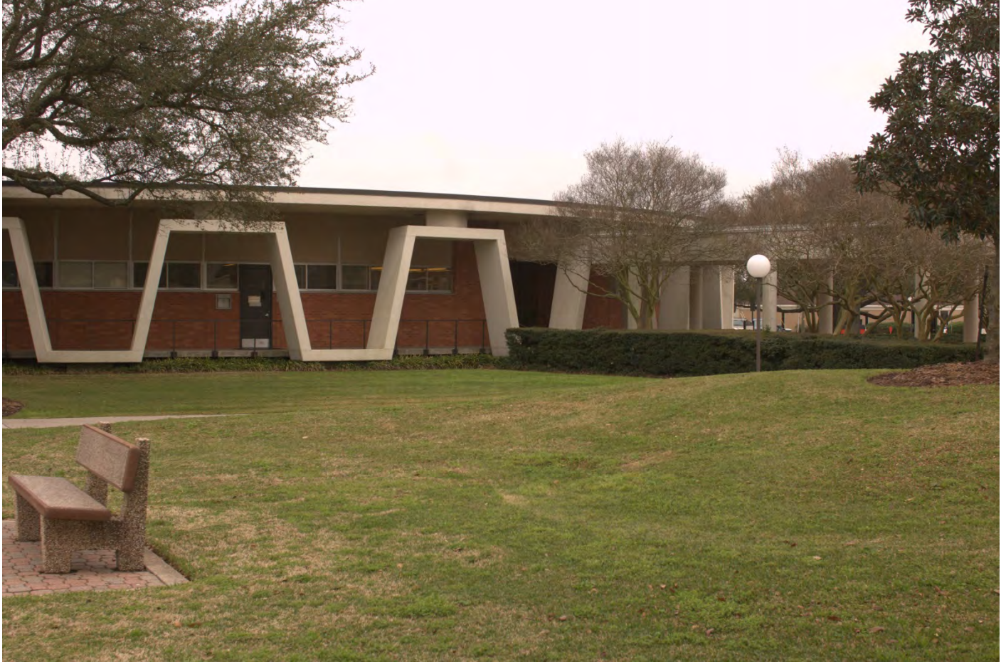
Photo 5 North side. Camera facing South.
