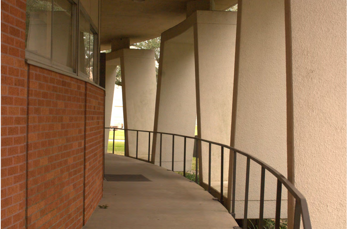
Photo 6 Exterior walkway, Northeast side. Camera facing Northwest.
