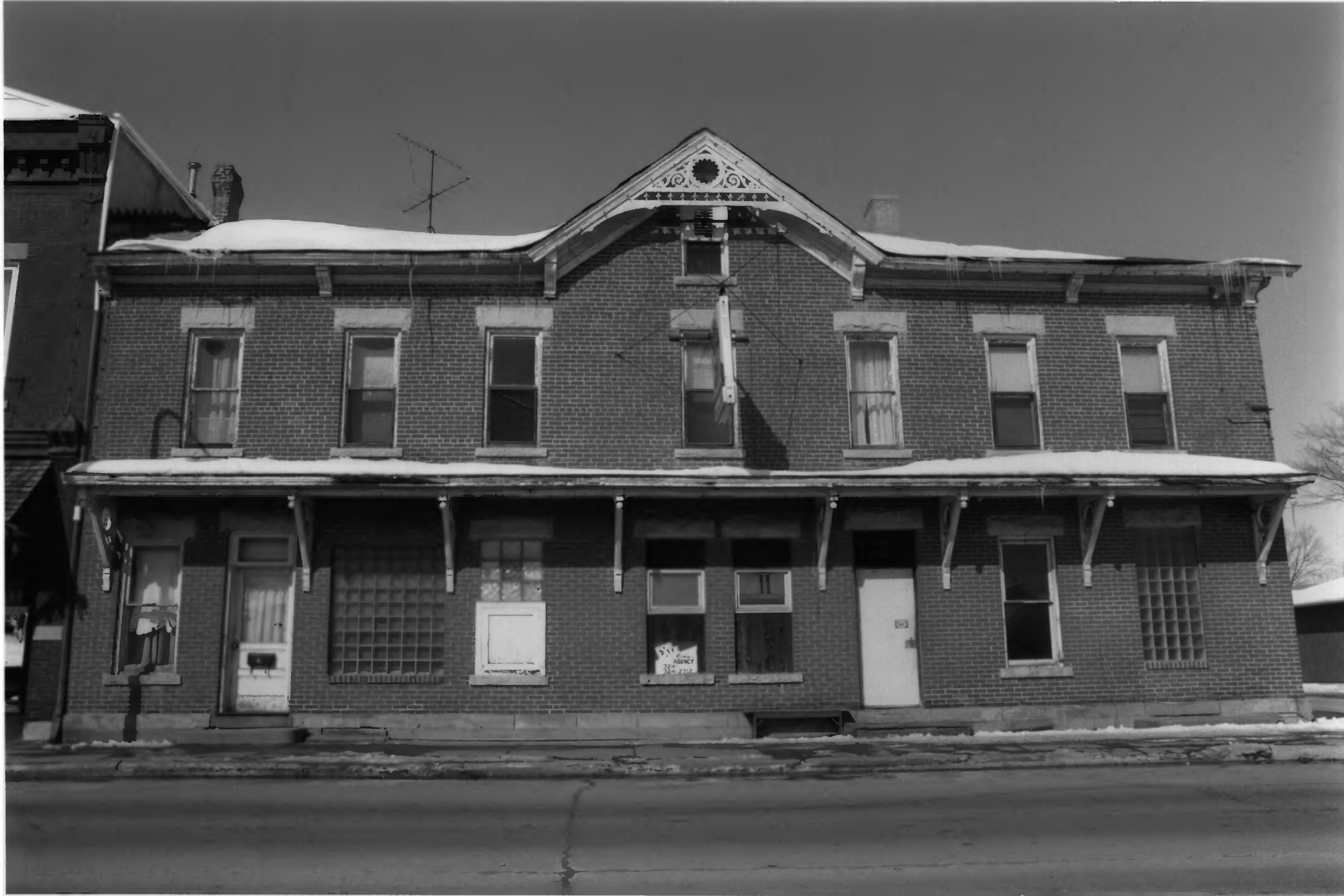
Spafford Williams House Caledonia Commercial Historic District Houston Co., MN 011562-19
