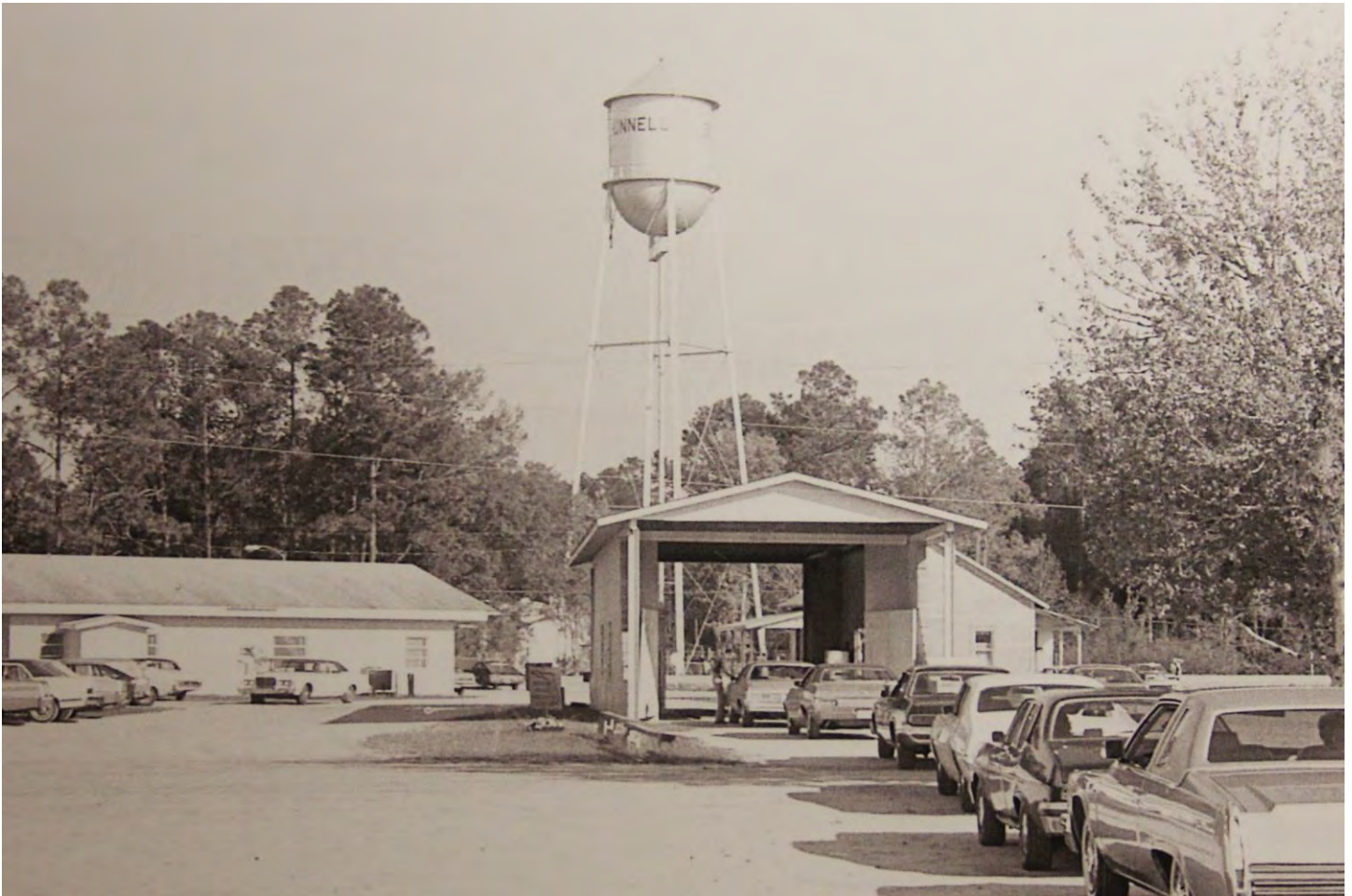
Figure 1: Bunnell Water Tower, December 1980.
