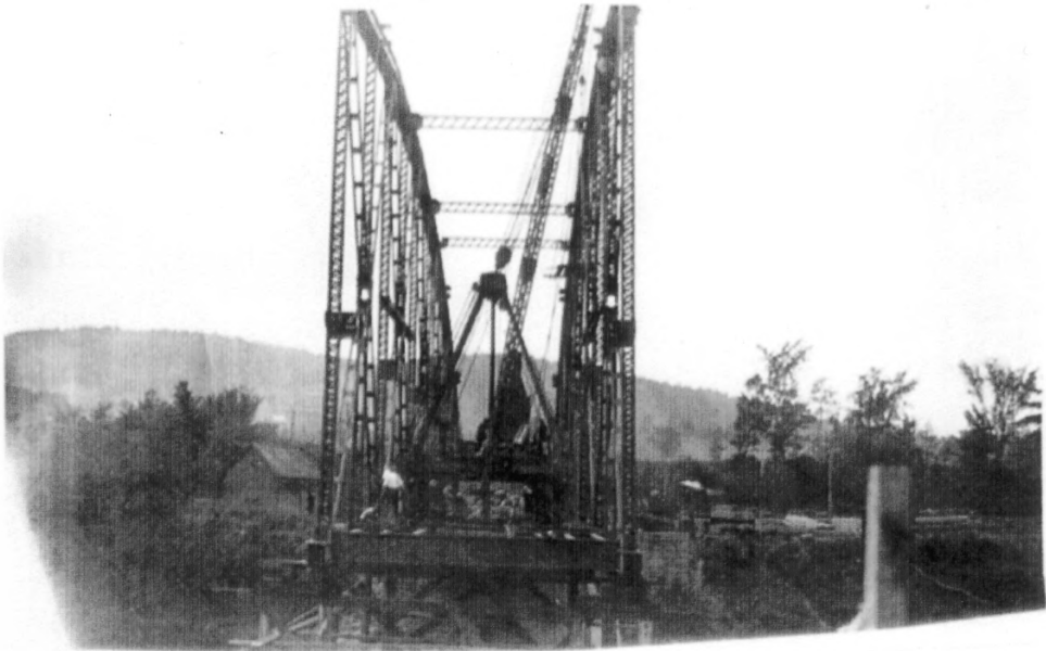
PIERMONT BRIDGE GRAFTON, NEW HAMPSHIRE PHOTO NO-5
