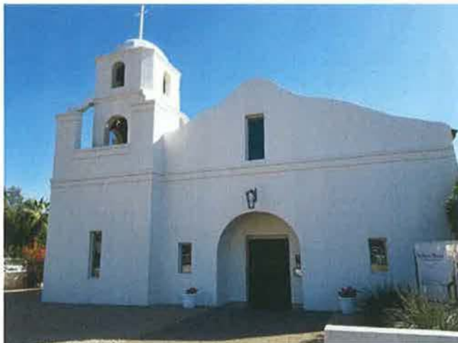
Figure 1: OLPH Mission Church, west façade. Source: Masinelli, 2018.
