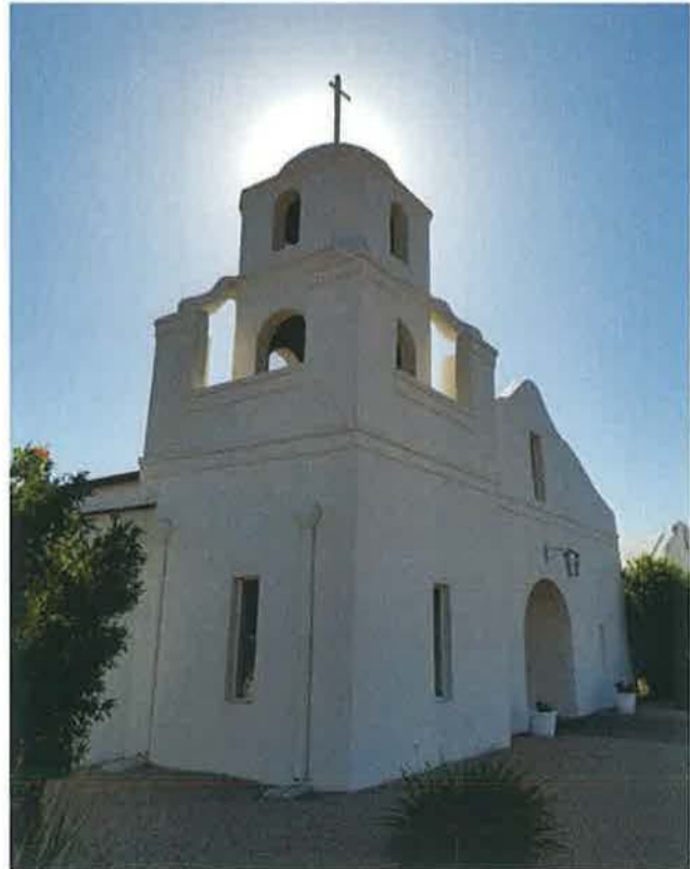
Figure 4. This southeastern view emphasizes the sacristy room at the ground floor topped by the bell tower. Focus is placed on the flying buttresses projecting from the four corners of the bell tower providing the structure with stability. The curvilinear parapet is visible from this view. Source: Masinelli, 2018.
