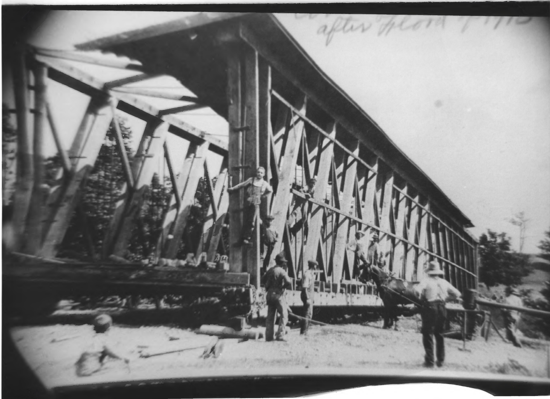
BRINGING BRIDGE BACK AFTER 1913 FLOOD WASHED IT DOWN RIVER
