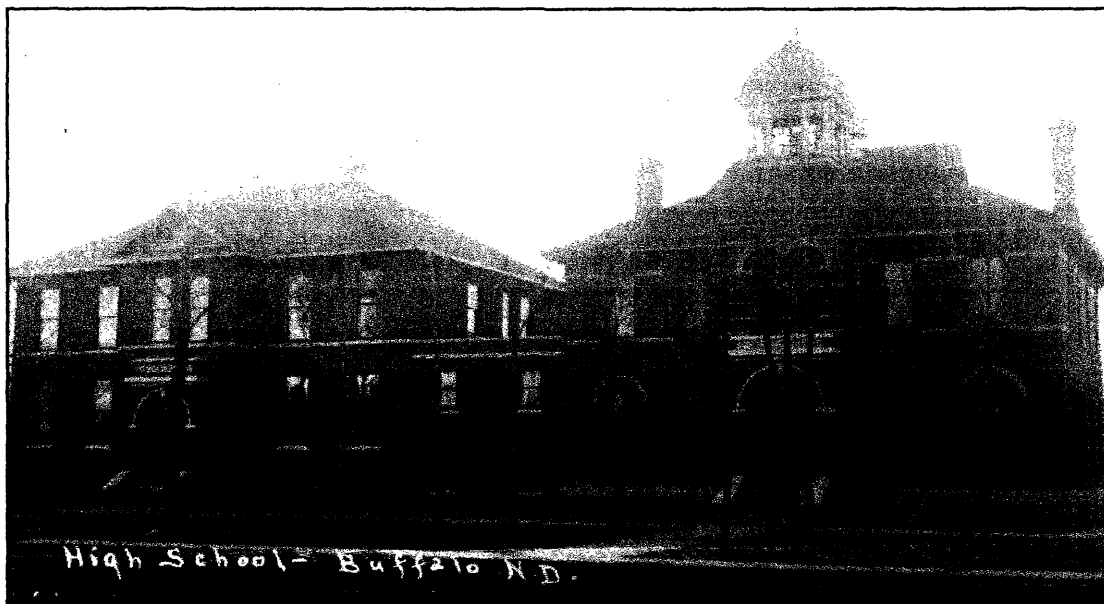
Figure 6. 1916 Buffalo High School constructed next to the 1902 Buffalo Public School.
