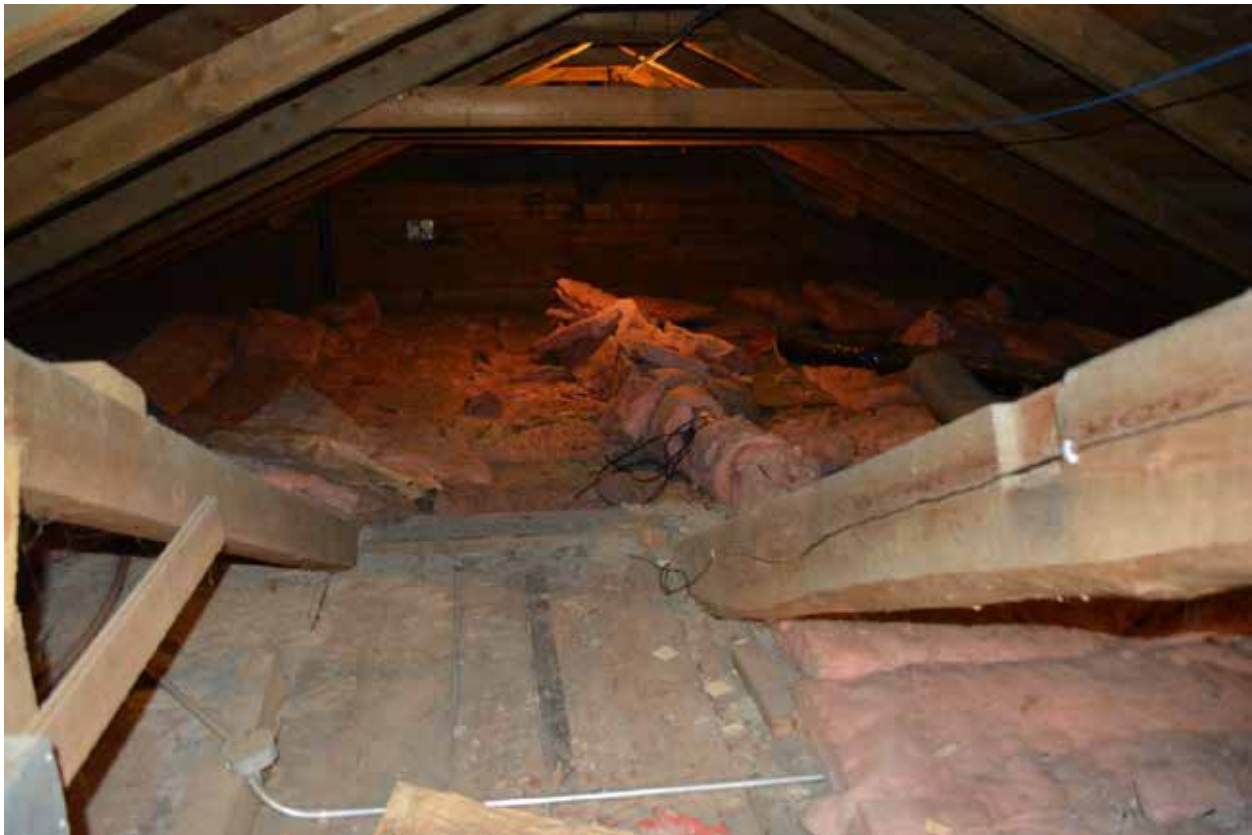
Photo 22: Looking North at north/south gable (attic)
