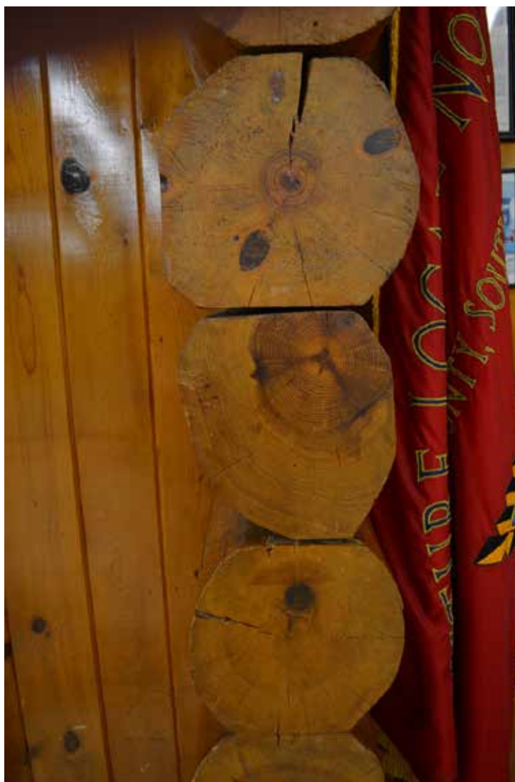
Photo 16: Looking South closeup of crown in main room
