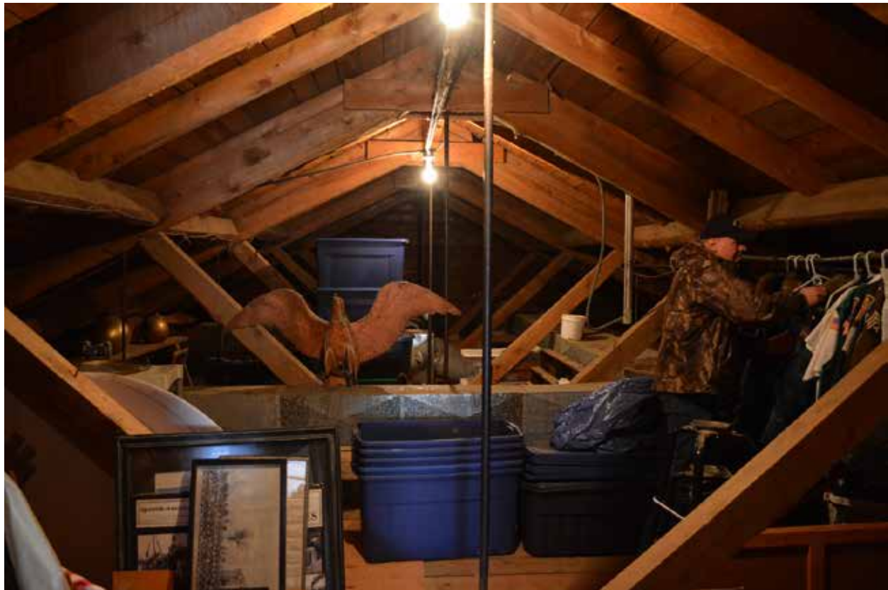
Photo 21: Looking East at east/west gable (attic)
