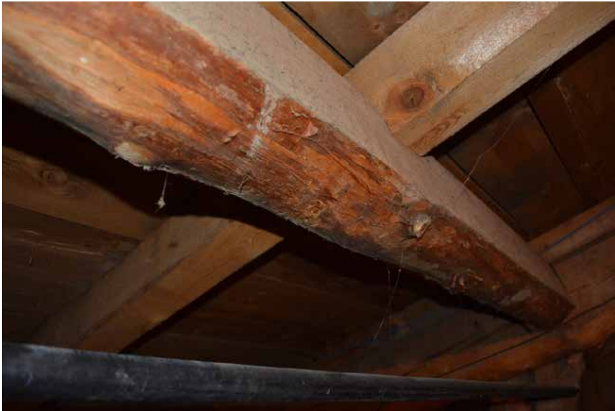
Photo 23: Looking South at purlin in east/west gable attic
