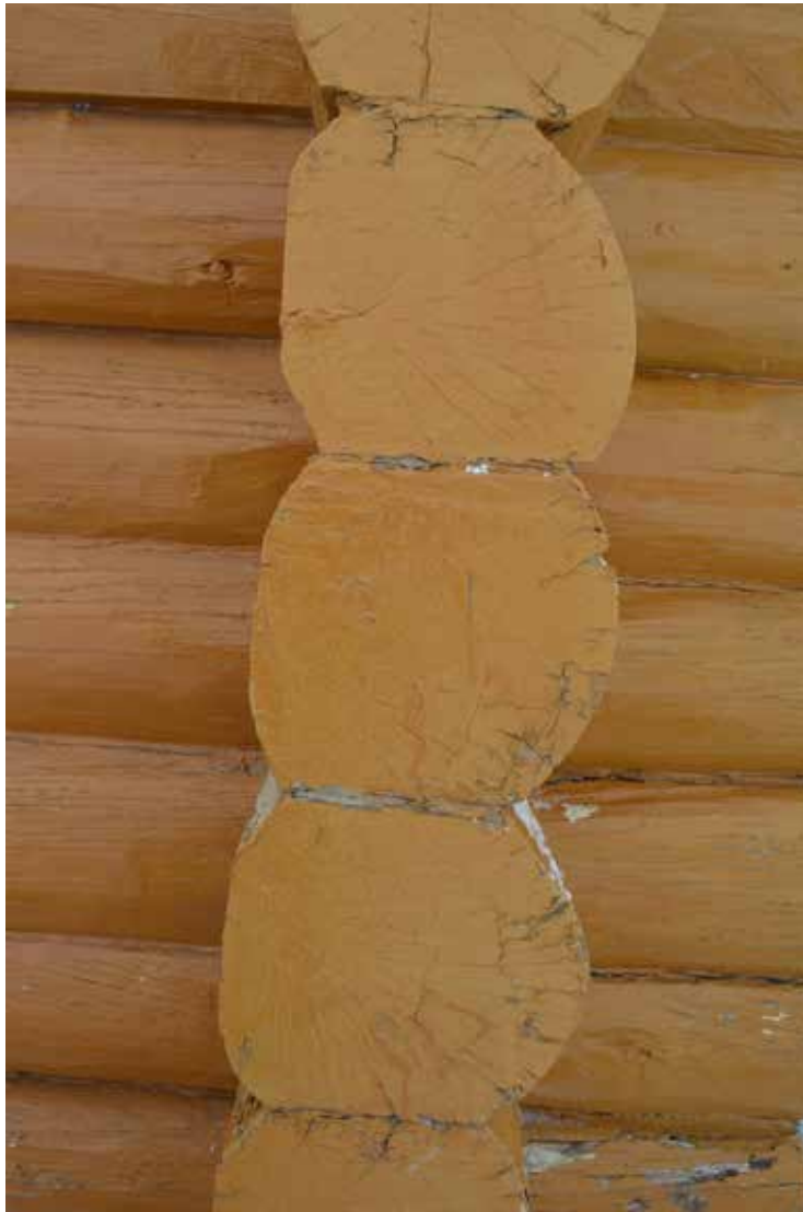
Photo 8: Close up of crown
