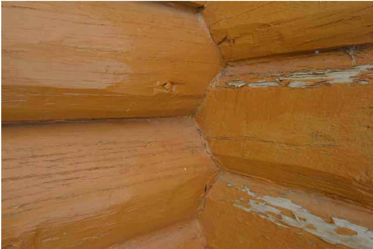
Photo 7: Closeup of joinery
