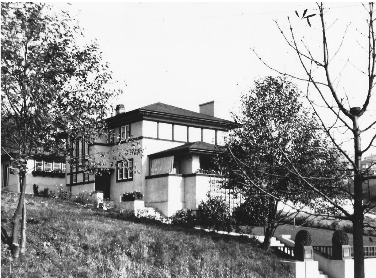
Matzen House exterior southwest corner of home. View to north.
