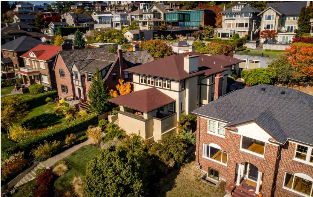
6 of 20. Rear (north) façade of Matzen House.
