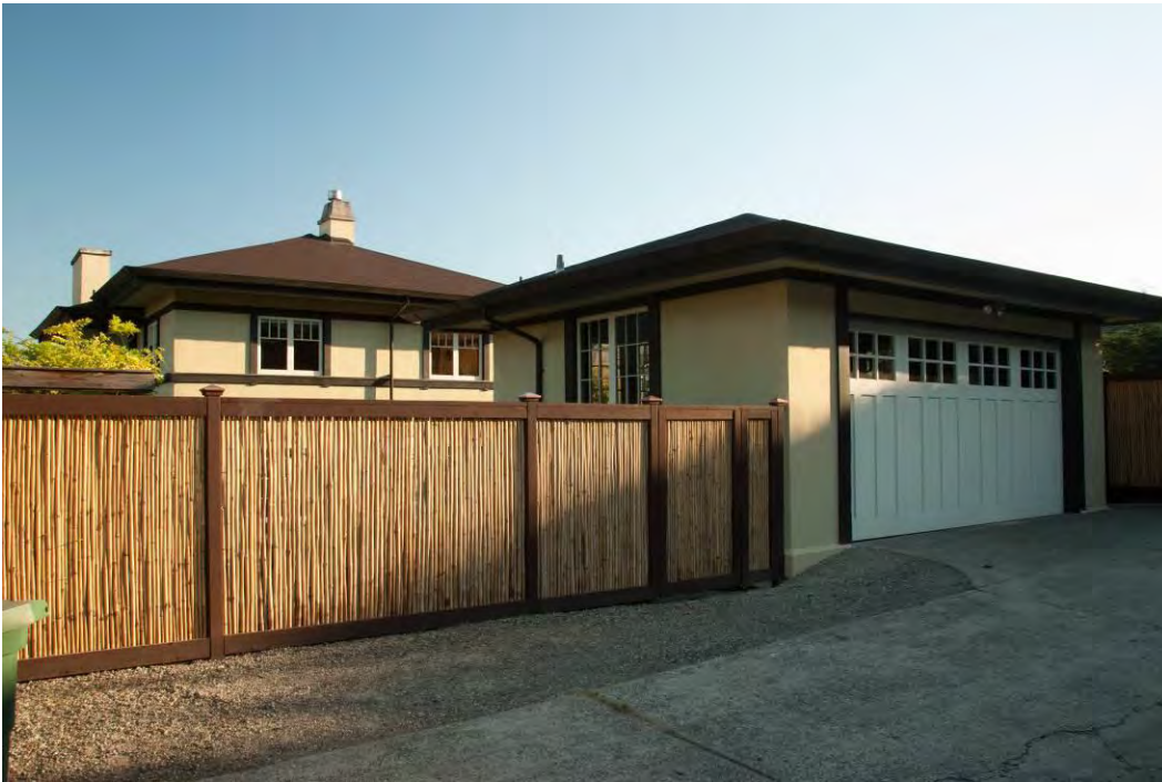
4 of 20. Rear (north) façade and garage of Matzen House.
