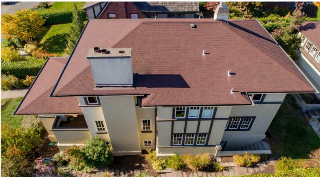
7 of 20. Rear (north) façade of Matzen House.
