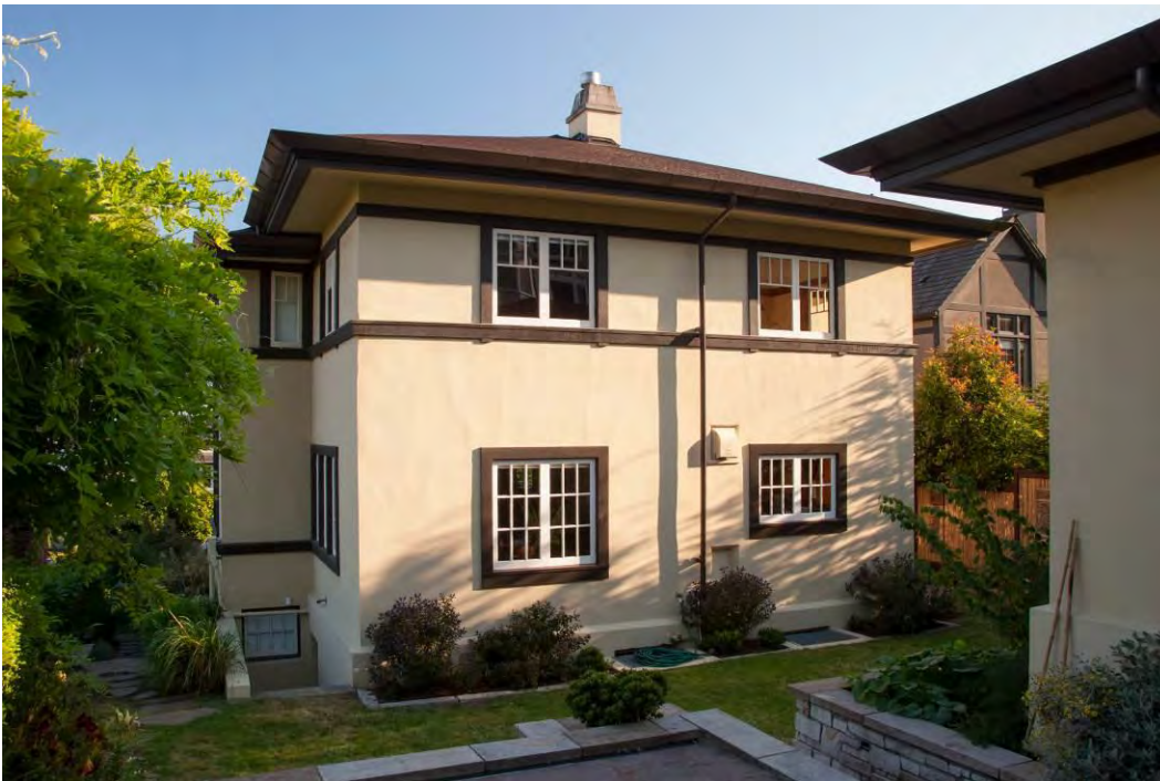
3 of 20. Rear (north) façade of Matzen House.
