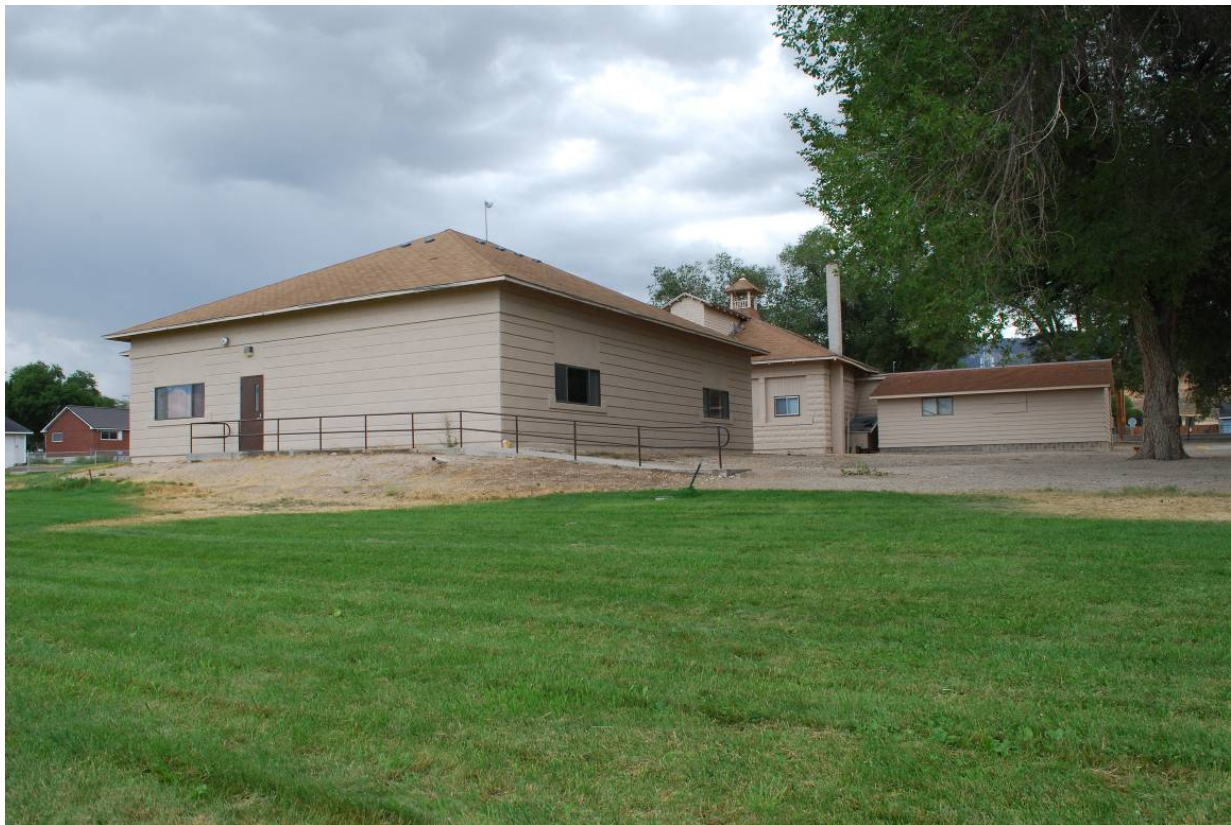
Photograph 7: West and south elevations of the classroom/lunch room addition, also showing the west elevation of the Kindergarten addition, looking northeast from the ball field (NVSHPO, 2017).
