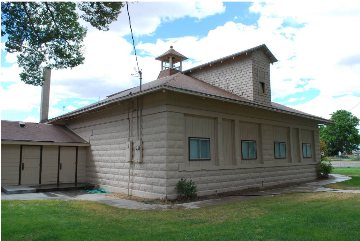
Photograph 2 - East elevation, looking northwest (NVSHPO, 2017).
