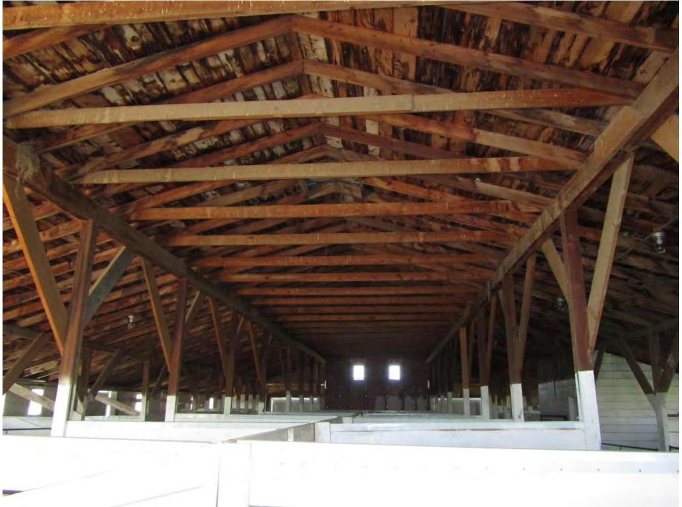
Photo 0008. Interior, Detail of Roof Structure, Facing: N
