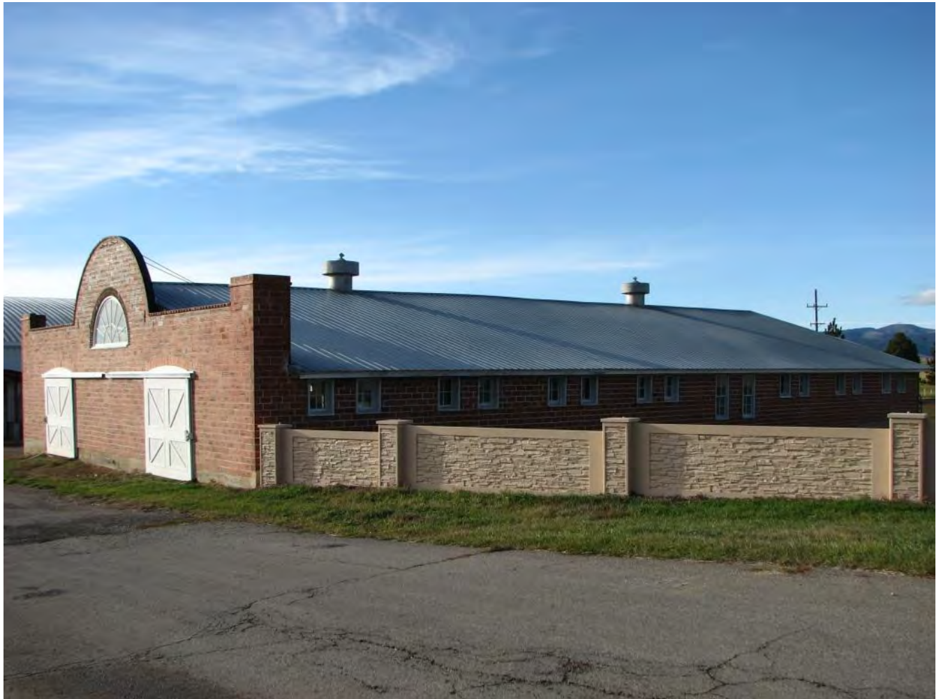
Photo 0004. South Façade and East Elevation, Facing: NW
