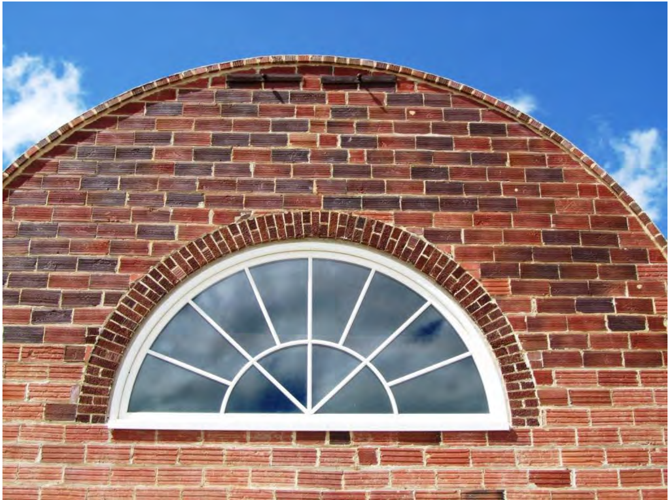
Photo 0005. South Façade, Detail of Fanlight, Facing: N
