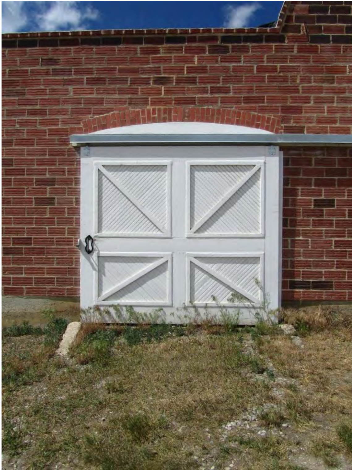
Photo 0006. South Façade, Detail of West Door, Facing: N
