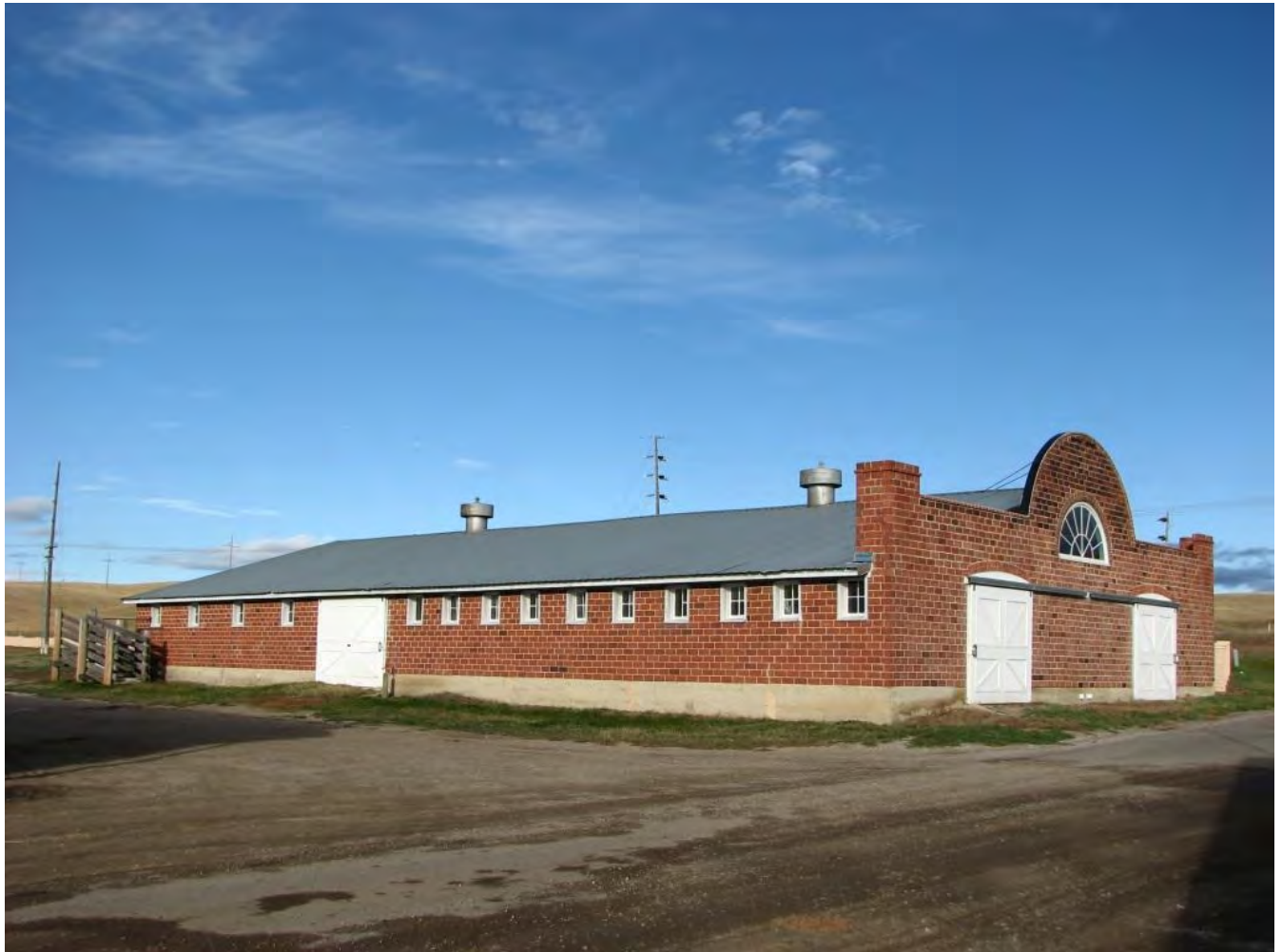
Photo 0002. South Façade and West Elevation, Facing: NE
