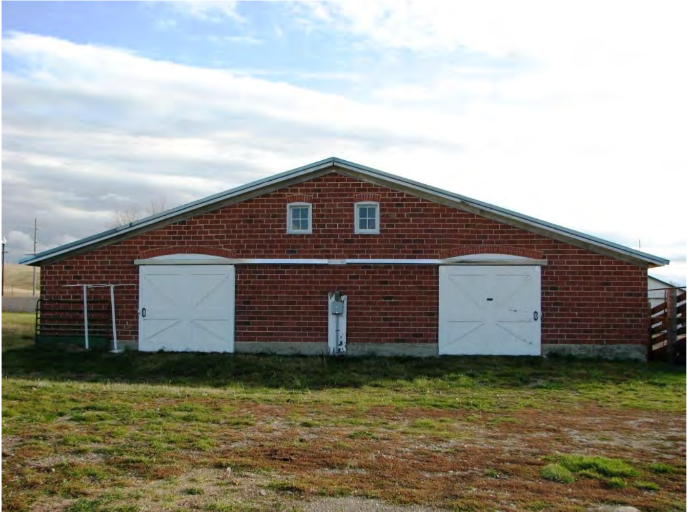
Photo 0003. Rear (North) Elevation, Facing: S
