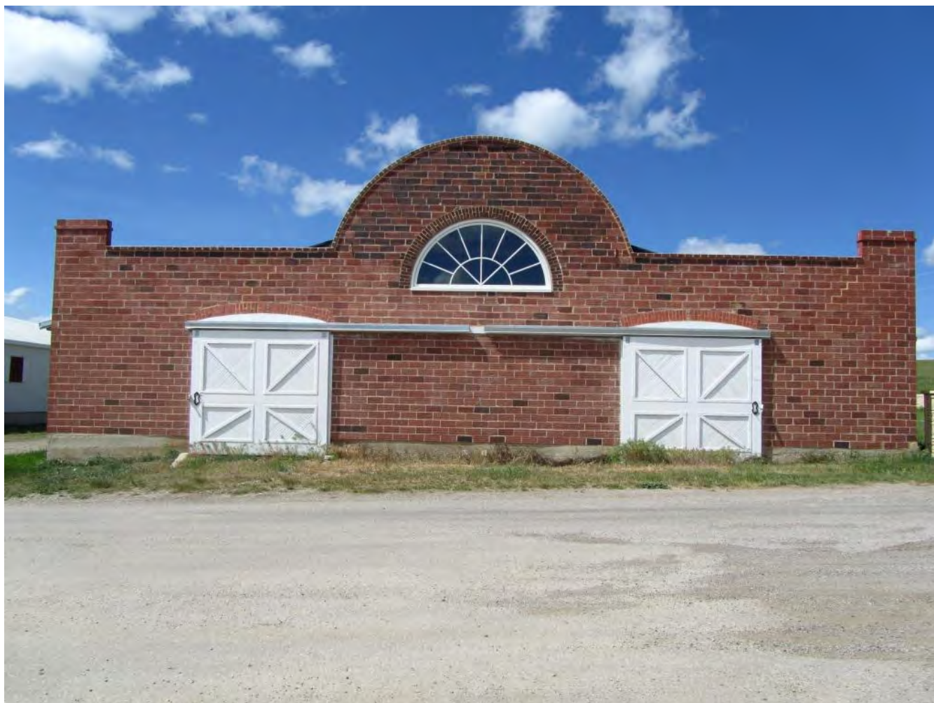
Photo 0001. South Façade, Facing: N
