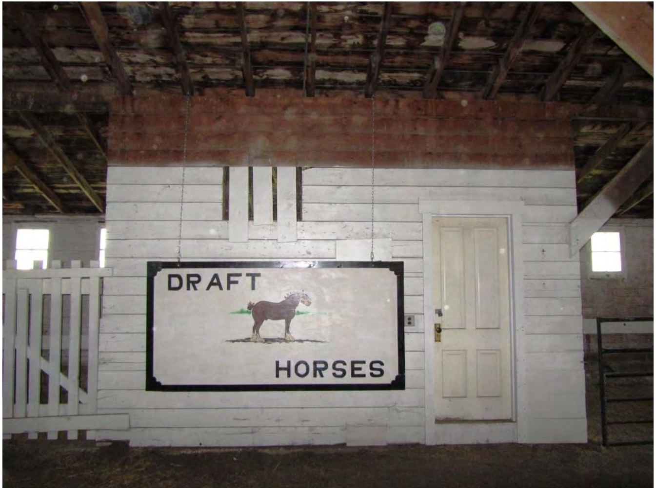
Photo 0009. Interior, Office at end of Cross Alley, Facing: E
