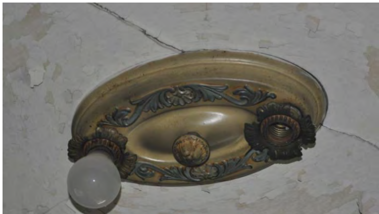
Image 4: Original light fixture and plaster ceiling. (Photo Perry, 2016)
