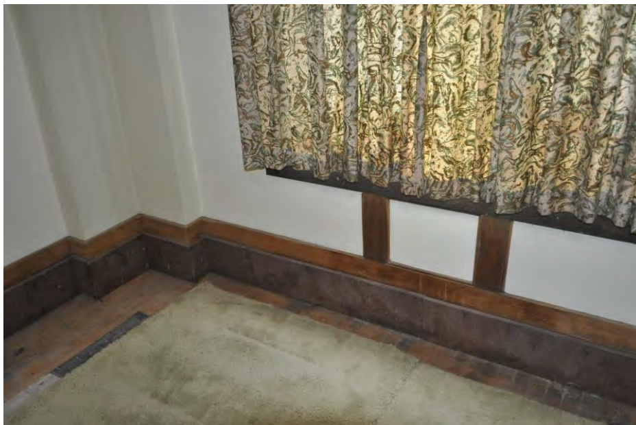
Image 7: Marble baseboards, capped with oak trim, decorate both the main lobby and the dining room. Note the decorative corner shape. (Photo Perry 2016)
