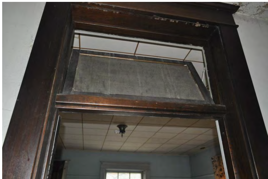
Image 2: Doors and transoms to the 50 guest rooms are intact, as is the wood trim. Some ceilings have tile covering. (Photo Perry, 2016)
