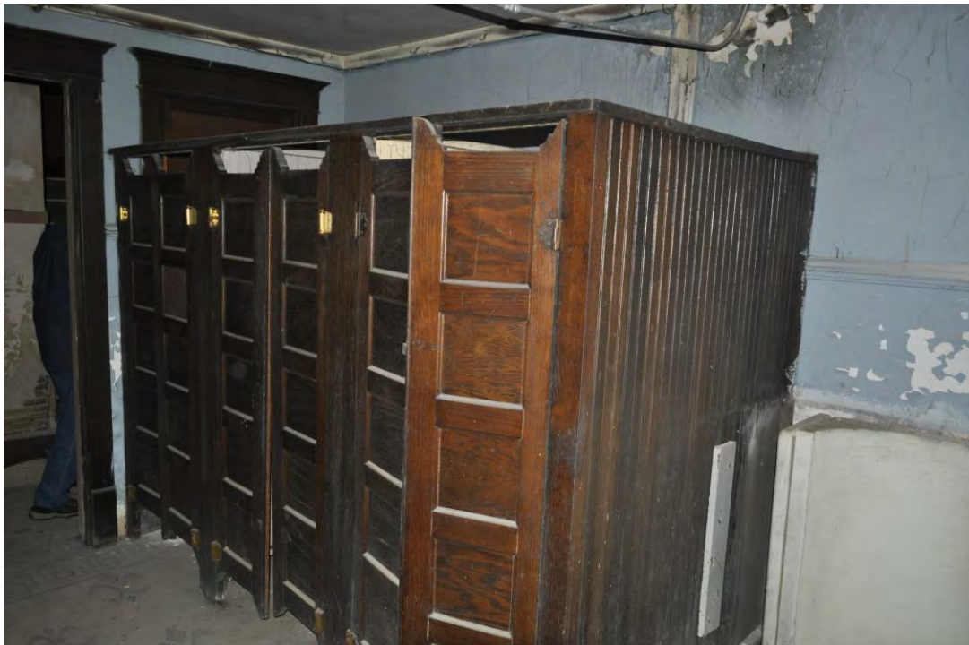
Image 9: Wood stalls in basement restroom. (Photo Perry 2016)
