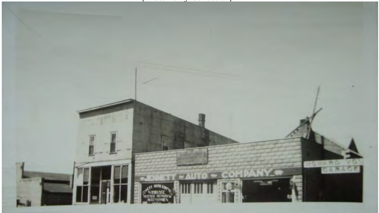
Image 15: Buildings immediately north of the Park Hotel. Concrete block construction was a common practice in the area. ca. 1920 (Block building extant, rest non-extant) (Photo Perry Collection)
