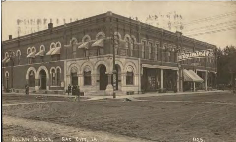
Image 12: The 1892 Allen Block on Sac City's Main Street housed a bank, city offices, and retail outlets on the main floor and a hospital to cure cocaine and alcohol addictions on the second floor. (buildings extant) (Name of building is misspelled on the post card.) (Photo Perry Collection)
