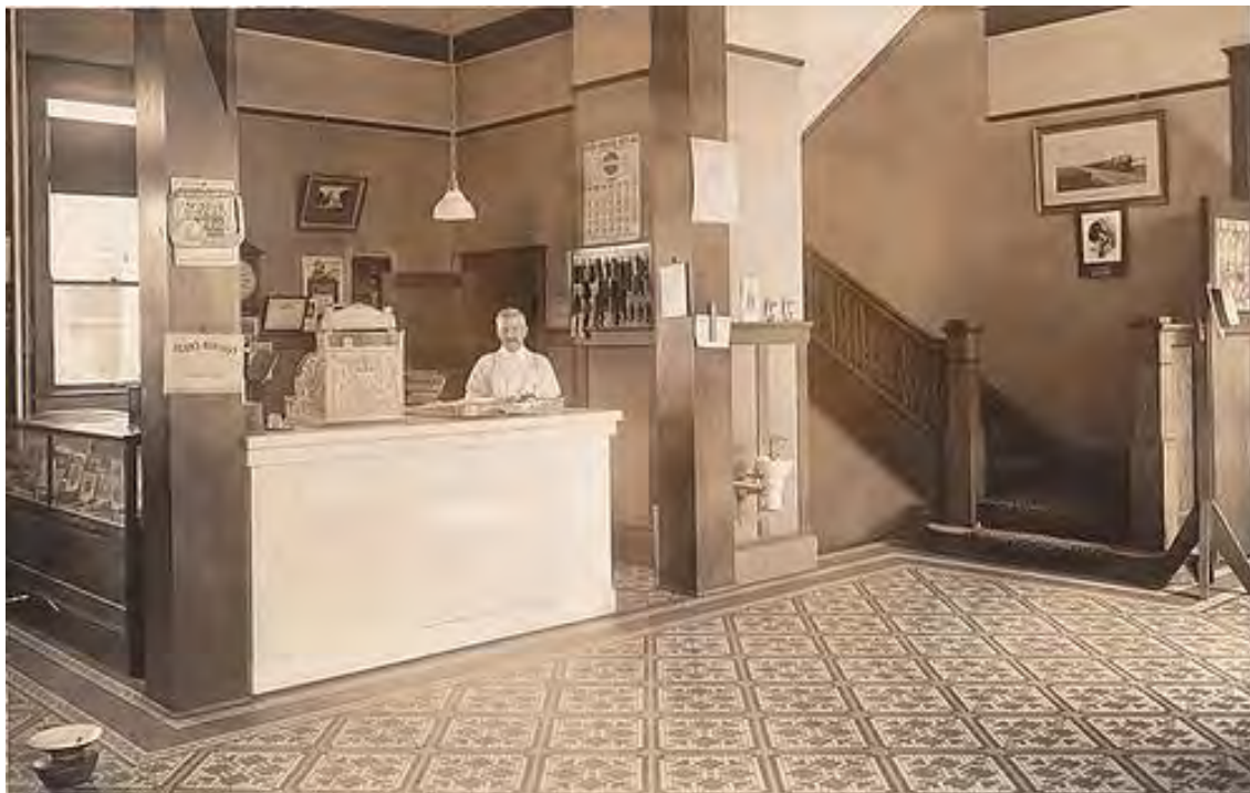
Image 34: 1915 view of Lobby of Park Hotel. White marble counter still sits in the lobby. The flooring is intact and in remarkable condition. Photo Perry Collection
