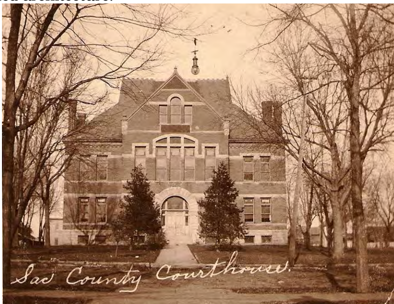
Image 11: 1907 view of Sac County Courthouse. The red brick and limestone construction was typical for buildings in the area. The dark area on the roof indicates where the cupola had been. (extant) (Photo Perry Collection)
