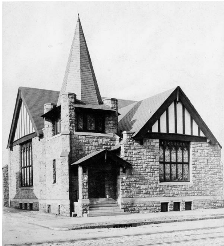
Figure 12: 1910 North Side Unitarian Church, 416 North West Avenue, Pittsburgh
