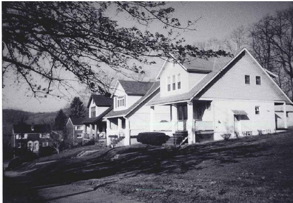
Figure 7: Craftsman/Bungalow homes along Delaware Avenue near its Intersection with 8 th Street (from PA SHPO files).
