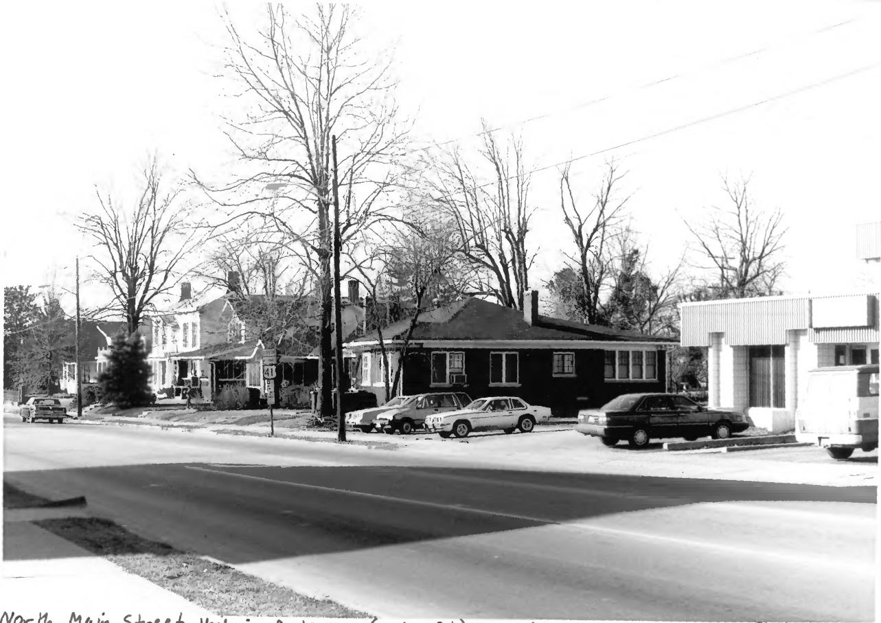
North Main Street Historic District (Madisonville)
