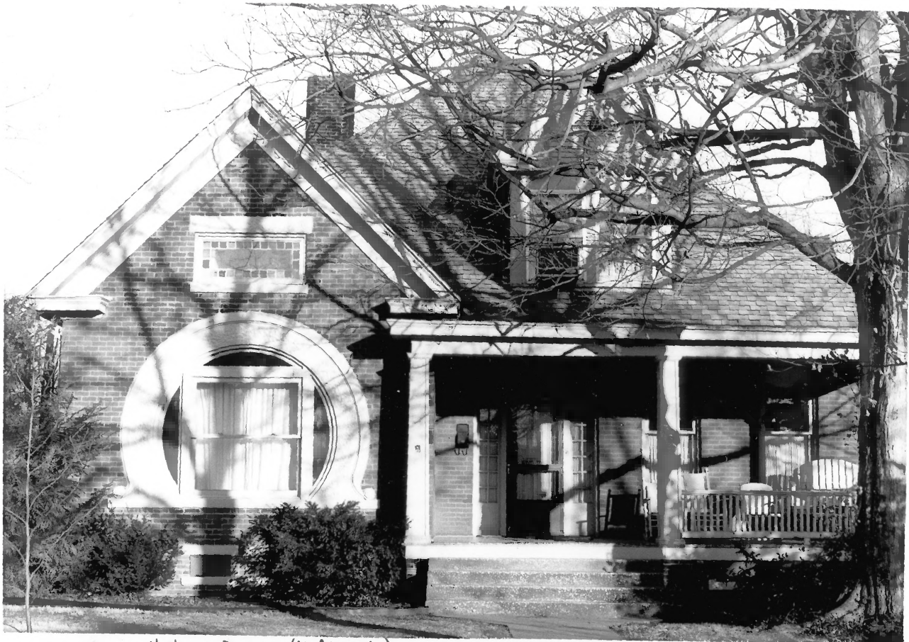
North Main Street Historic District (Madisonville)
