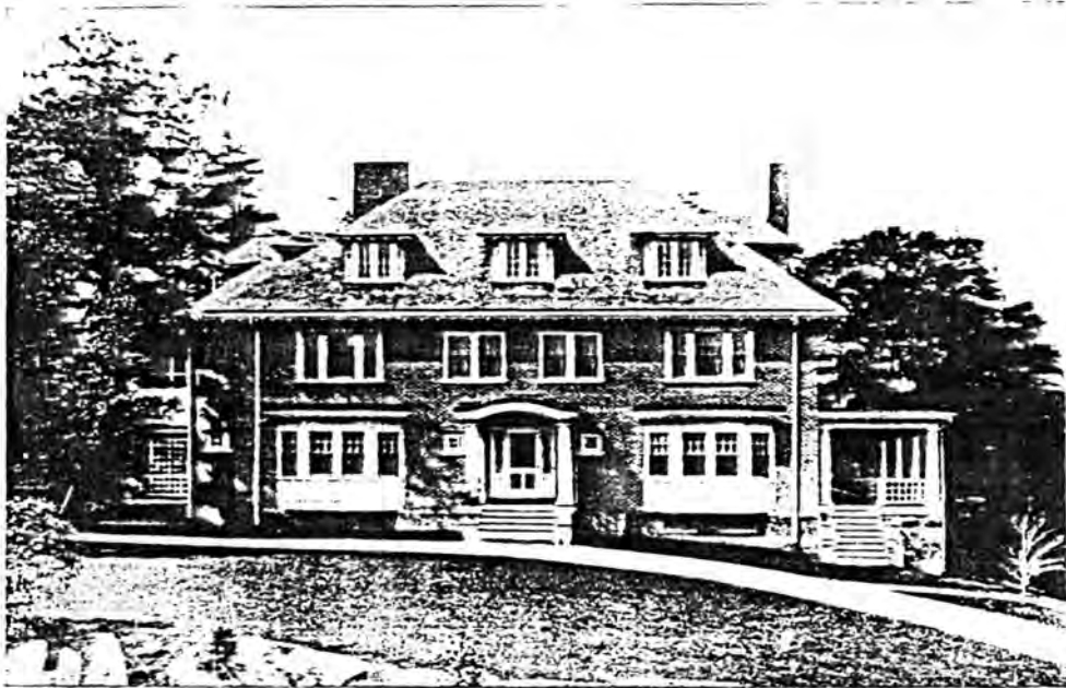
RESIDENCE OF FREDERIC F. CUTLER, HOBART ROAD, NEWTON CENTRE.
