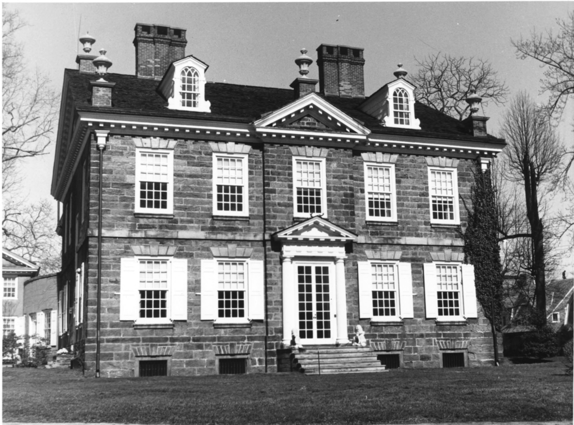
Cliveden, 6401 Germantown Avenue, Philadelphia, Pennsylvania
