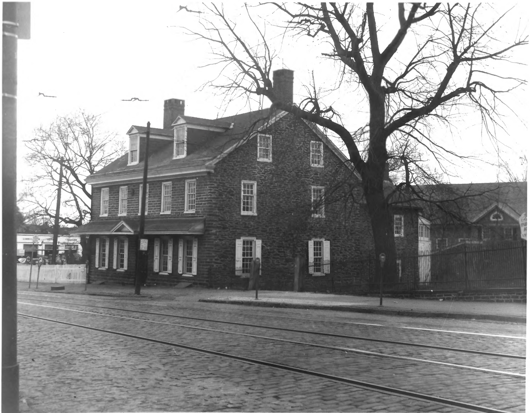
The Johnson House, 6306 Germantown Avenue, Philadelphia, Pennsylvania
