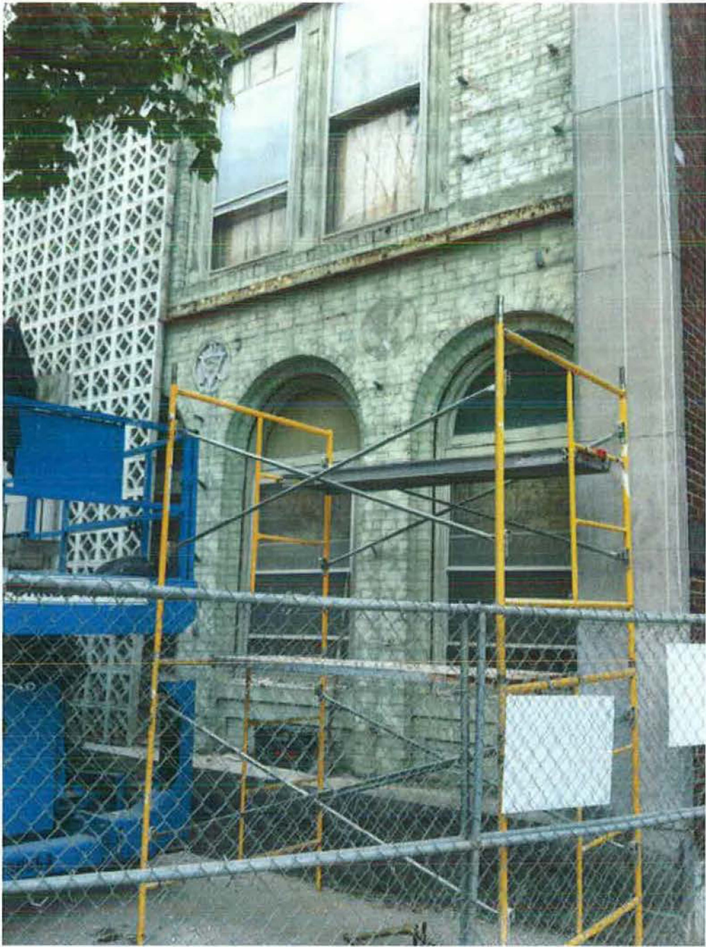
Photo 3. Detail of revealed 1913 façade of YMCA building.
