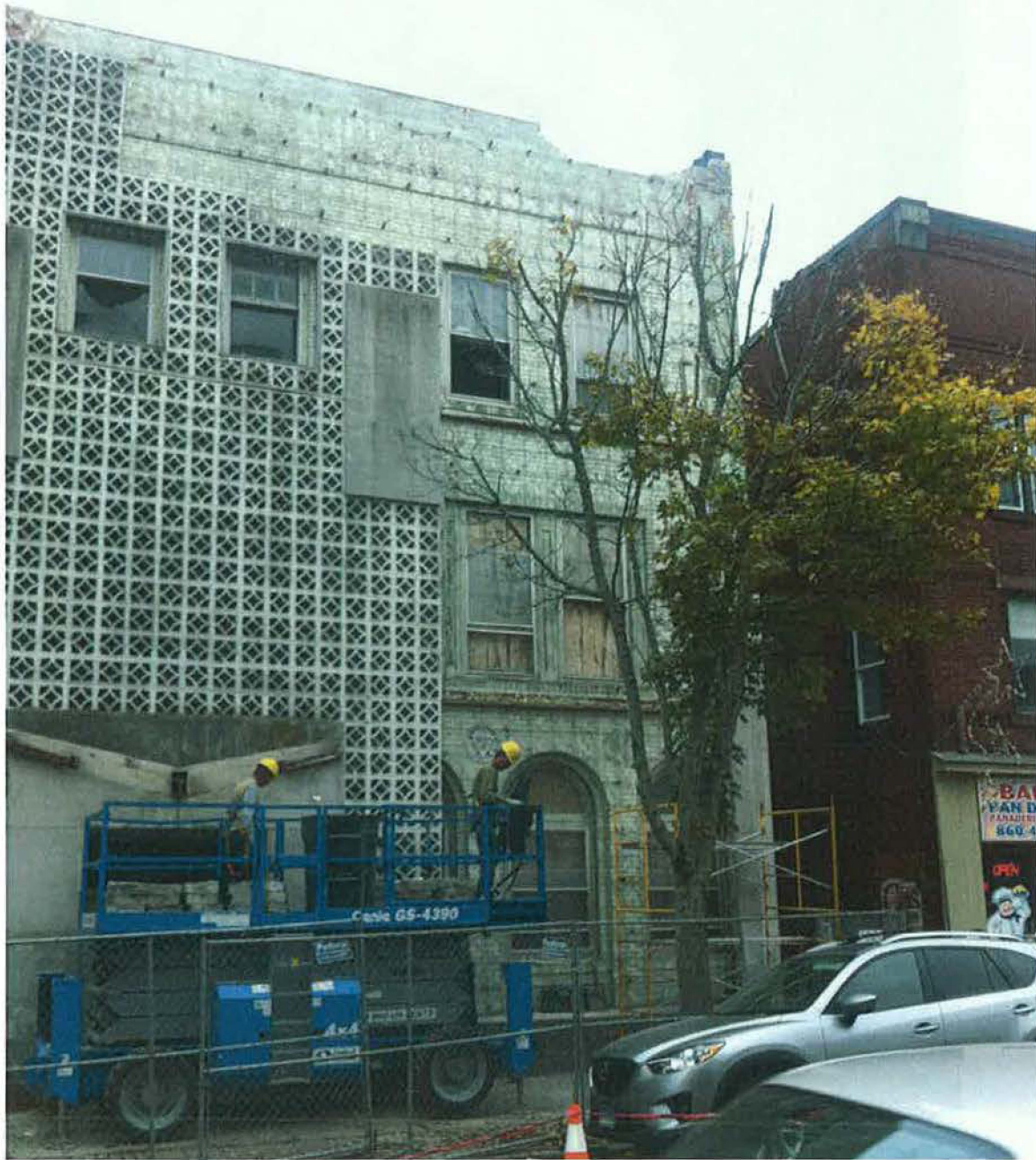
Photo 2. Workmen removing 1964 façade.
