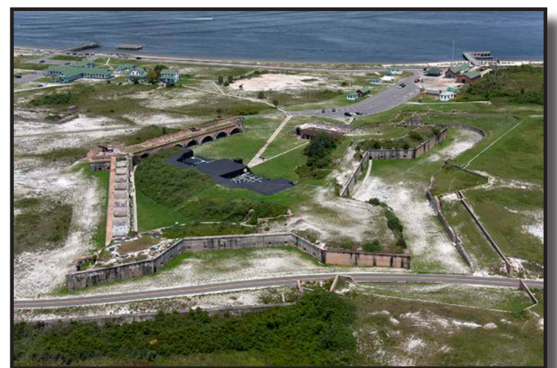
Aerial Image of Fort Pickens in Florida.
