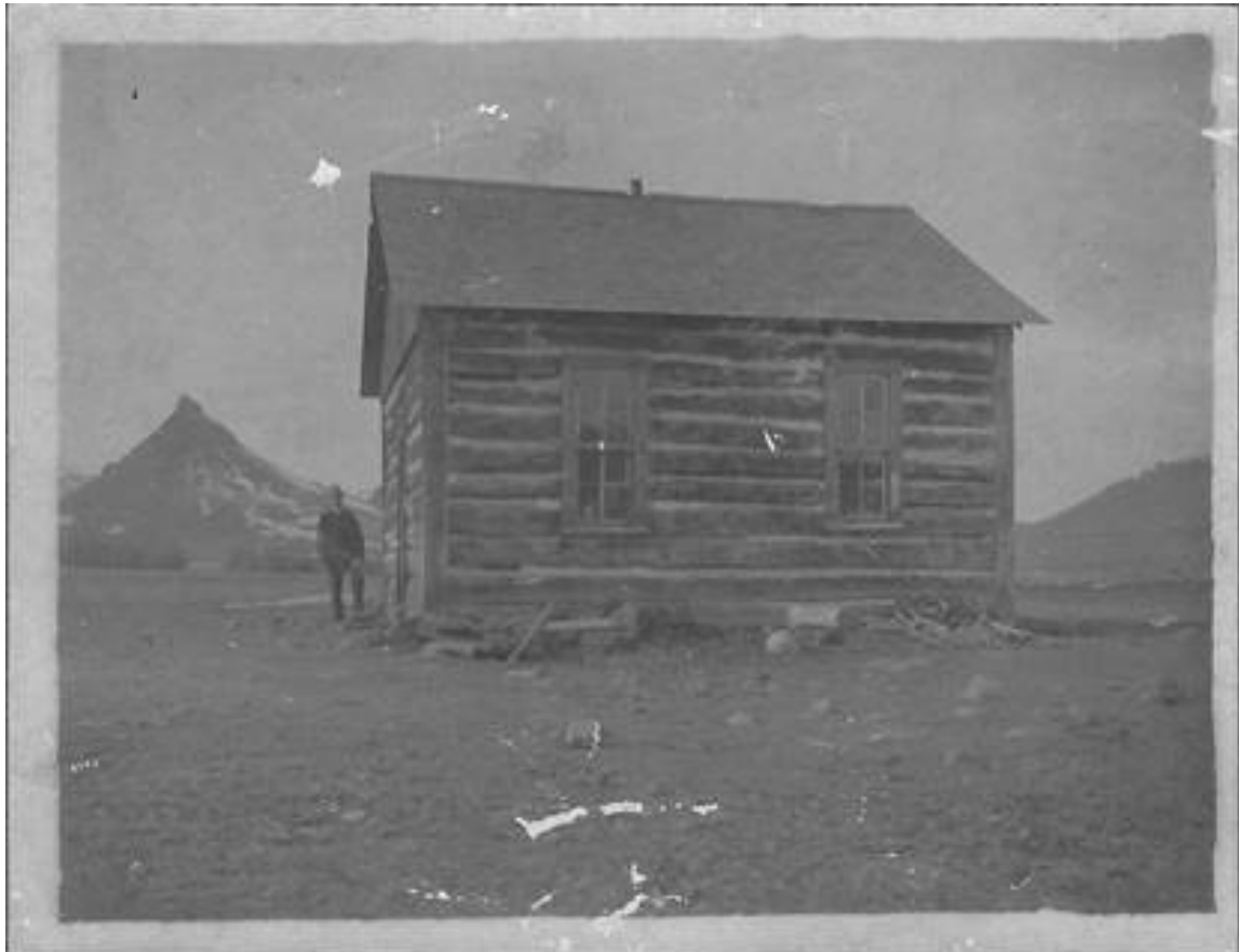
Original Dean School constructed from logs, 1904. Archive Collections, Museum of the Beartooths, Columbus, MT.
