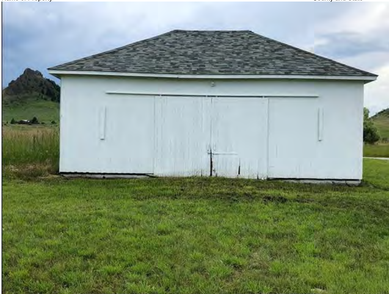
Description: Dean School Garage, East elevation, view to the west. MT_StillwaterCounty_DeanSchool_0008
