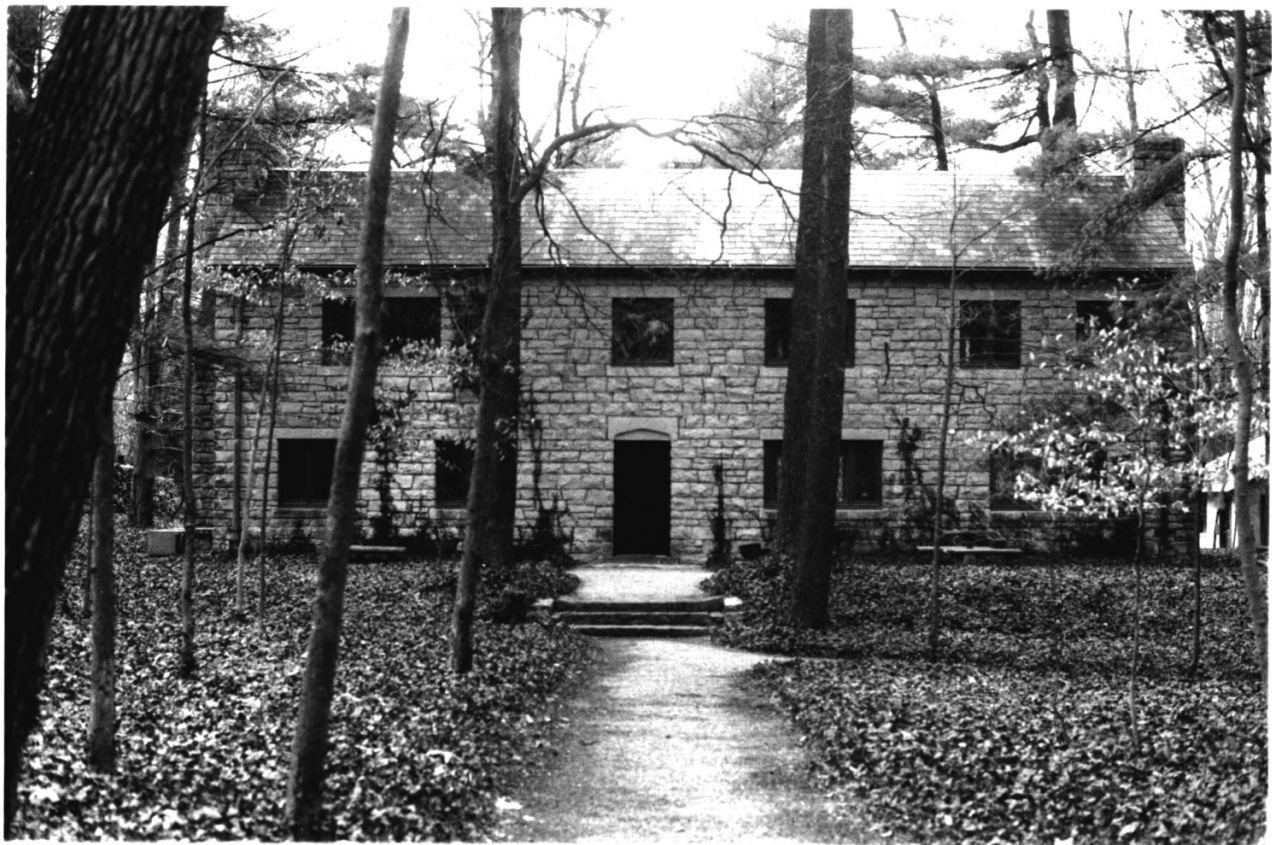
#7 Central Avenue Historic District - Fewee Valley, Oldham Co., Ky.
