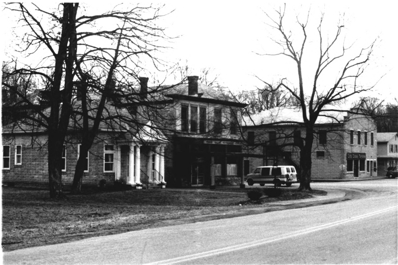
#2 Central Avenue Historic District - Fewee Valley, Oldham Co., Ky.
