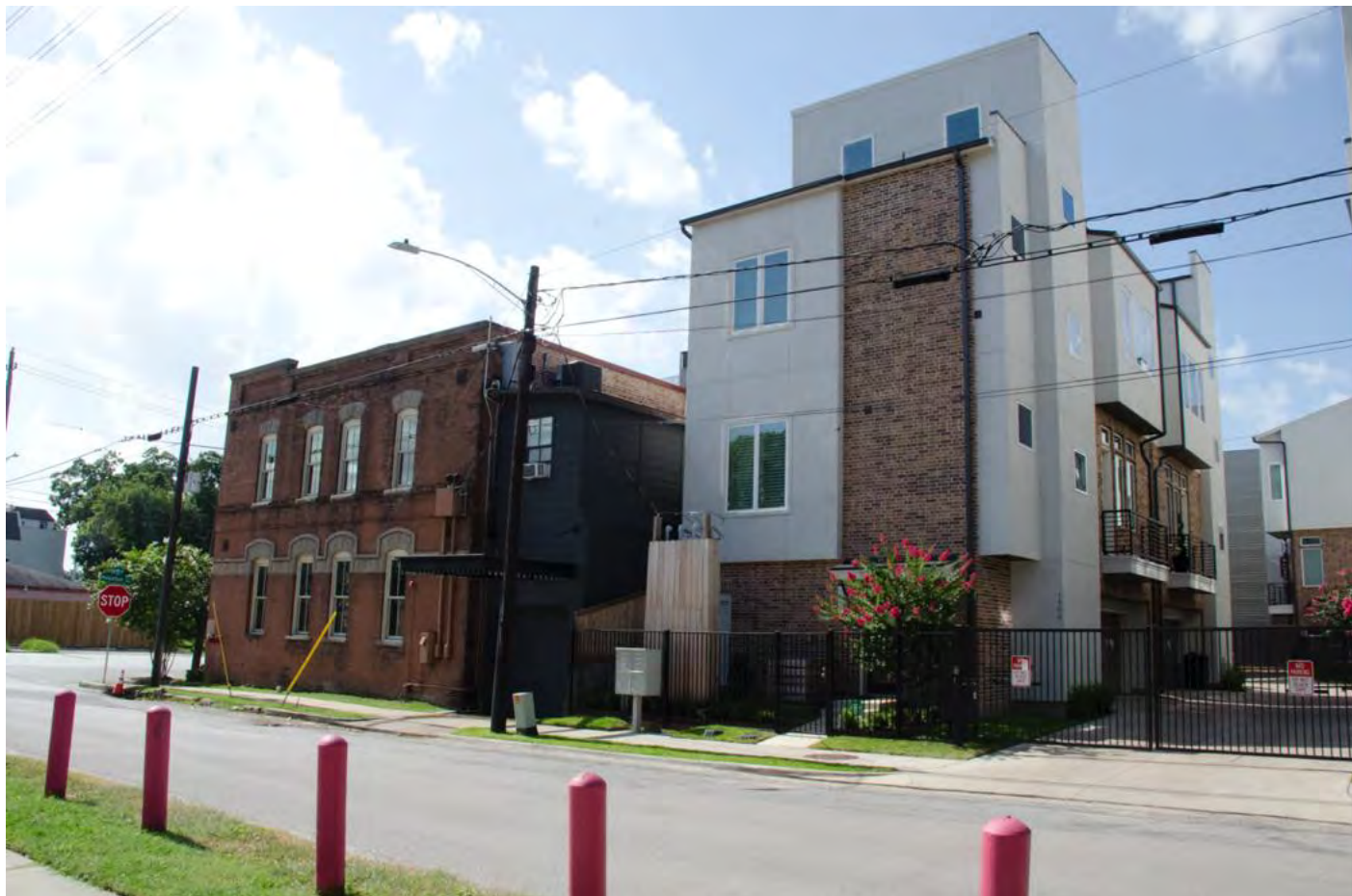
Photo 7: North & partial west elevation. Camera facing southeast.
