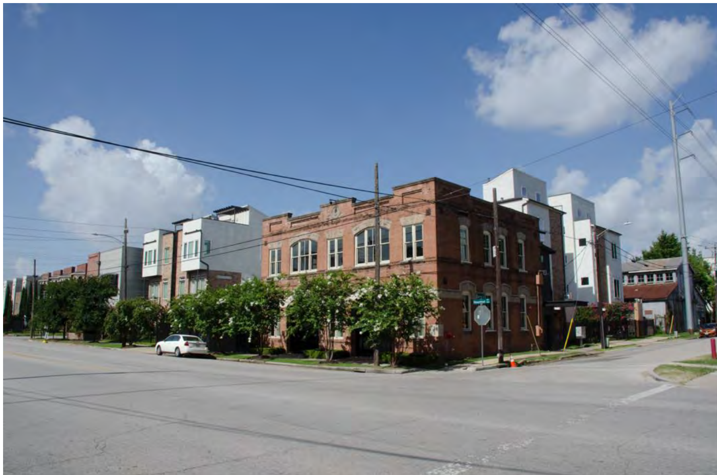
Photo 3: East & north elevations. Camera facing southwest.
