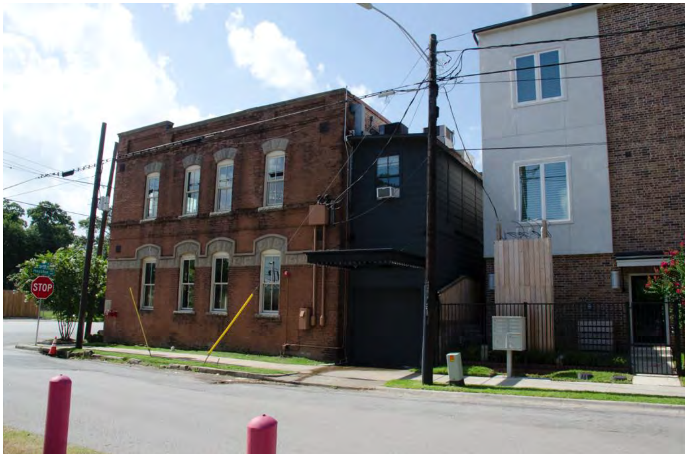
Photo 6: North & partial west elevation. Camera facing southeast.
