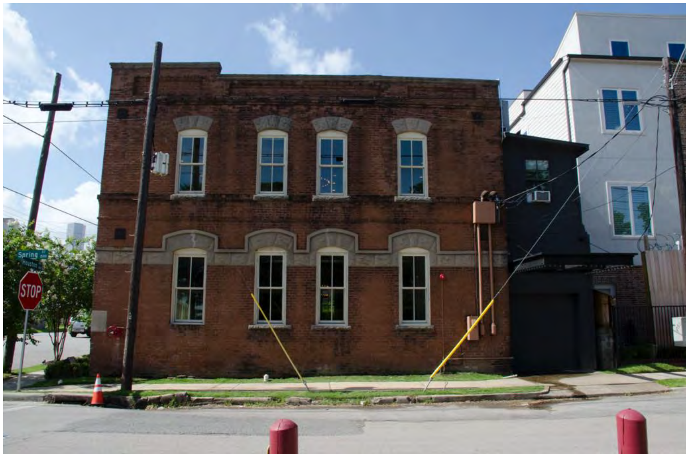
Photo 5: North elevation. Camera facing south.
