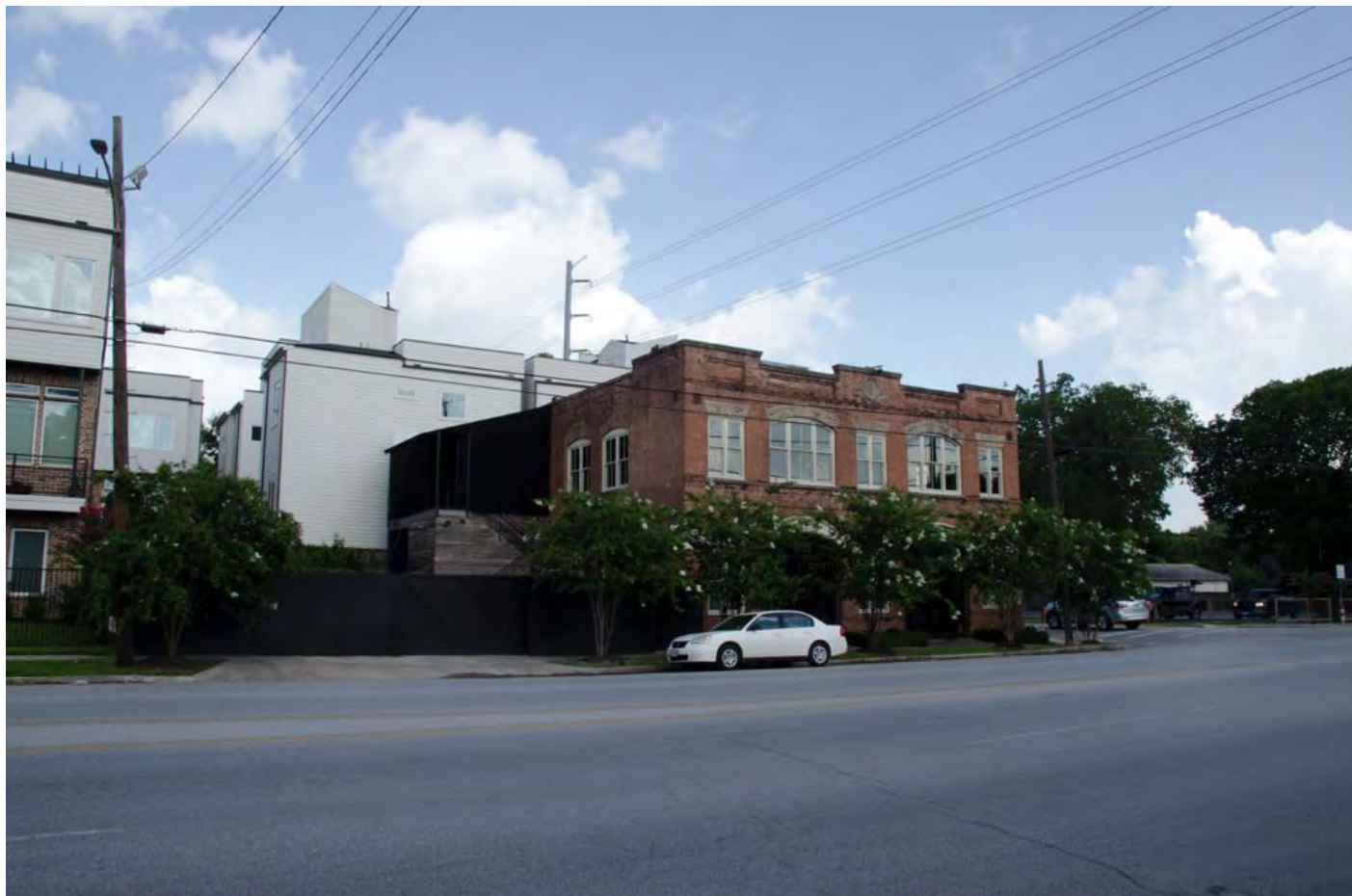
Photo 8: East & south elevations. Camera facing northwest.
