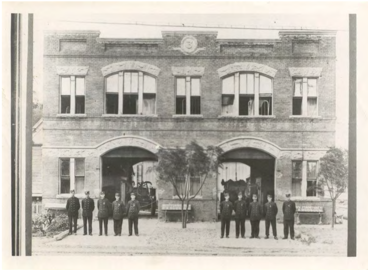
Figure 1: Historic Photograph of Fire Station No. 3, c. 1905. Source: Houston Metropolitan Research Center
