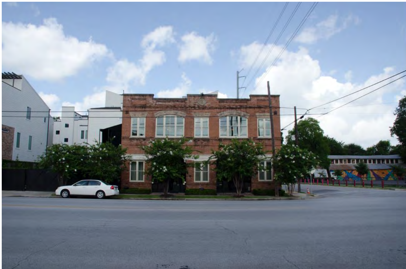
Photo 2: Primary (east) elevation. Camera facing west.
