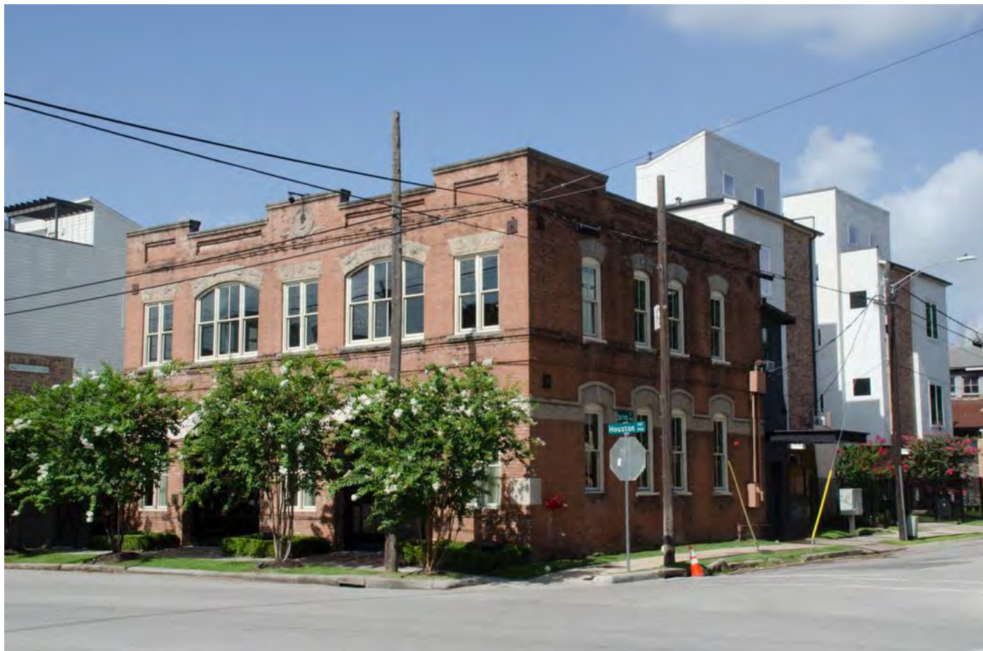
Photo 4: East & north elevations. Camera facing southwest.
