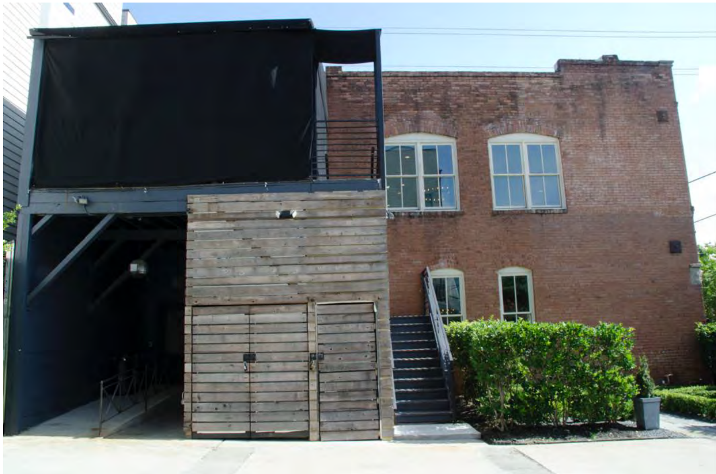
Photo 10: South elevation. Camera facing north.
