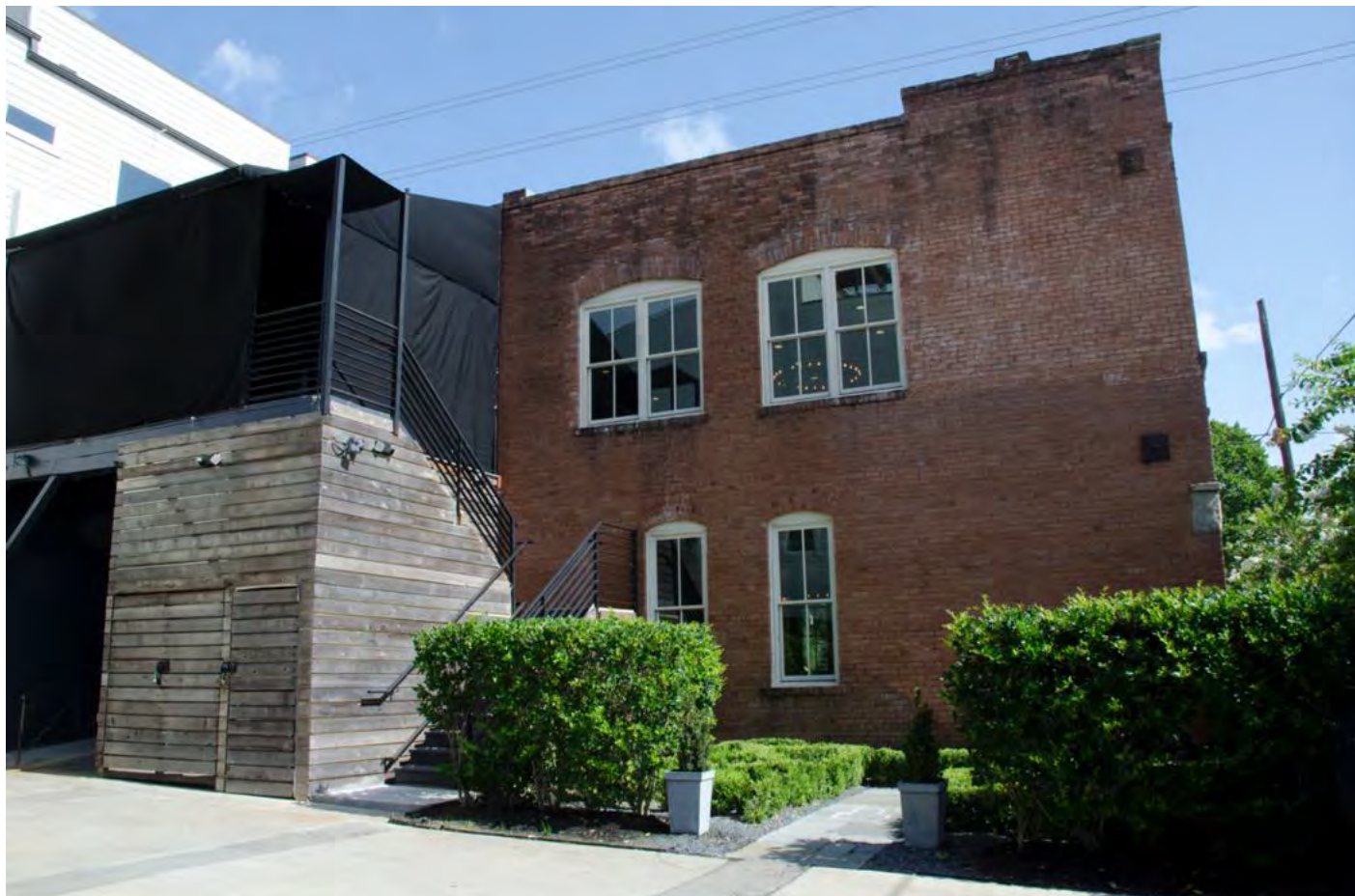
Photo 9: South elevation. Camera facing northwest.
