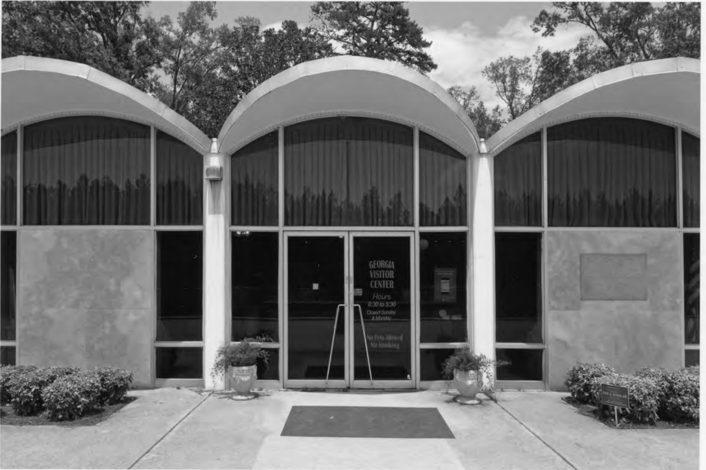
Georgia Welcome Center Screven County, Georgia Photograph 9 of 26
