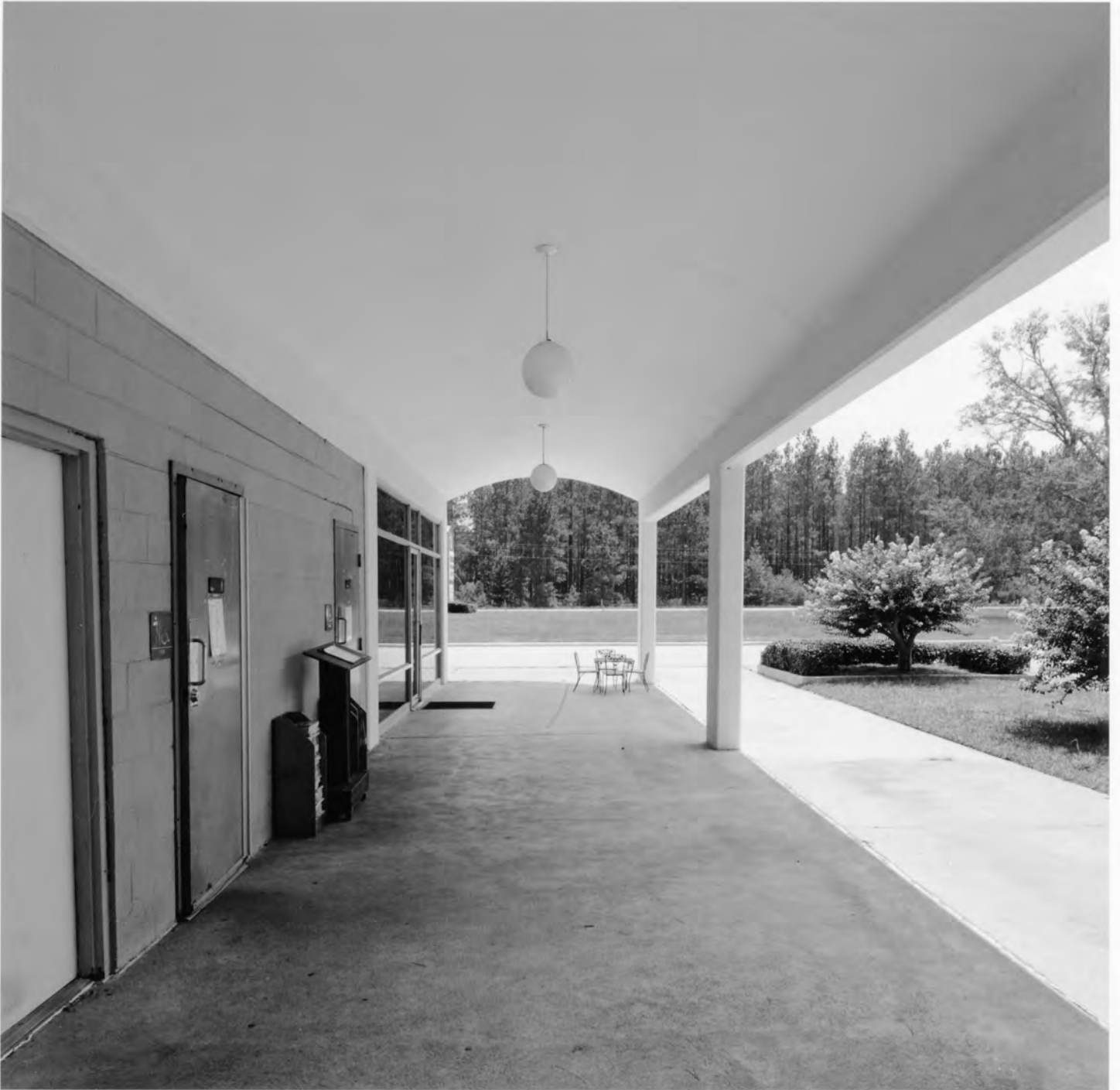
Georgia Welcome Center Screven County, Georgia Photograph 12 of 26
