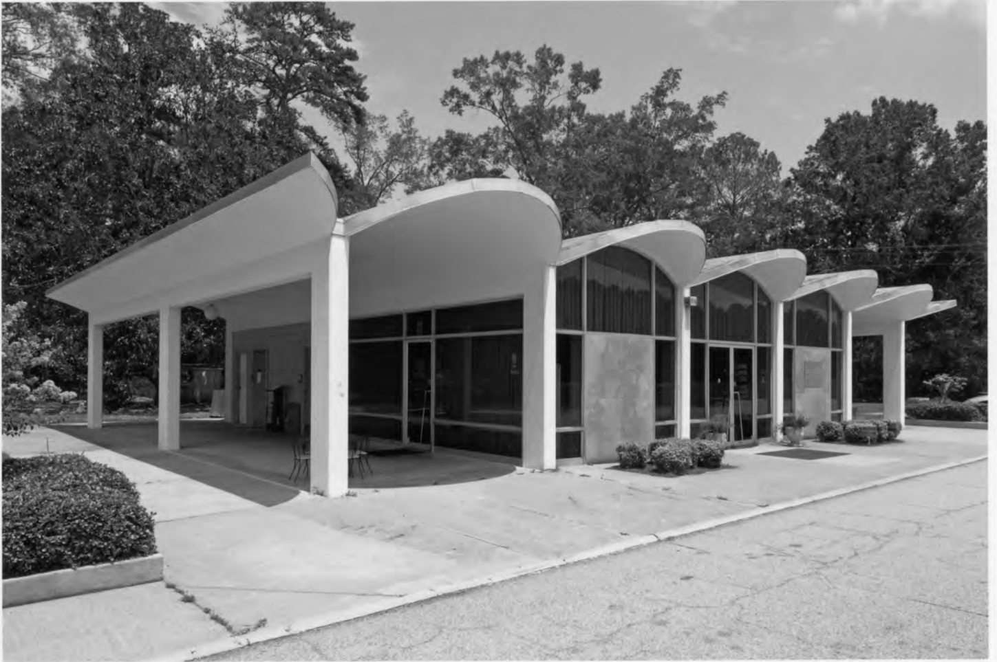
Georgia Welcome Center Screven County, Georgia Photograph 8 of 26
