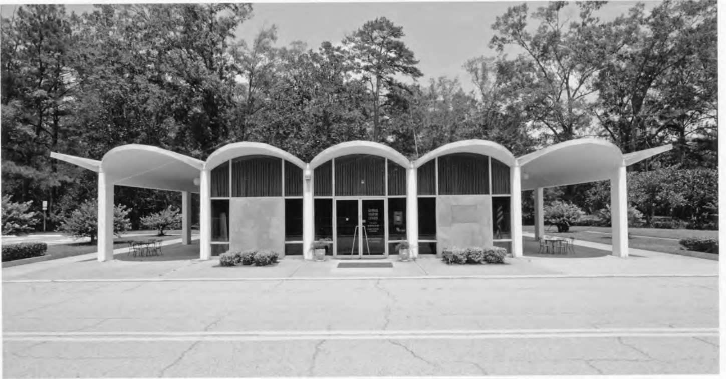
Georgia Welcome Center Screven County, Georgia Photograph 1 of 26
