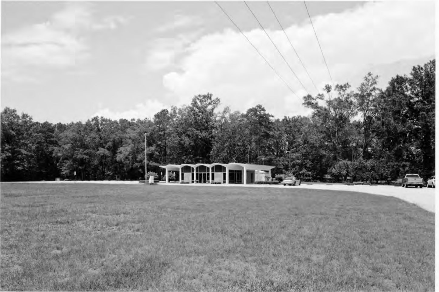
Georgia Welcome Center Screven County, Georgia Photograph 5 of 26
