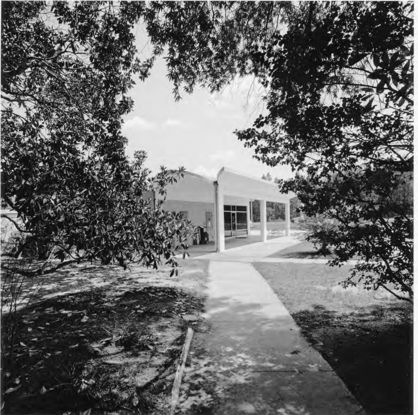
Georgia Welcome Center Screven County, Georgia Photograph 13 of 26
