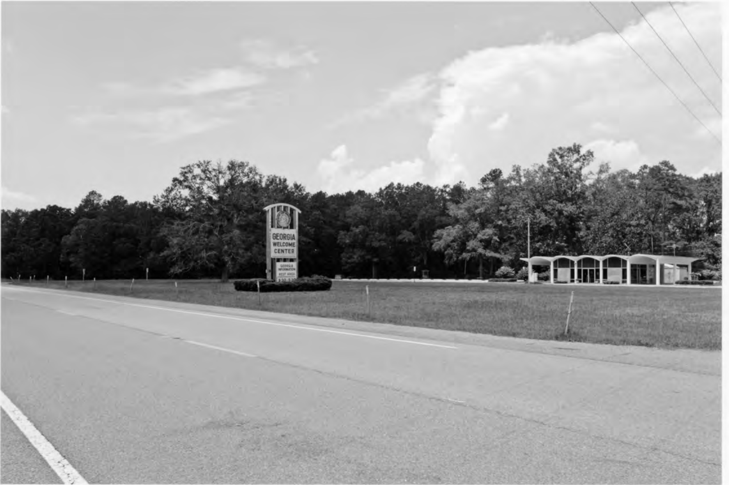
Georgia Welcome Center Screven County, Georgia Photograph 2 of 26
