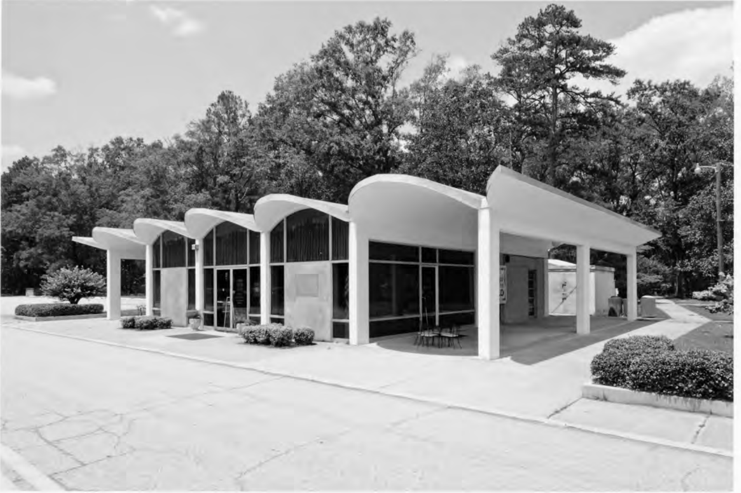
Georgia Welcome Center Screven County, Georgia Photograph 6 of 26
