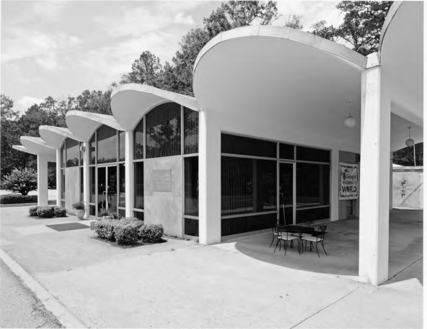
Georgia Welcome Center Screven County, Georgia Photograph 7 of 26
