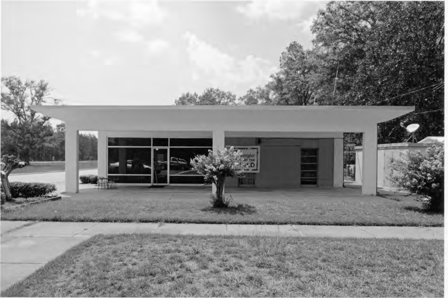
Georgia Welcome Center Screven County, Georgia Photograph 11 of 26
