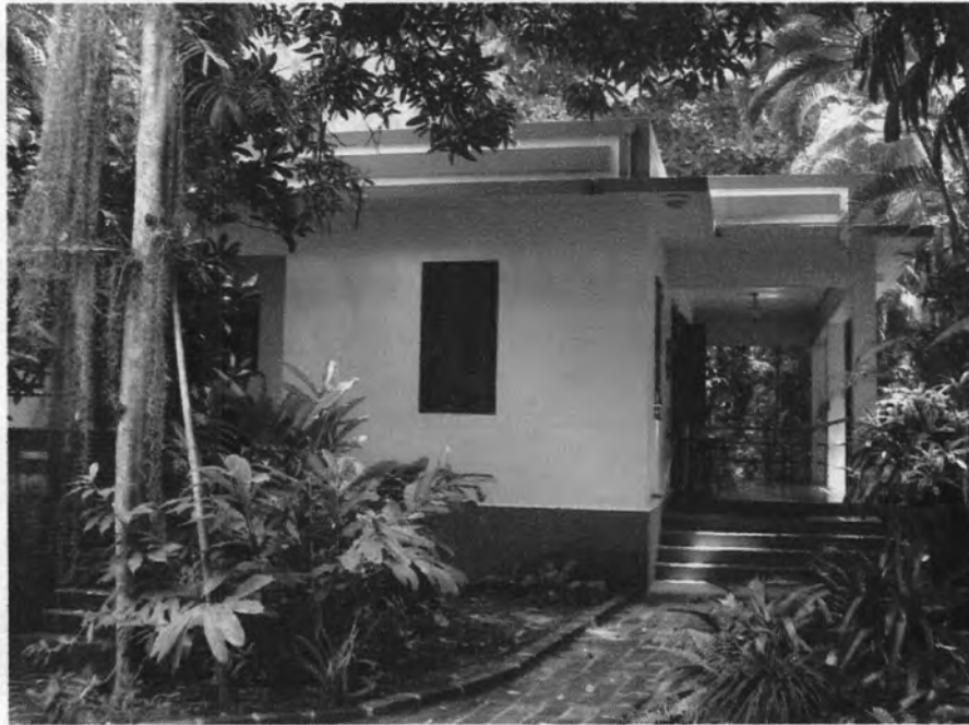
Figure 3 Façade view of main house, Photo María F. López, November 2010
