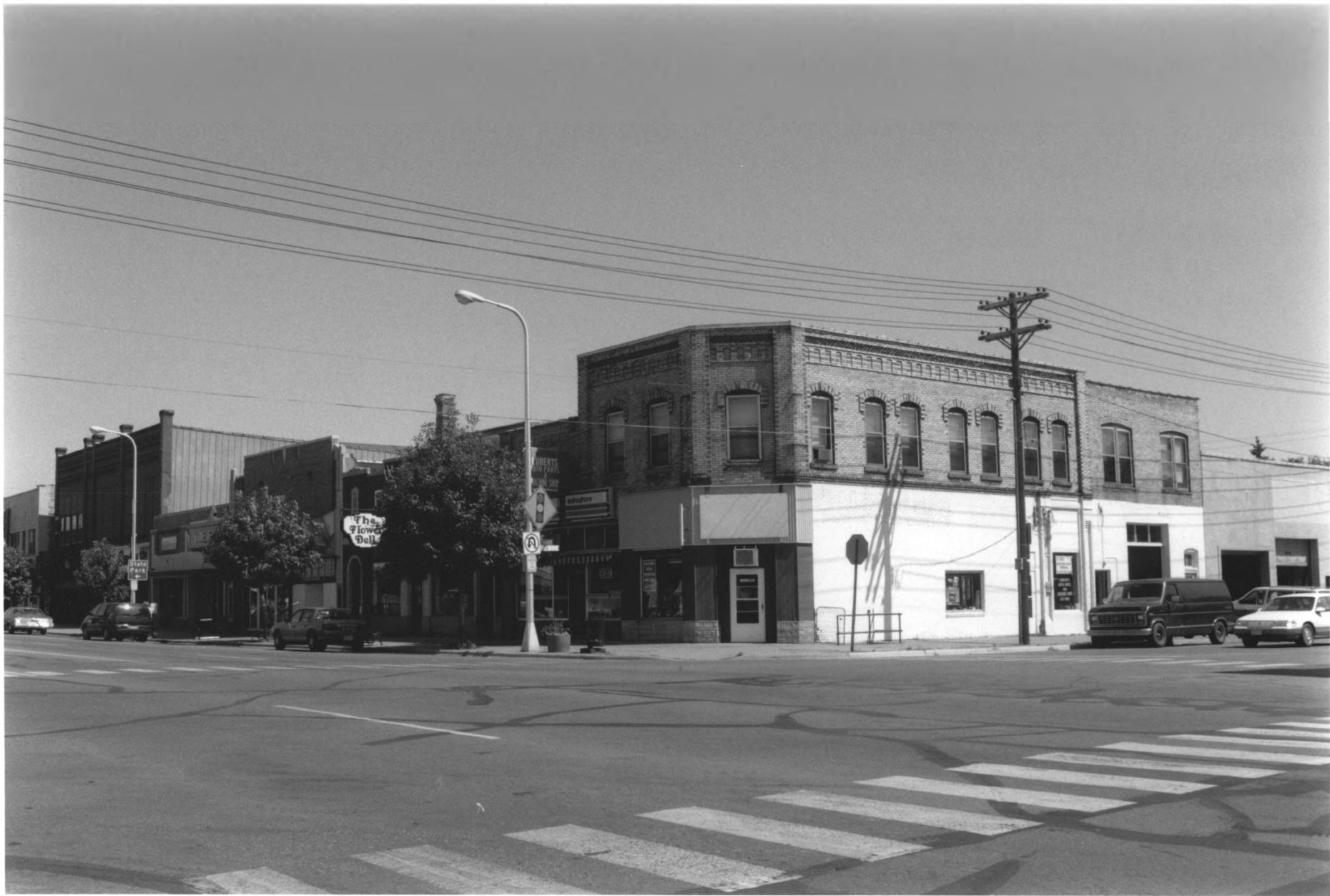
Streetscape: East side of 1st Street SE between First Ave. and Broadway - Little Falls Commercial Historic District Morrison Co. MN 011711 | 18
