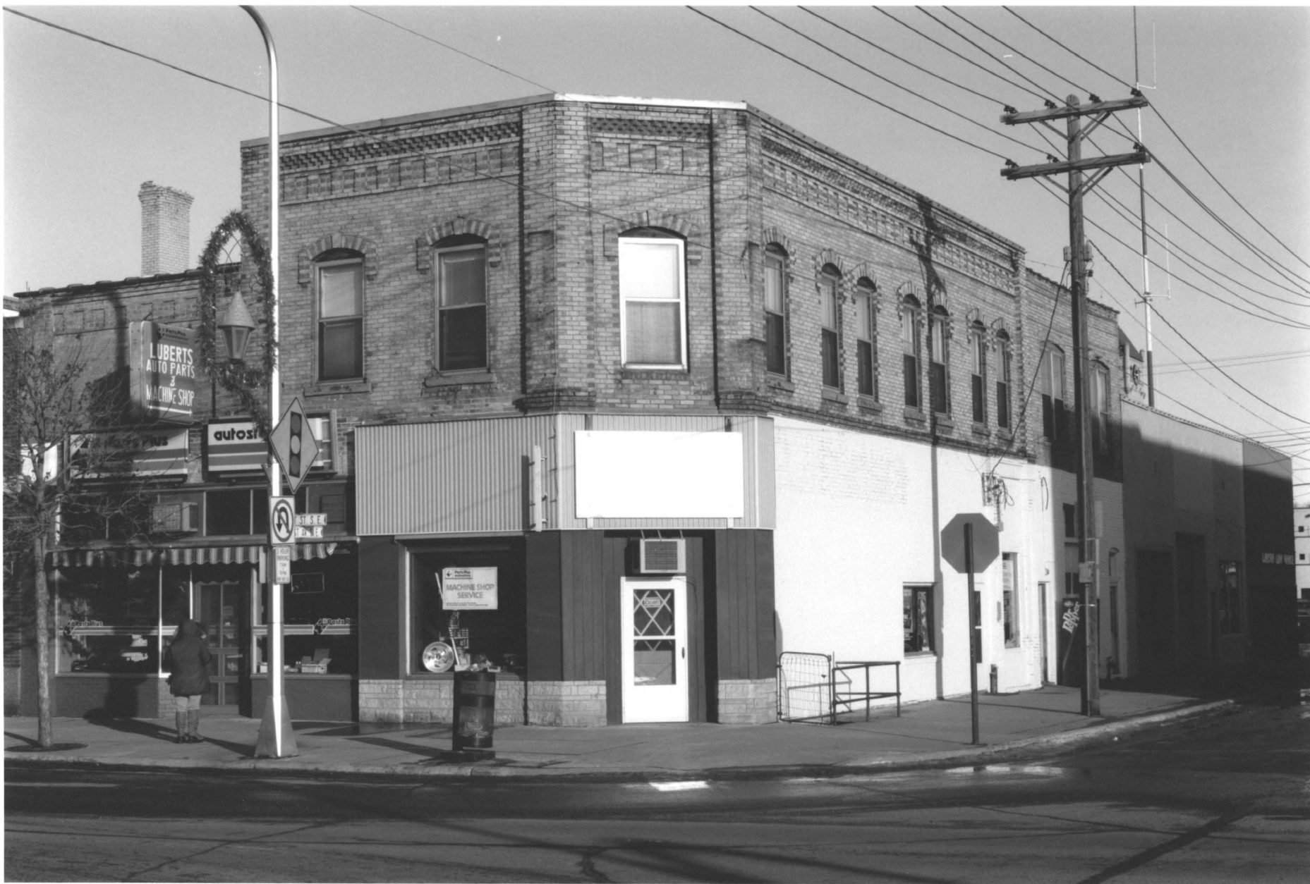
Hoffman Block #28 Little Falls Commercial Historic District Morrison CO. MN 011549 | 1A
