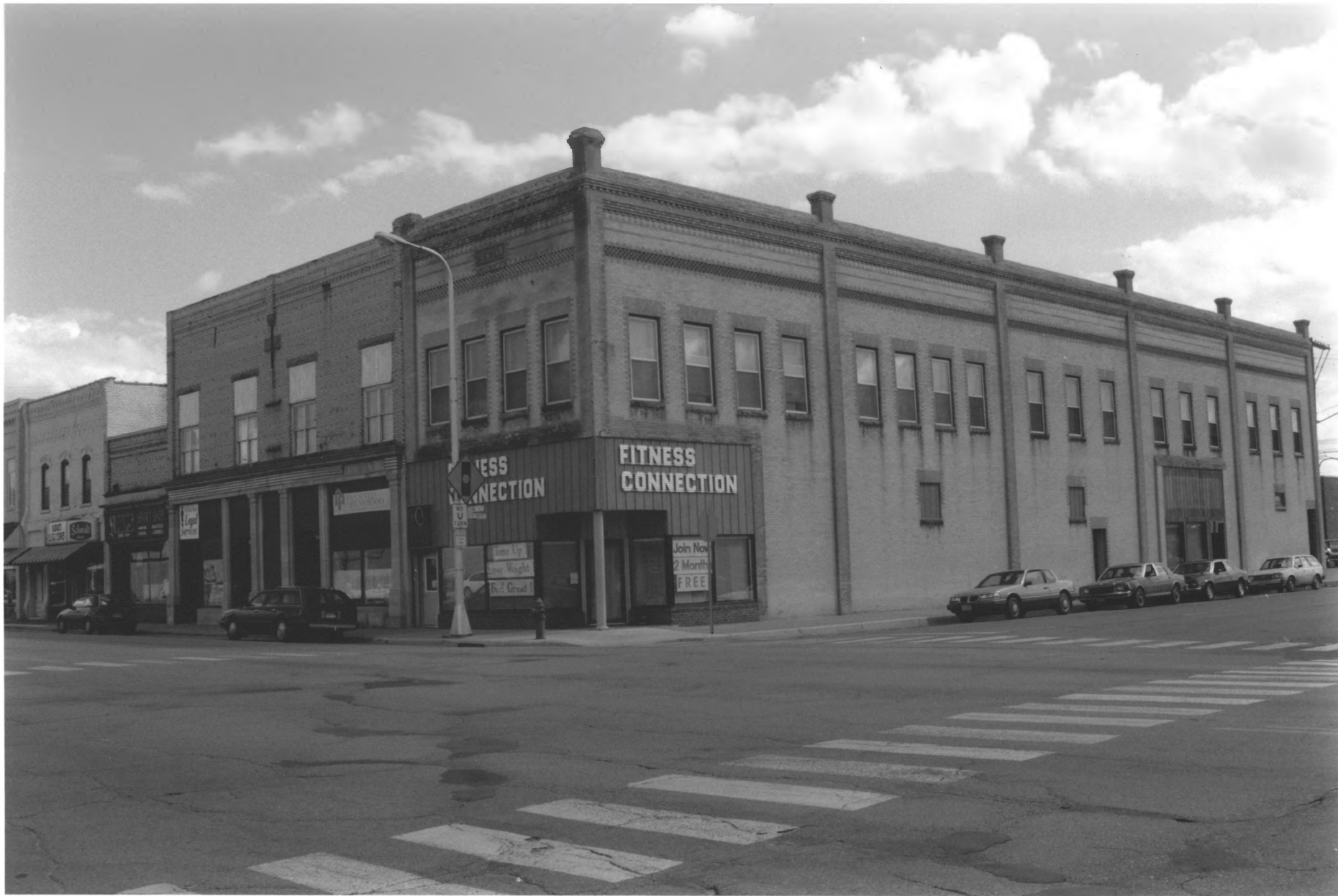
Left- Union Block Cardinal-wilcox Block #33 Right- Kiewel Building #32 Little Falls Commercial Historic District Morrison Co. MN 011710 | 5
