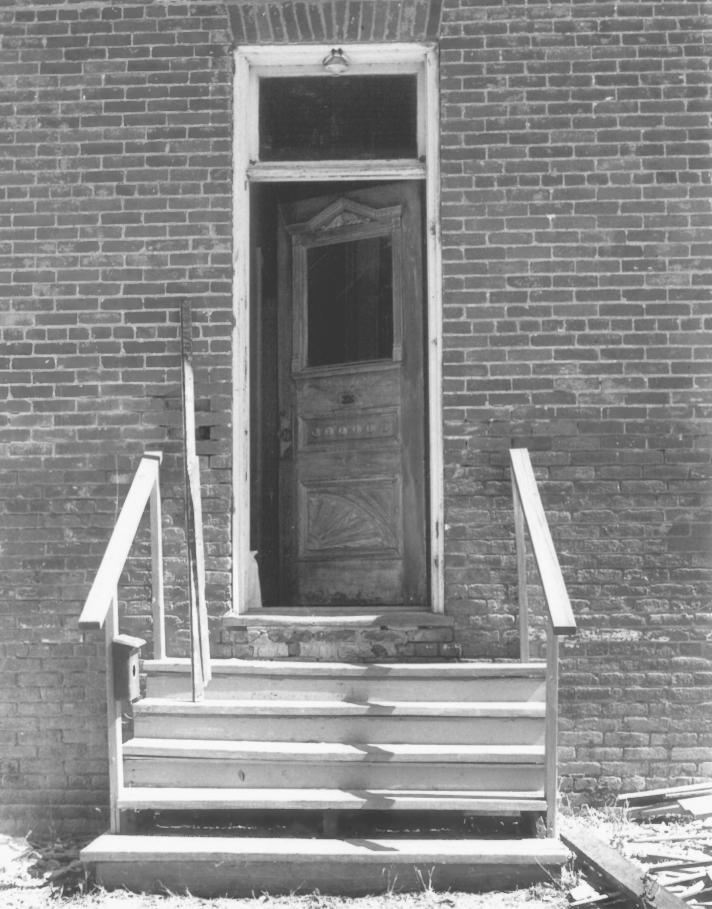
The Carr House Benicia, Ca. Photo by Nancy Olson, July 78 Hill's Library Forlorn view of the front door and stoop facing north. The electric wire to outside light probably holds door and door-frame in place. Bricks by rail have no mortar.
