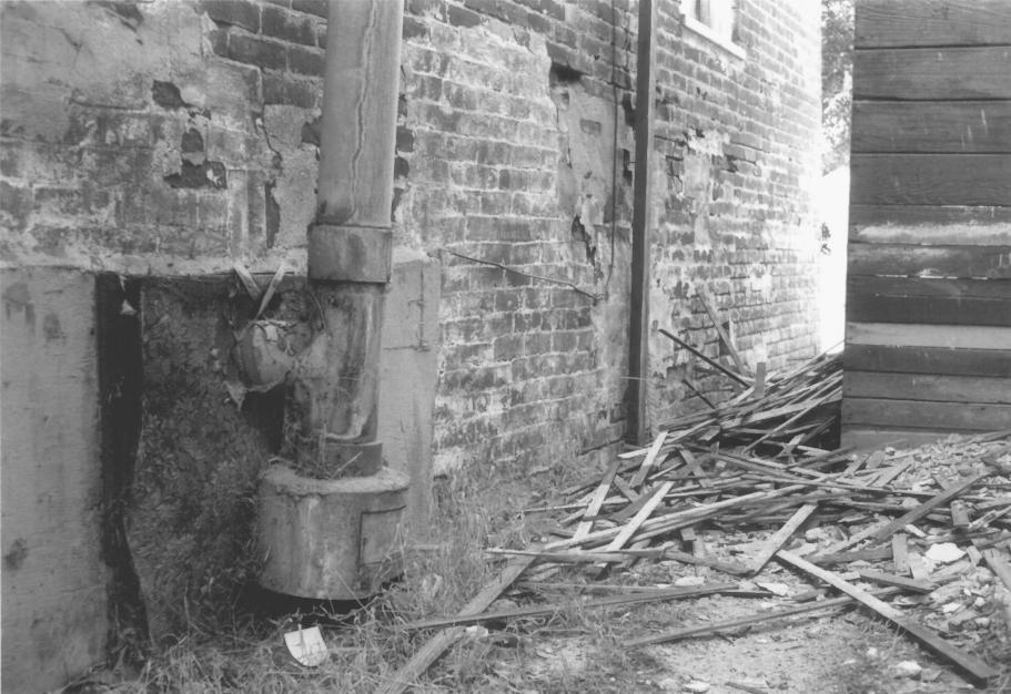
DOE The Carr House Benicia, Ca. SEP 3 #9412 Solano County, California Hill's Library Facing east and showing old concrete botch of a patch and sad condition of brick. Cistern is by left corner and believed to be egg-shaped. When frame addition is jacked, cellar will be dug to expose the cister.
