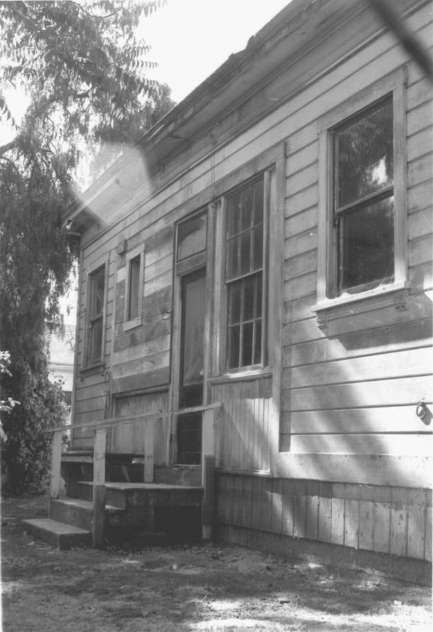
SEP 3 979 #8412 The Carr House Benicia, Ca. Solano County, California Photo by Nancy Olson, July 78 JUL 3 0 1979 Hill's Library Back door facing south. Note how rear center section has been filled in and enclosed using the older window which probably came from the original back wall. Wincow brackets are in keeping with 1900 frame addition.
