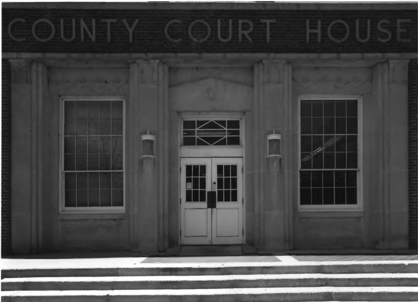
QUITMAN COUNTY COURTHOUSE AND OLD JAIL QUITMAN COUNTY, GEORGIA 2 OF 7
