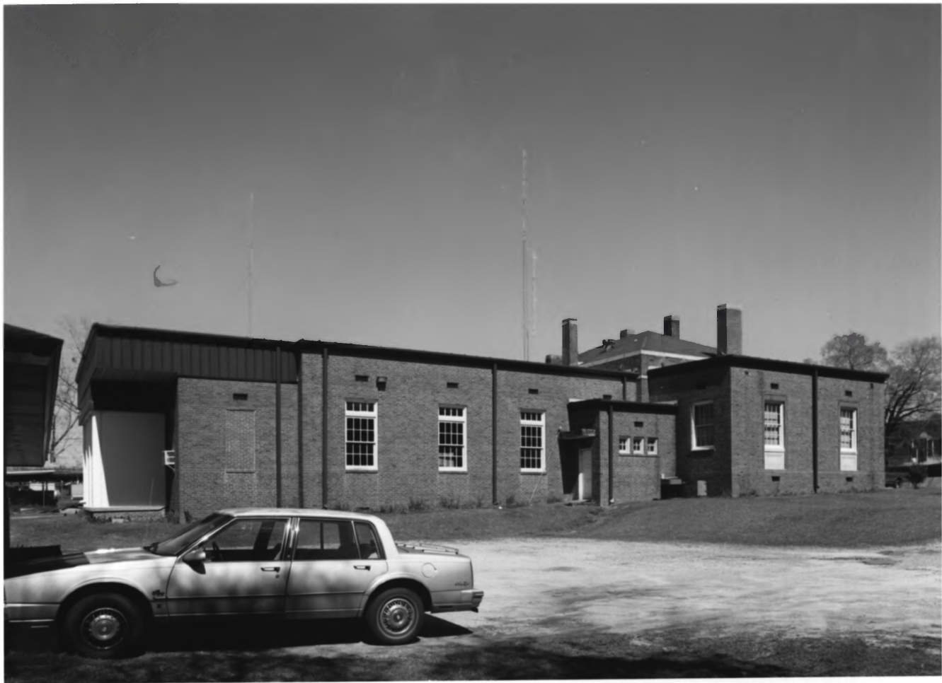
QUITMAN COUNTY COURTHOUSE AND OLD JAIL QUITMAN COUNTY, GEORGIA 3 OF 7
