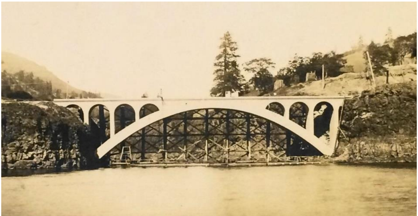
Figure 17. SP&S Klickitat River Bridge, reinforced-concrete arch. Source: MHS.
