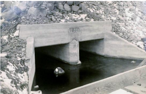
Figure 41. SP&S two-chamber concrete culvert.
