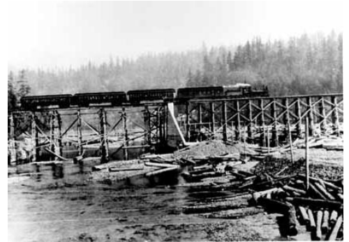
Figure 21. SP&S framed trestle at Wind River.
