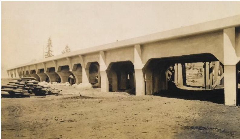
Figure 18. SP&S reinforced-concrete viaduct. Source: MHS.
