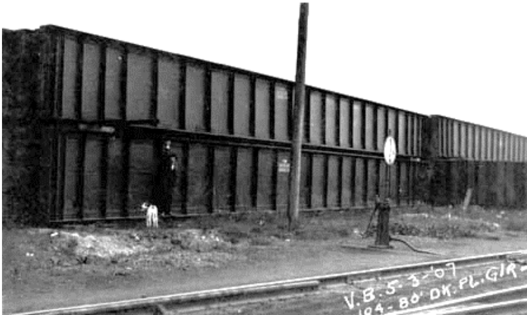
Figure 13. SP&S deck plate girder bridges stacked for future installation, 1907.
