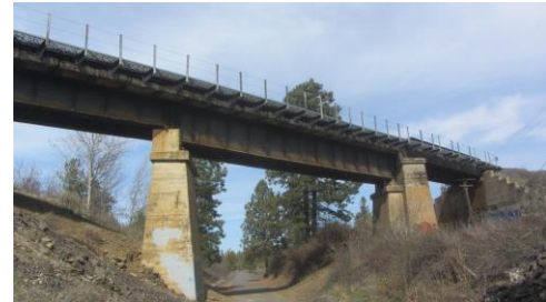
Figure 24. SP&S “deck-plate” girder span, Fish Lake Bridge.
