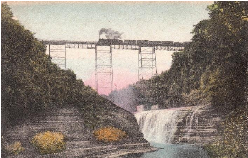
Figure 16. Portage Viaduct after replacement of original iron trusses with steel deck plate girders and trusses.
