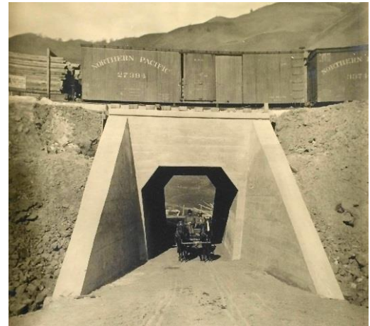
Figure 19. SP&S reinforced-concrete culvert. Source: MHS.
