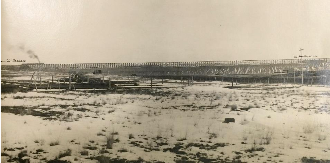
Figure 9. Sprague Gulch trestle, ca. 1908. Source: MHS.
