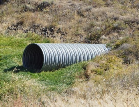
Figure 42. SP&S metal pipe culvert.
