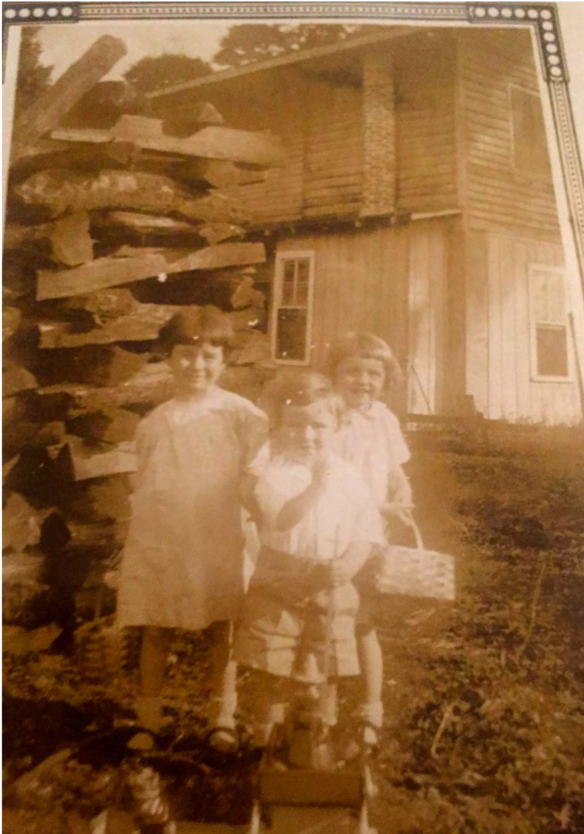
Figure 2. Kleinpeter children standing by the rear elevation of the Kleinpeter House - Willow Grove c. 1929. Image courtesy of the author. This view shows the loggia already enclosed and the small kitchen addition in place.
