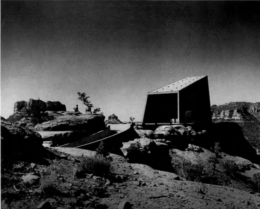
Figure 4. View looking SE showing the main entrance, a portion of the serpentine ramp, the skylights and the setting of the Chapel of the Holy Cross immediately after completion. Anshen & Allen, Fall, 1956.
