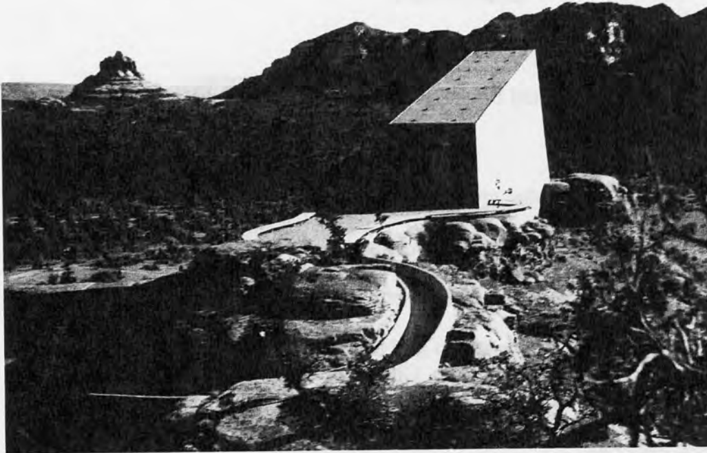
Photograph looking south, showing the serpentine ramp, the main entrance and patio area at the top of the ramp, Chapel of the Holy Cross, by George Jordan, 1960.
