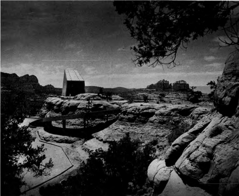
Figure 6. View looking west showing the main entrance, a portion of the serpentine ramp, the skylights and the setting of the Chapel of the Holy Cross, immediately after completion. Anshen & Allen, Fall, 1956.
