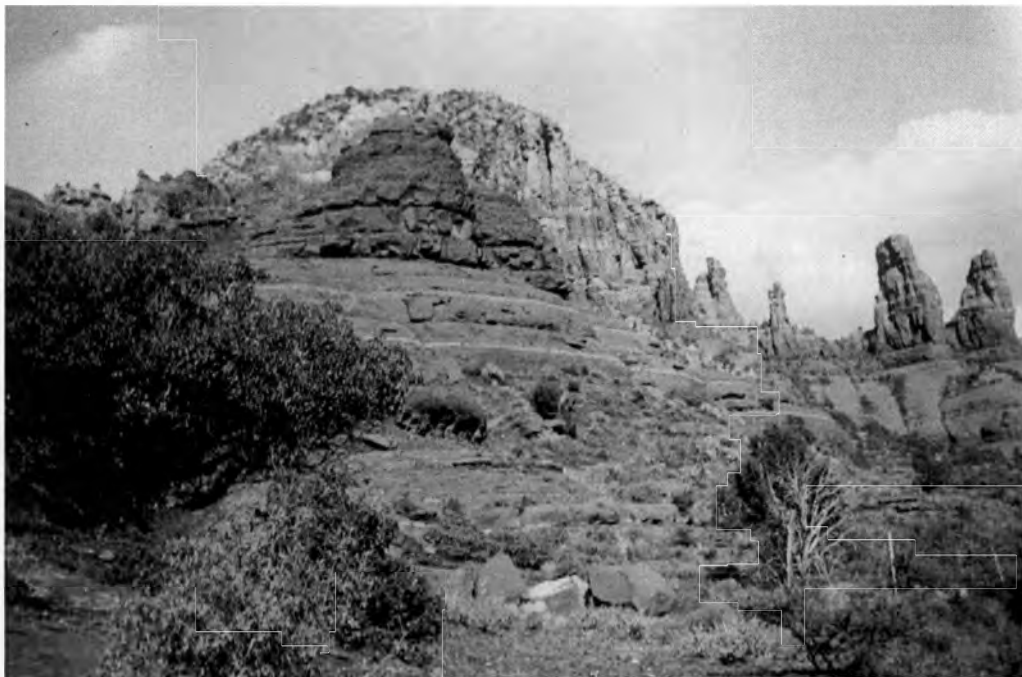
Figure 2. View looking NE showing the site of the Chapel of the Holy Cross prior to beginning construction; shows the twin buttes that form the base of the chapel. Anshen & Allen, Spring, 1955.
