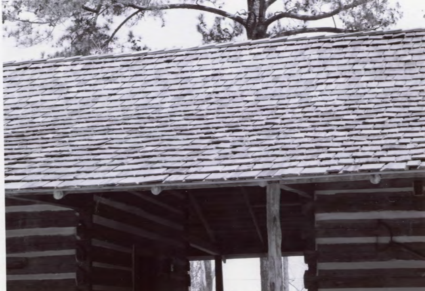
MS- Forrest County — Meador — 0003.tif Exterior Roof cedar shank shingles
