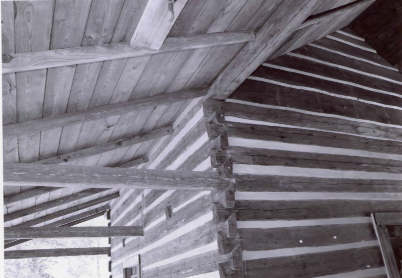
MS_ Forrest County - Meador_0004.tif Exterior East Front Porch, Roof, Walls Beams, rafters, chinking, dovetail corners, logs
