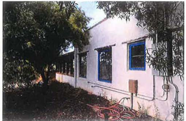
Photograph #8 View of west façade showing glazed sleeping porch.
