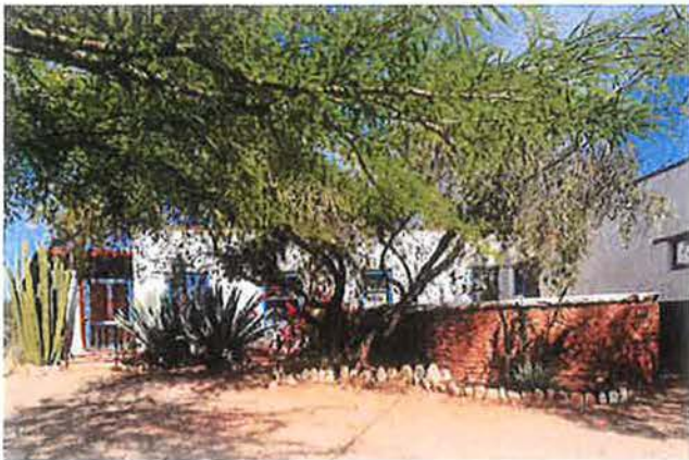
Photograph #3 View of southeast facade showing side porch entry and service yard wall.
