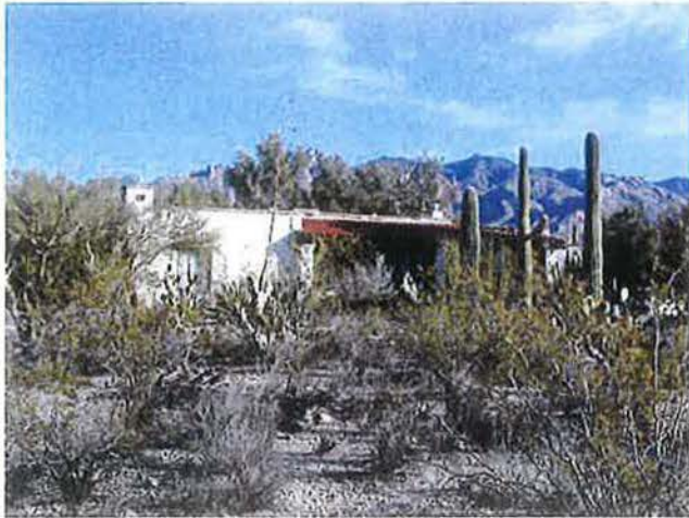
Photograph #1 View of site looking north towards house.
