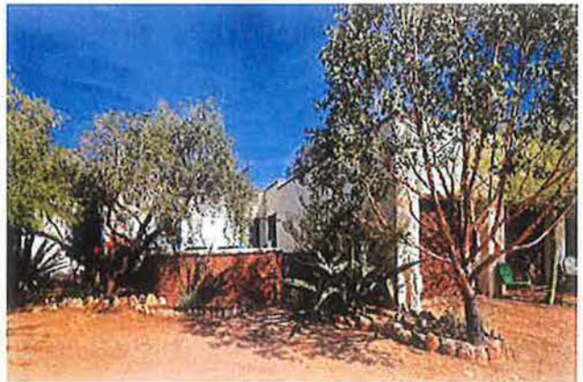
Photograph #4 View of part of southeast facade showing service yard wall and garage.
