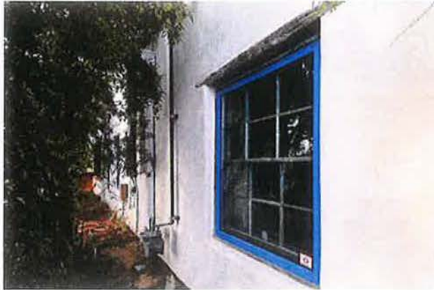
Photograph #9 View of west façade showing double hung windows with storm window.
