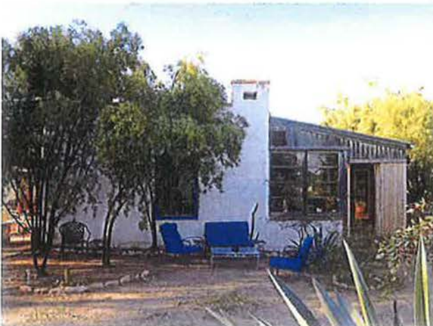
Photograph #7 View of north façade showing glazed sleeping porch.
