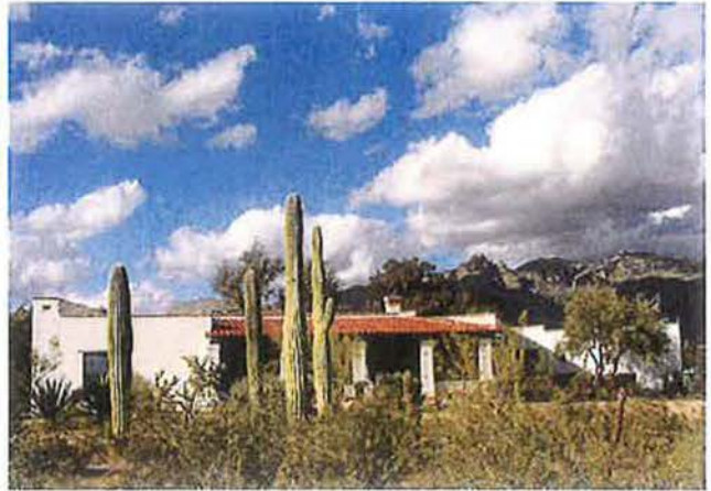
Photograph #2 View of south (primary) facade showing covered porch.
