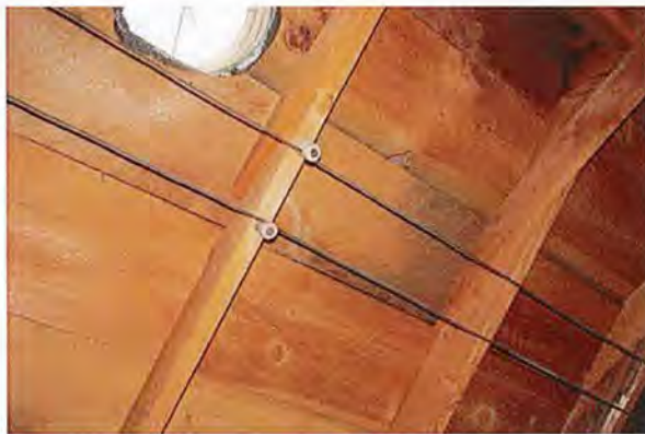
Knob and tube wiring visible in the attic space of the house at 207 S. Arizona Ave., Prescott, 2018. Source: Cat Moody, City of Prescott Historic Preservation Officer.
