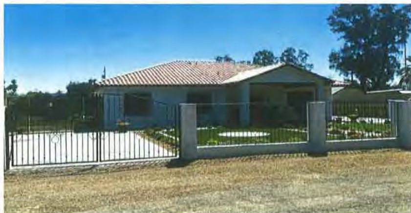
Figure 2. House at 336 S. Calle de Madrid, Tucson, 2018.
